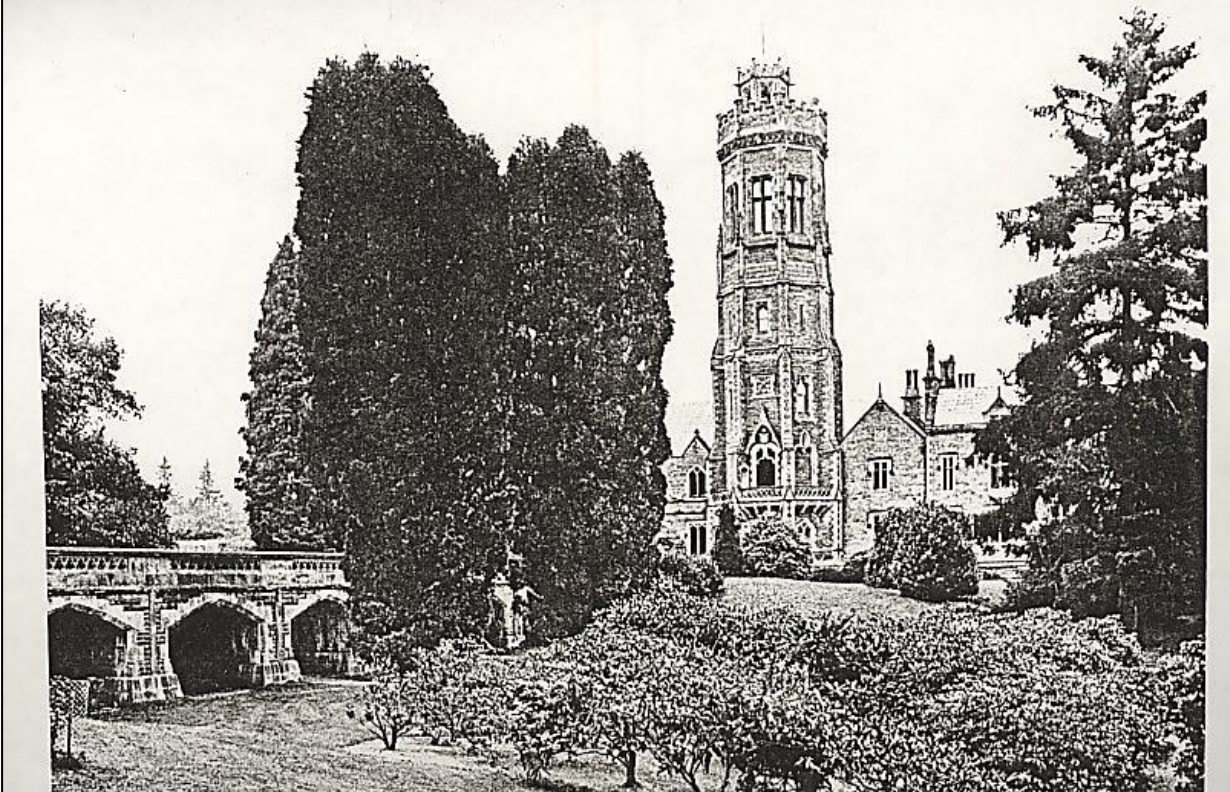
Bridge on the South East
