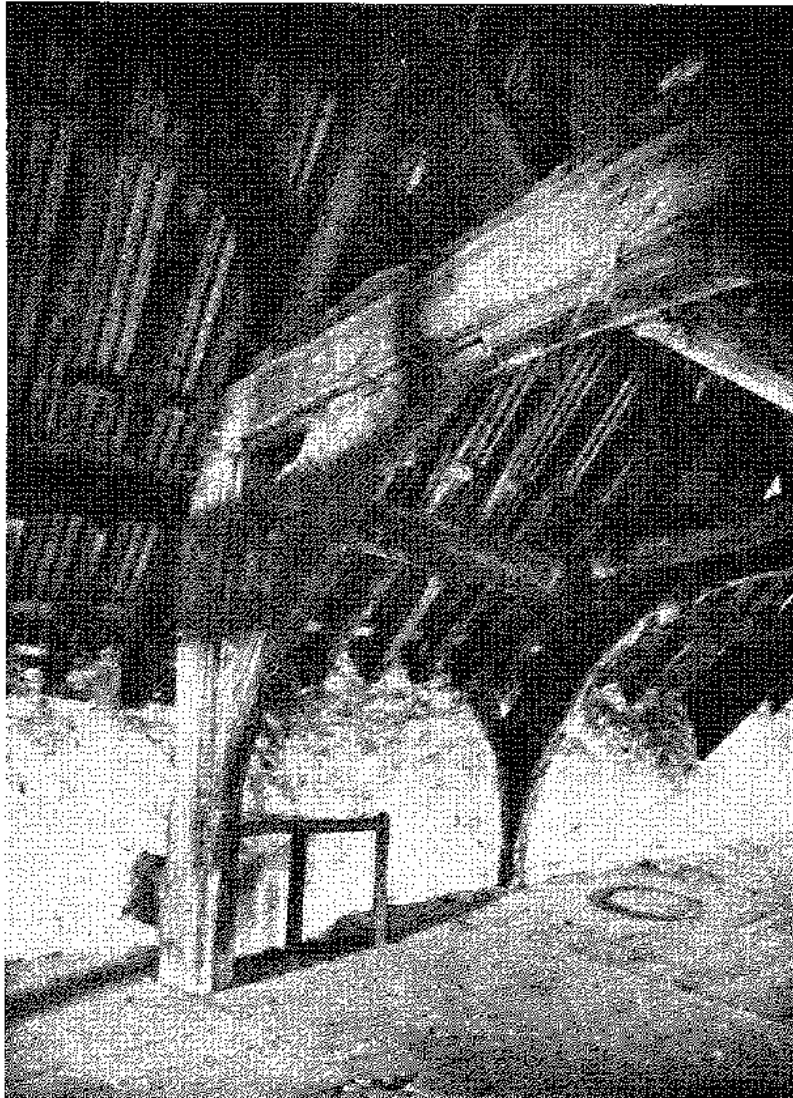
Fig. 5. Plas Uchaf. The Main Roof Truss.
