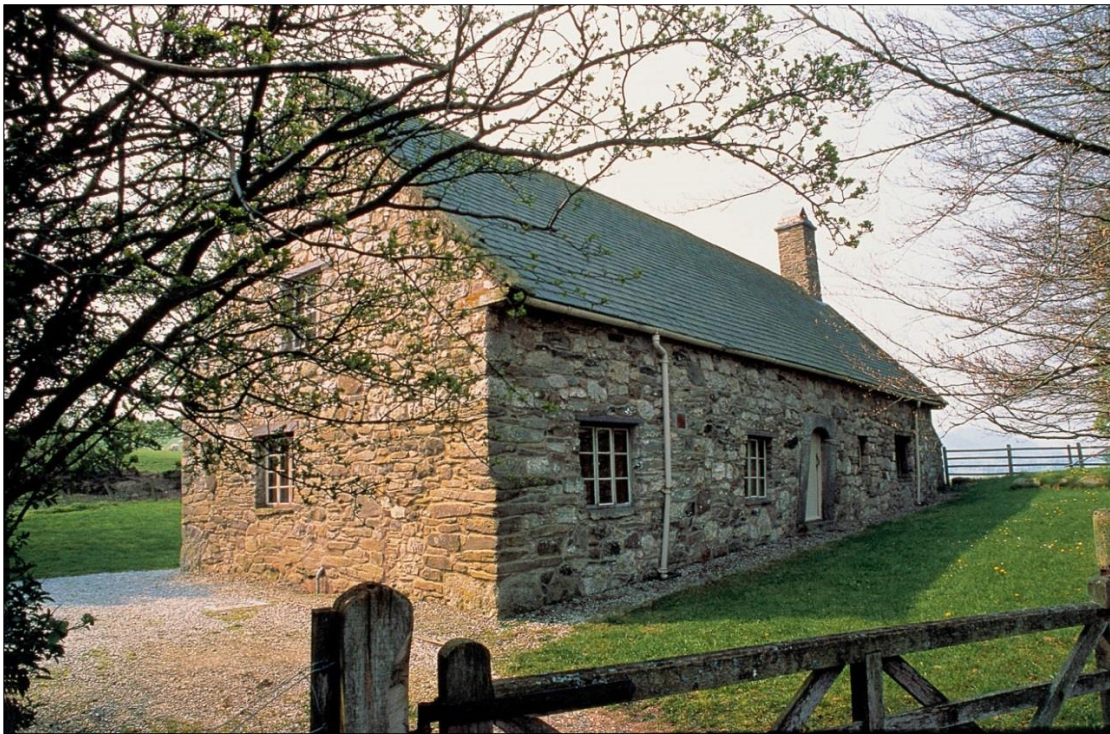
The completed north front.
