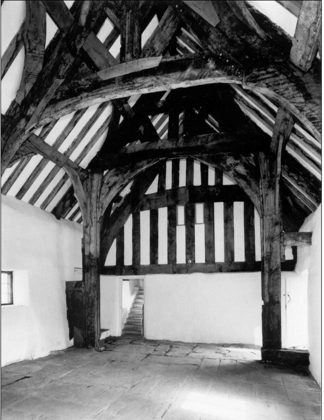
Interior after restoration.
