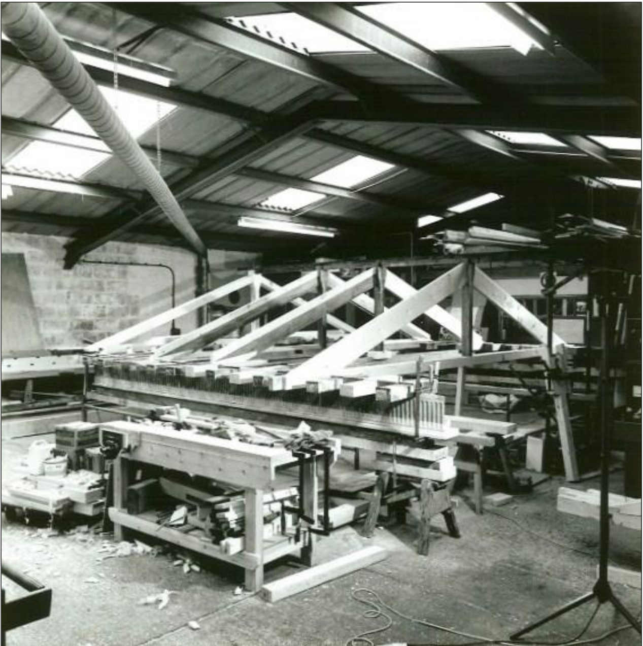
Meanwhile the roof was gradually reassembled in Houghton's joinery workshop.
