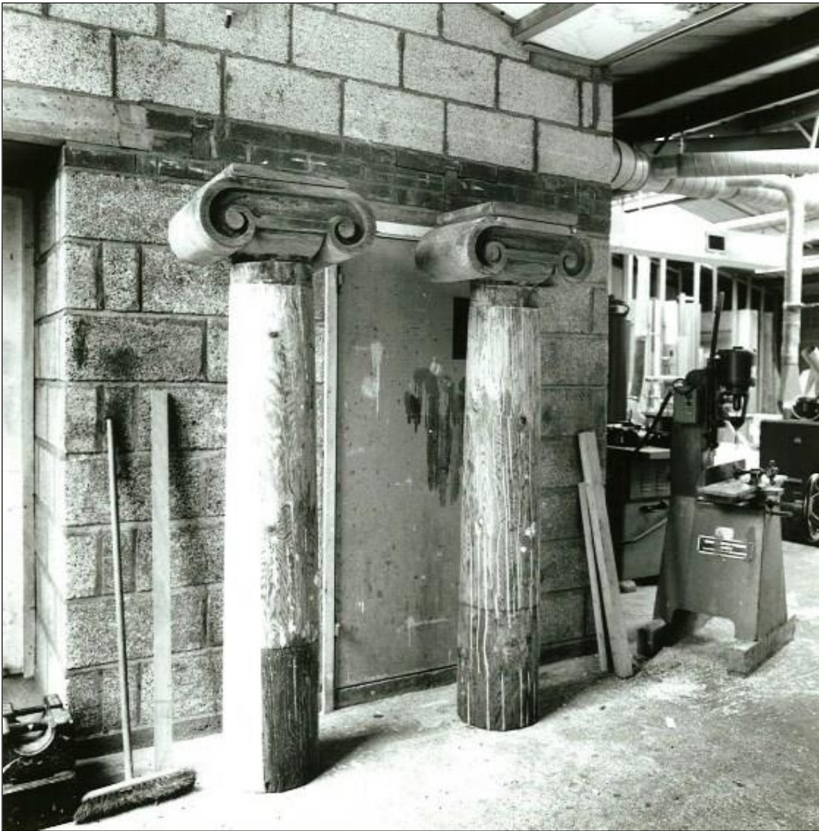
The two columns that could be saved. The paler strips are where new wood has been filleted in.
