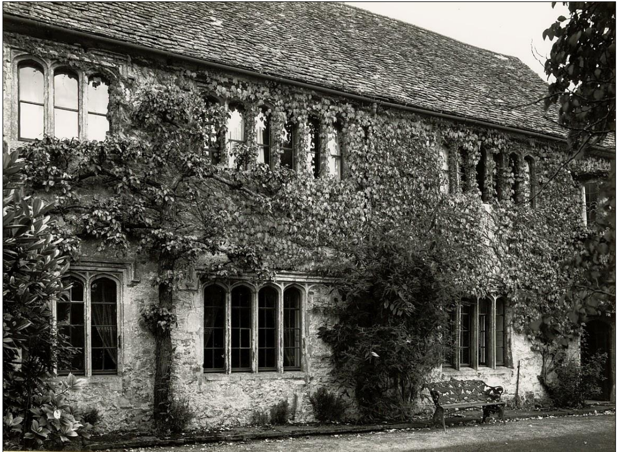
The west front in 1937. The blocked window lights of the central window can clearly be seen.
