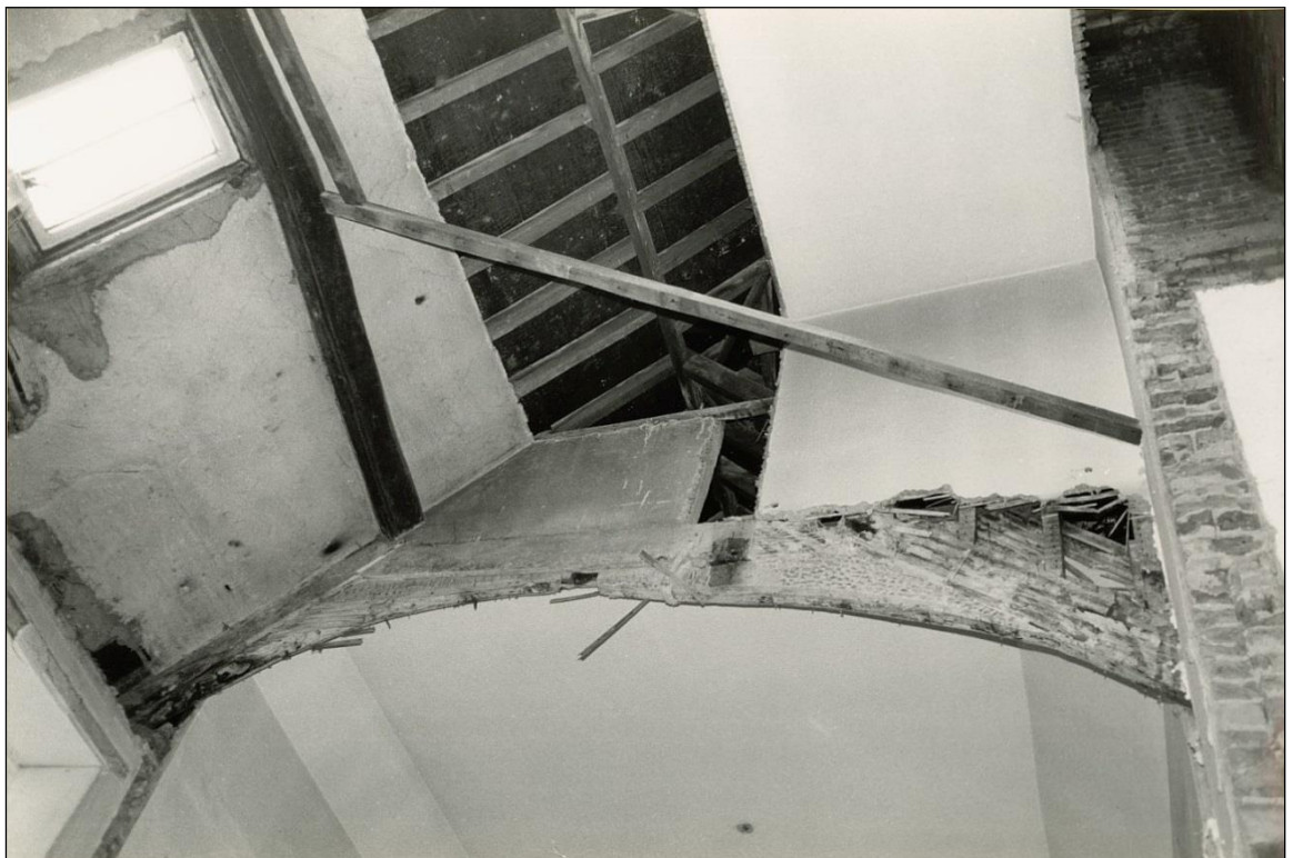
An altered collar beam in the east wing. High up on the left is a Tudor tie beam which has been re-issued as a purlin.
