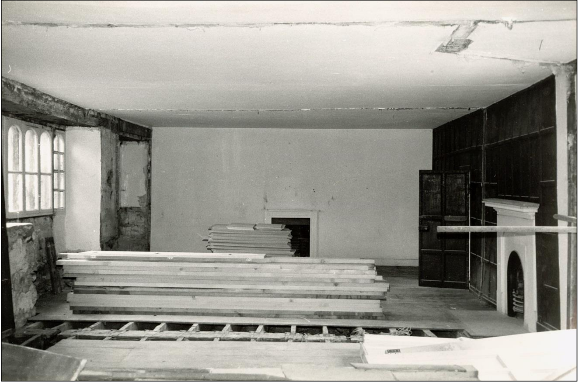
The end frame of the east wing added c. 1425. On the right an earlier brace of the main block's original timber frame can be seen
