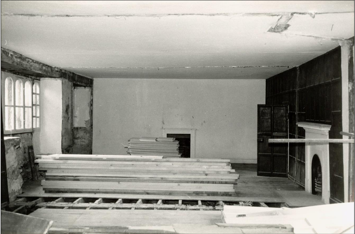
The first floor after the 1819 partitions were taken down. New floor boards had to be laid.
