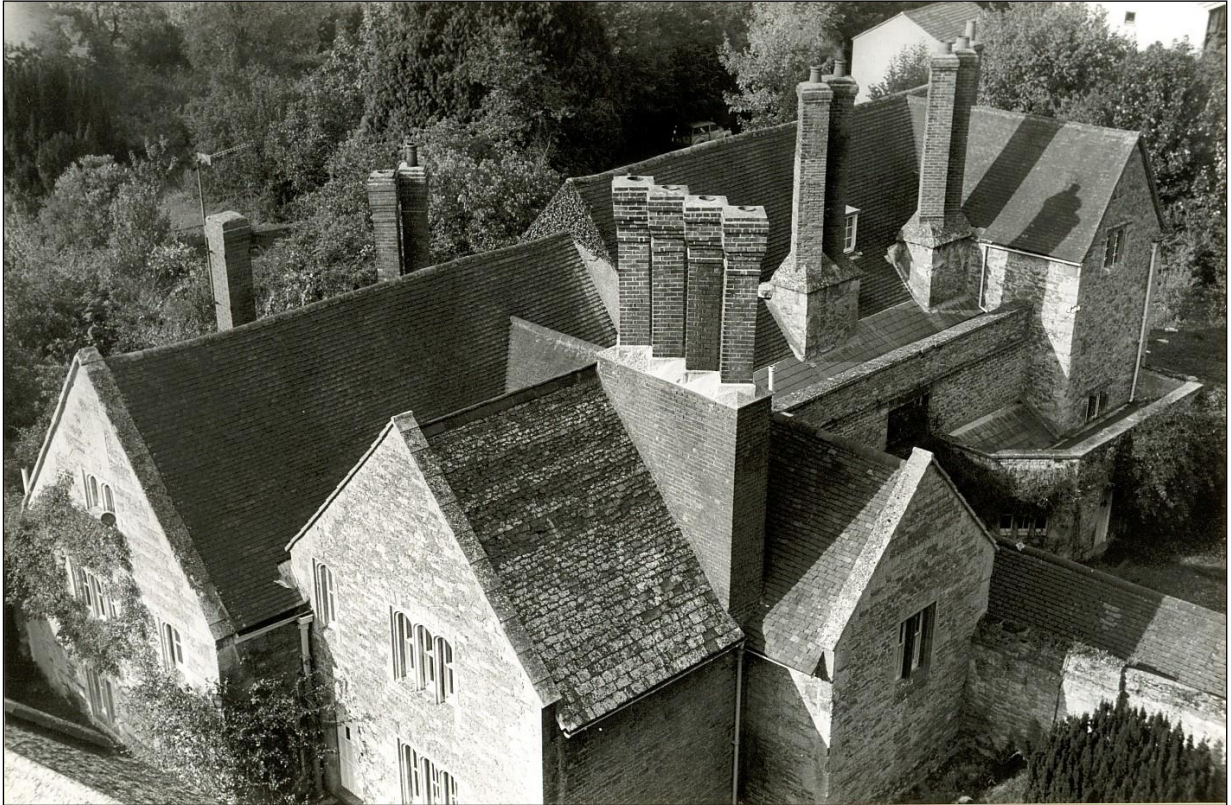
From the top of the Church tower, showing the 1819 corridors and the 1839 porch.
