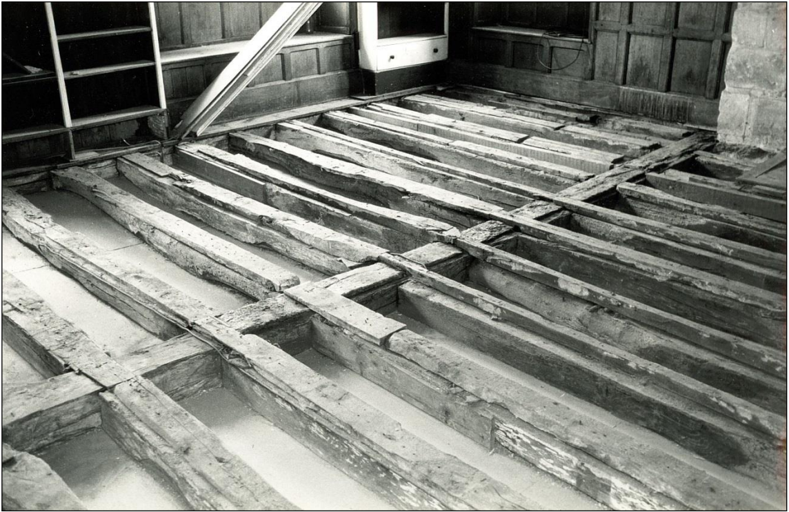
The medieval floor joists in the study, on the first floor of the South Block
