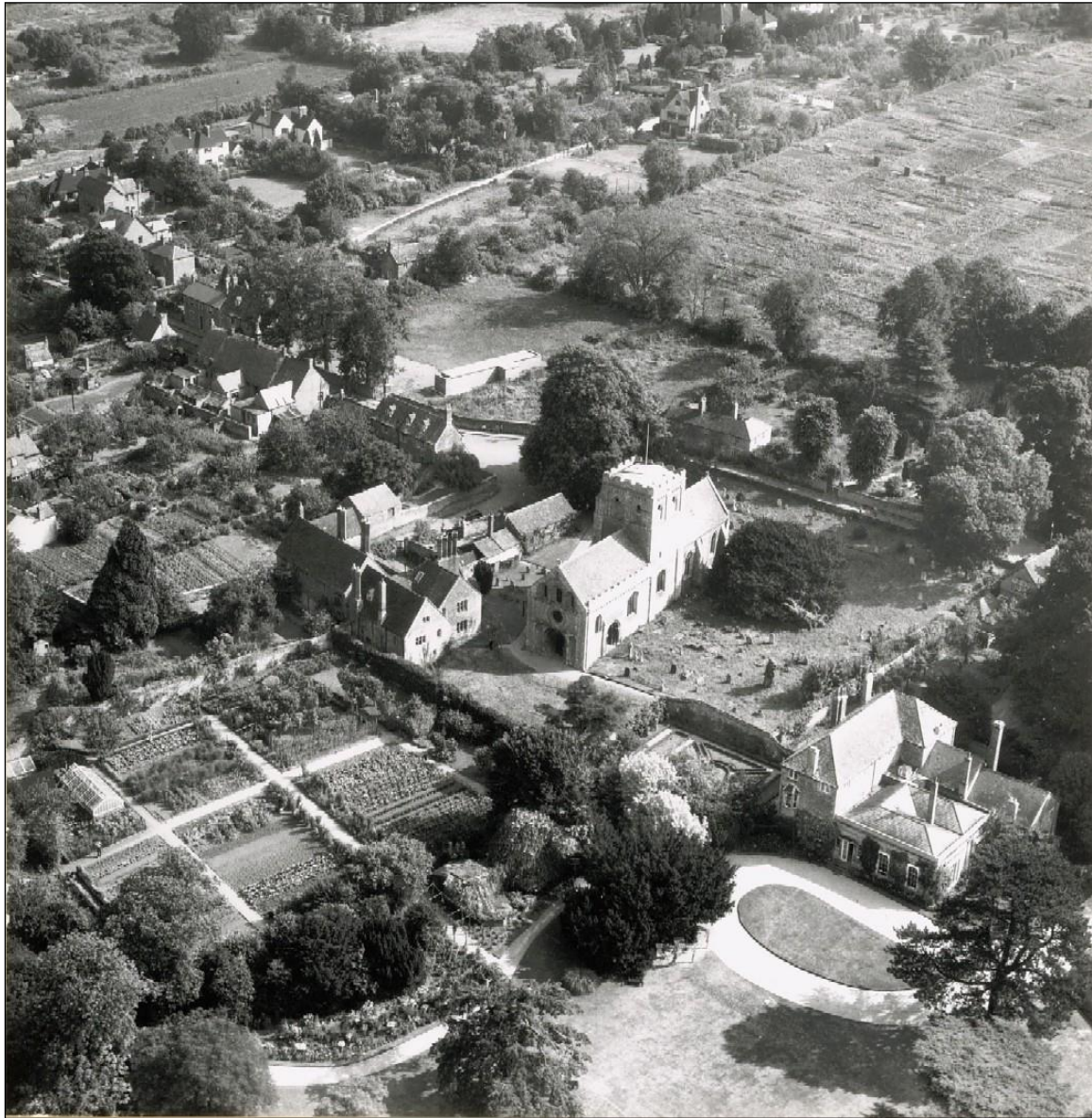
An Aerofilms view of Iffley in the 1950s, when little change had occurred for a century or more. At this time, the garden wall of Court Place, the large house in the foreground, still ran very close to the South block of the Rectory.
