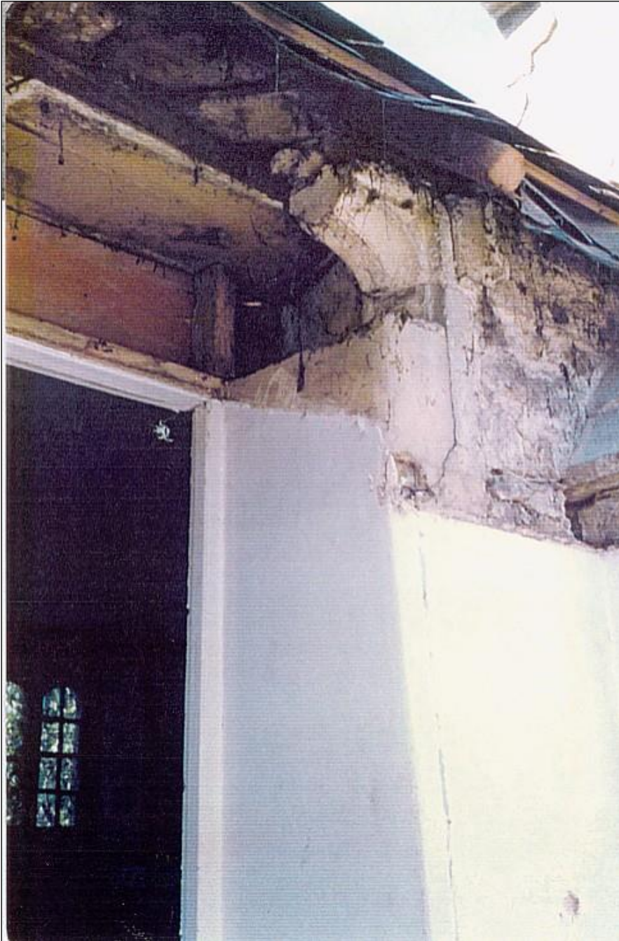
Remains of a Tudor window, found between the chimneys
