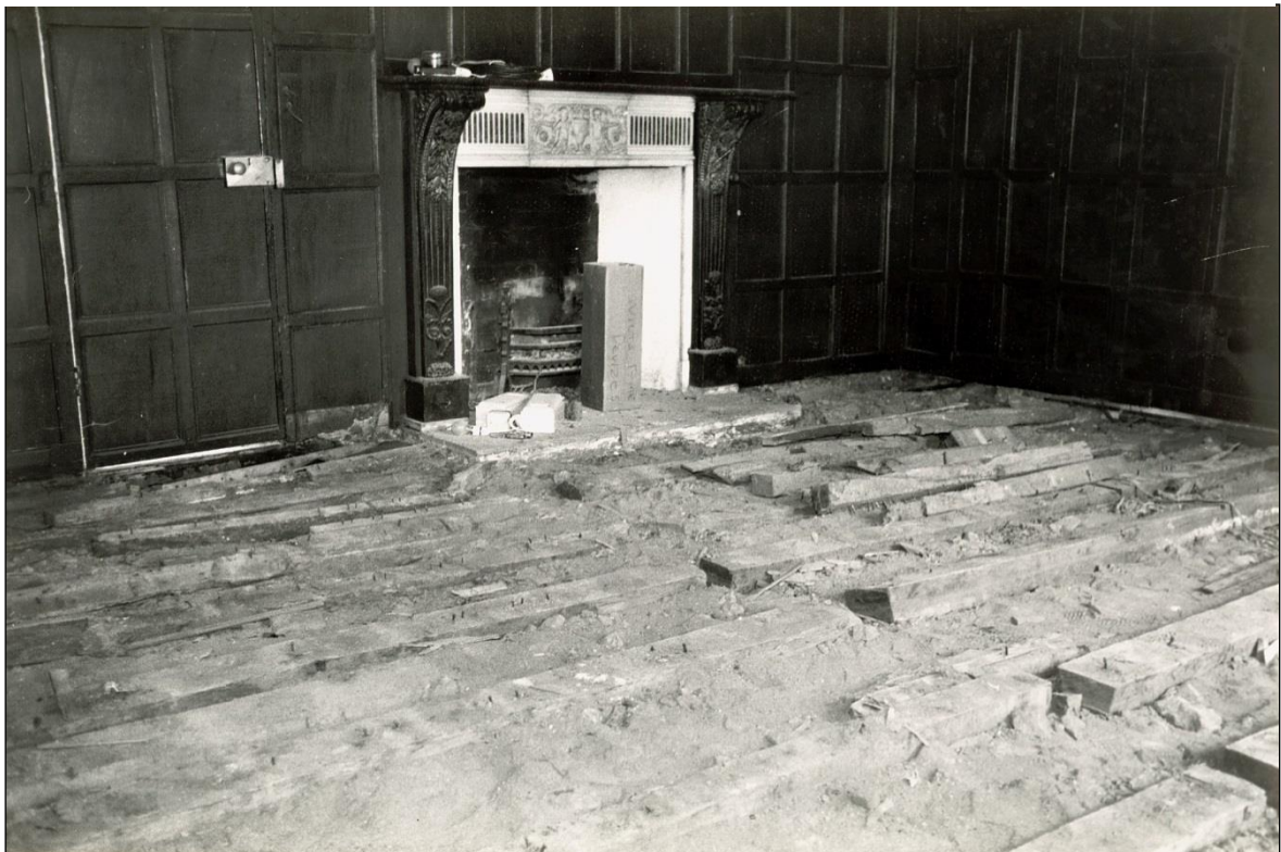
The Tudor joists, lying directly on the ground in the drawing room
