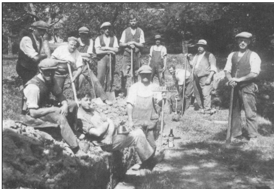
Pyments' men building Griggs' house in Campden, Dover's Court, in the late 1920s. The same team may well have worked on the repairs to the Almonry.
