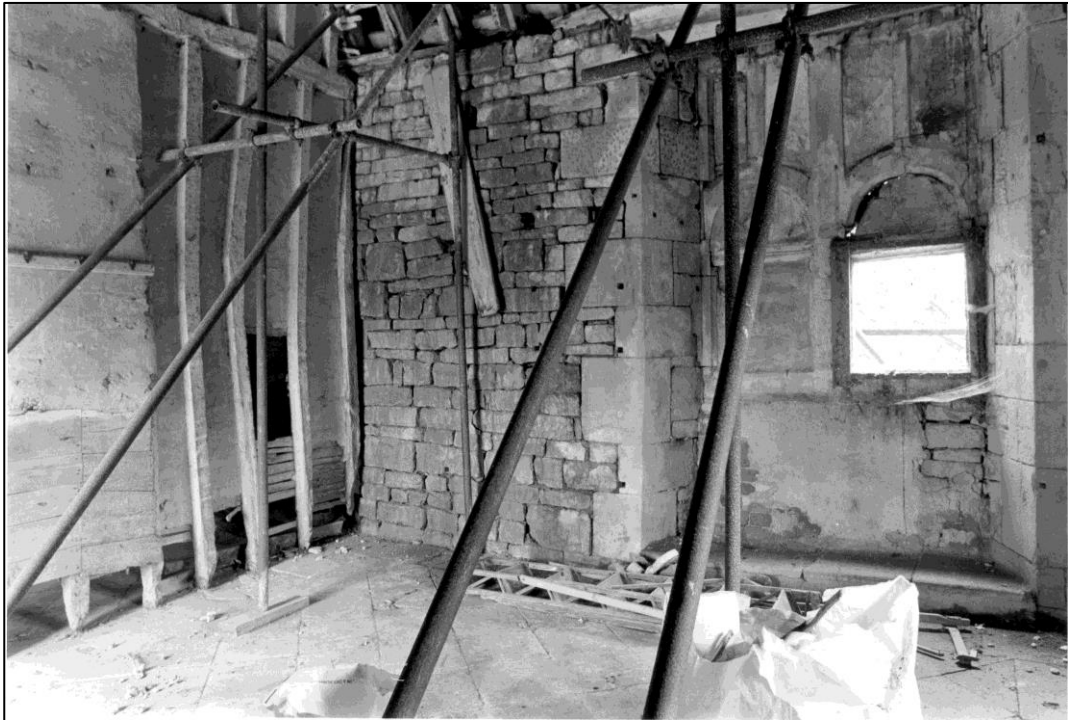
The first floor before restoration.
