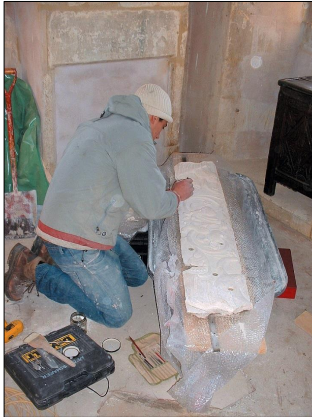
Piecing together fragments of the decorative frieze below the cornice on the first floor.
