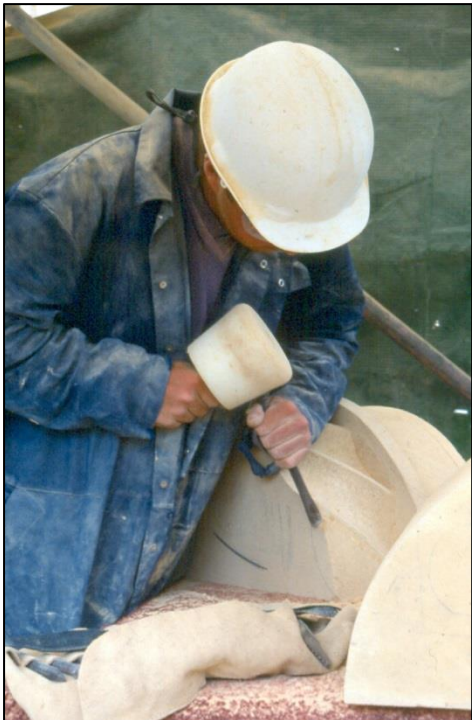
Chiselling the 'barley sugar' fluting on the new chimneys.
