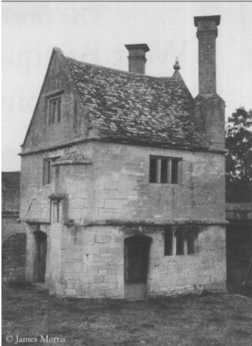
The Almonry before restoration.
