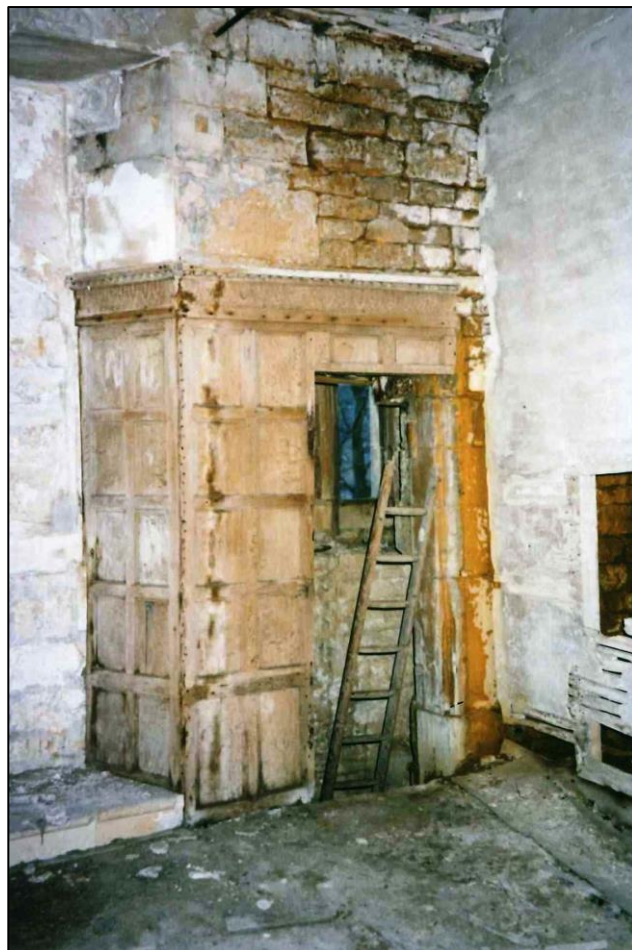
Panelling surviving on the upper floor.
