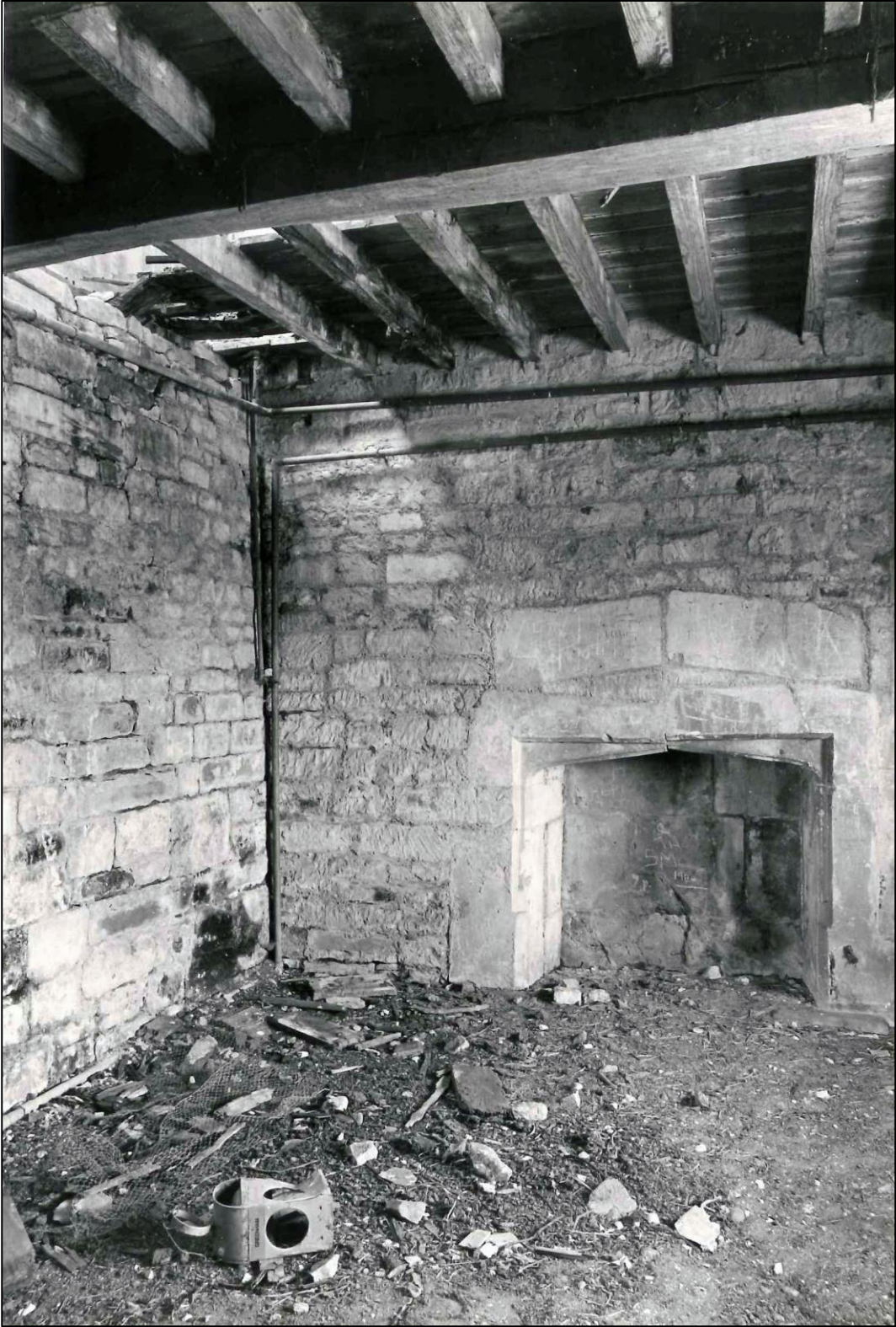
The staircase up to the top floor is now in this corner.
