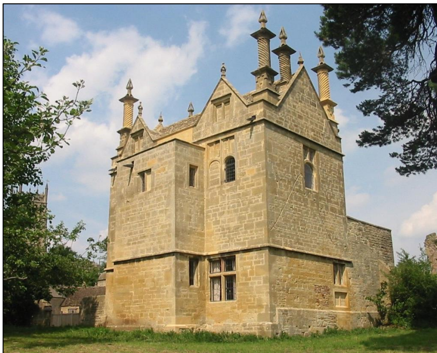
The view of the south-west elevation after restoration showing the unblocked west window and the re-blocked lower half of the window on the south.
