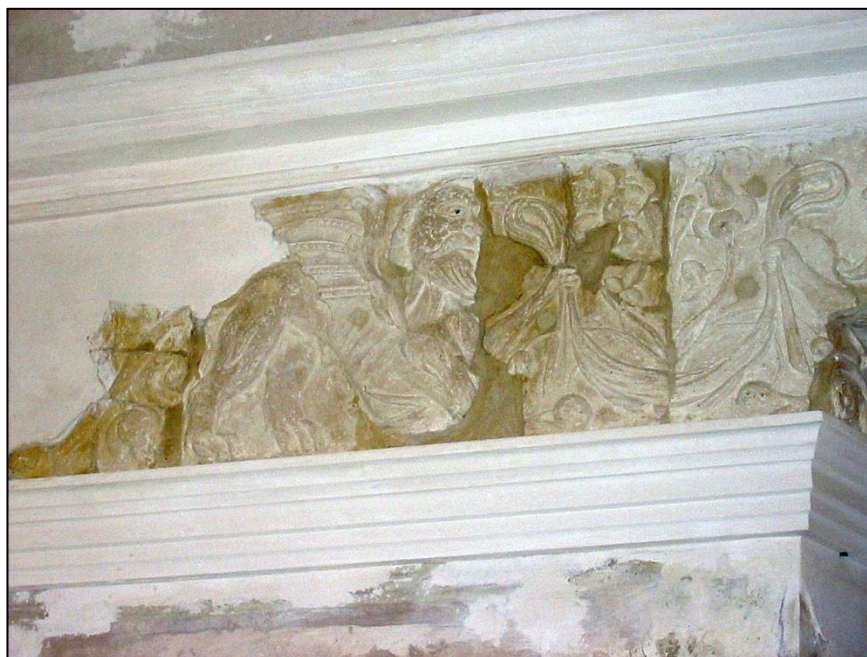
The blackened eye of the winged grotesque was the only evidence of colour that remained and which we have reinstated.
