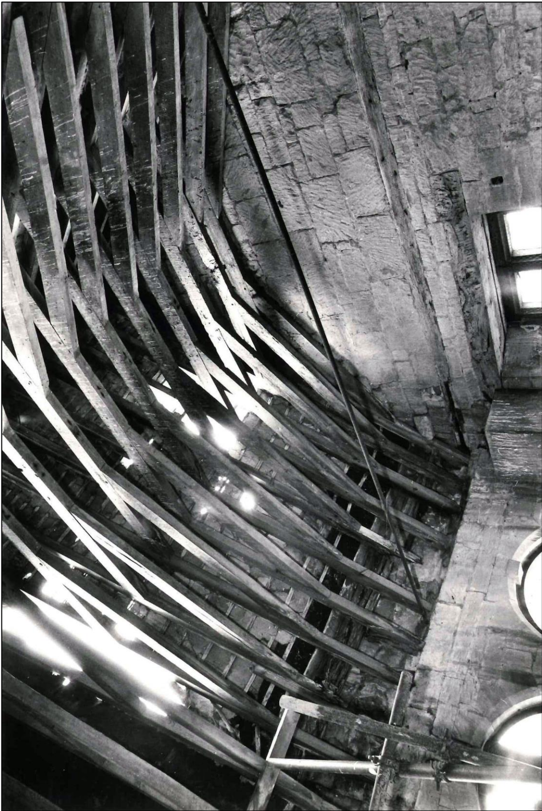
The roof had to be completely dismantled.
