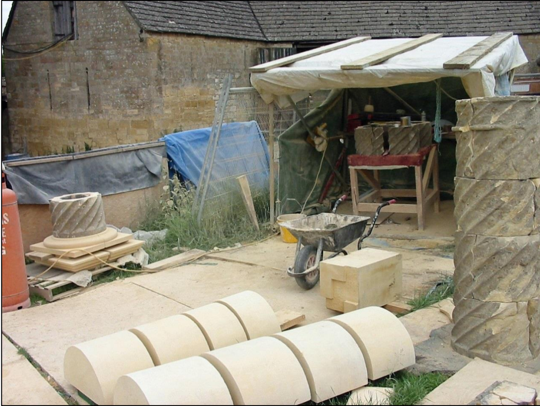
Two new chimneys were built on site in a traditional stonemason's bankers' shed, June 2002.
