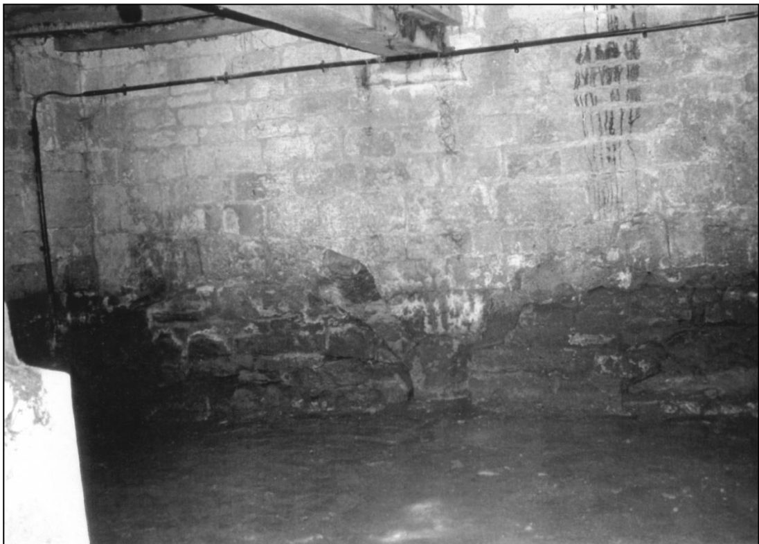
The cellar of the Almonry, showing the possible conduit arches built into the wall (now blocked) and drainage channel down the centre.
