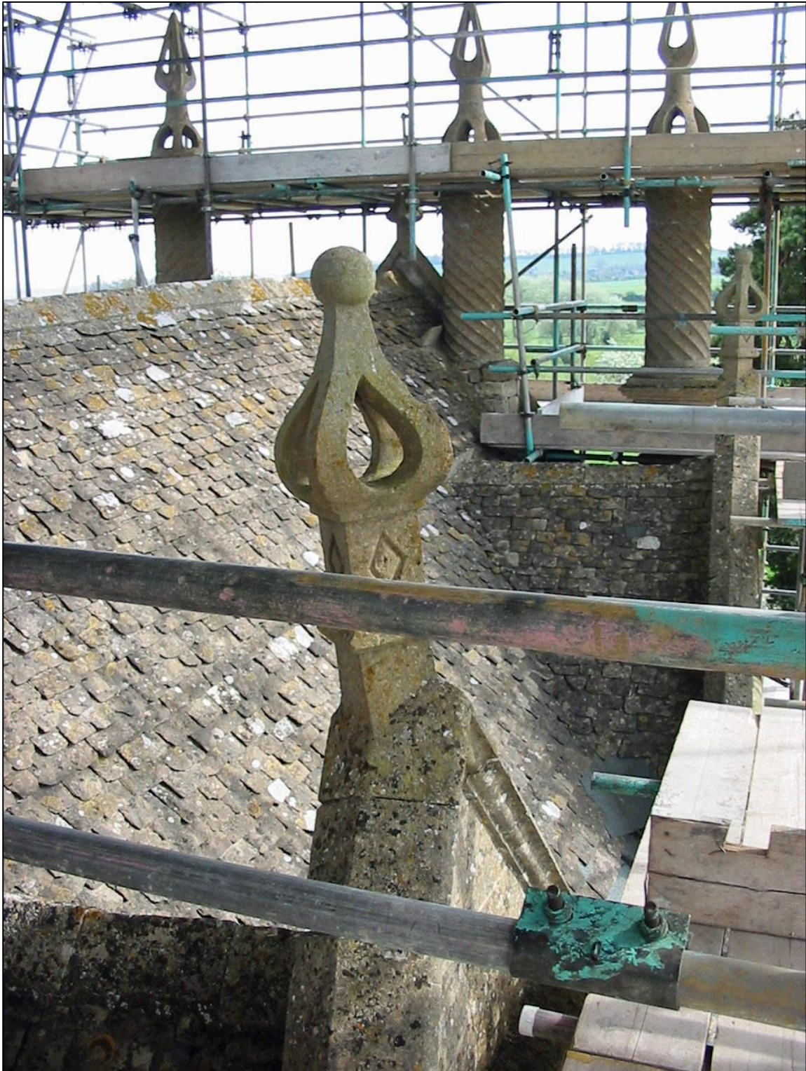
The roof undergoing repair.
