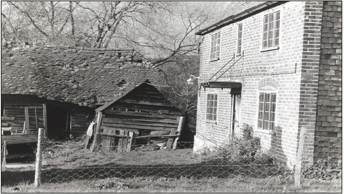
The cow-byre with attached shed prior to renovation, 1991.
