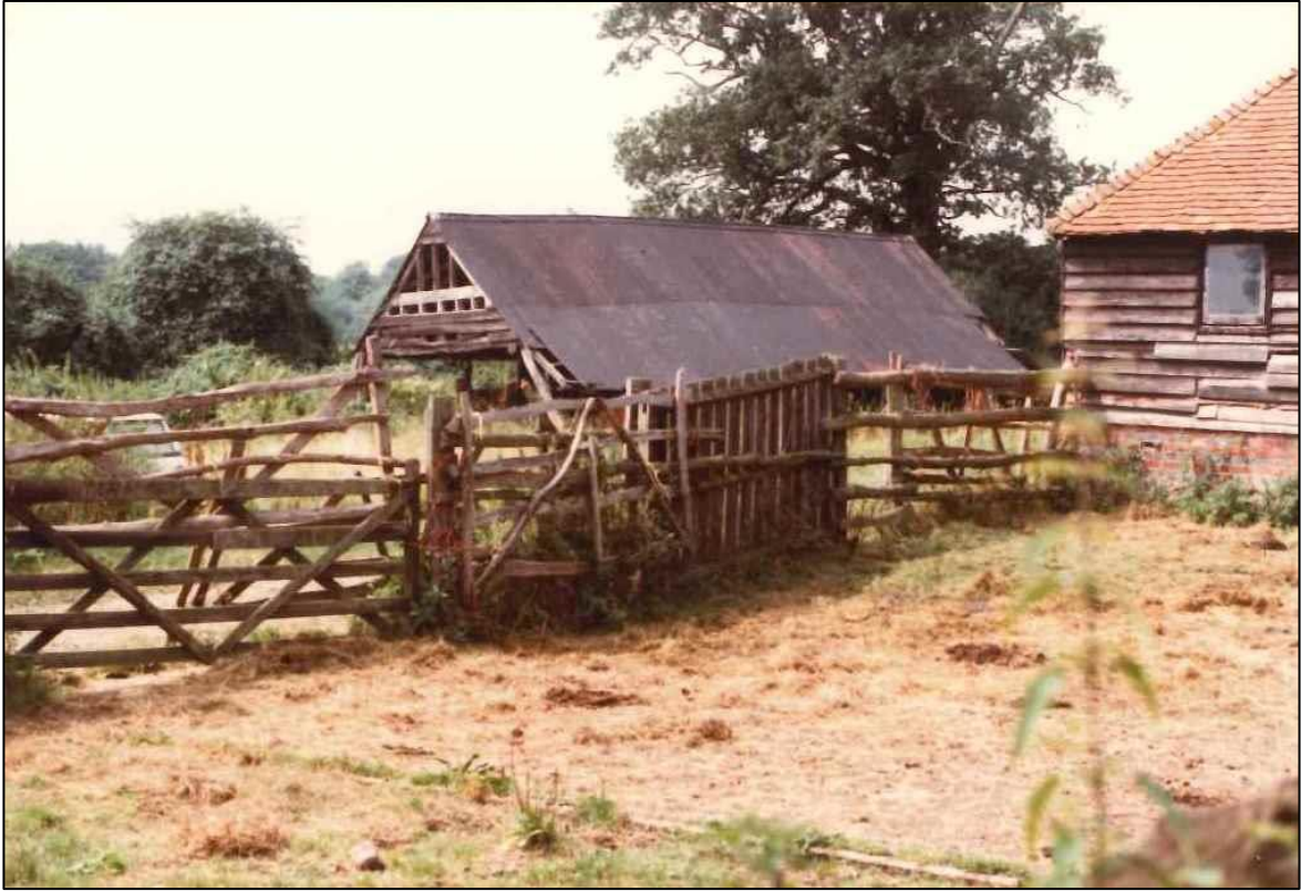
The demolished cartshed.
