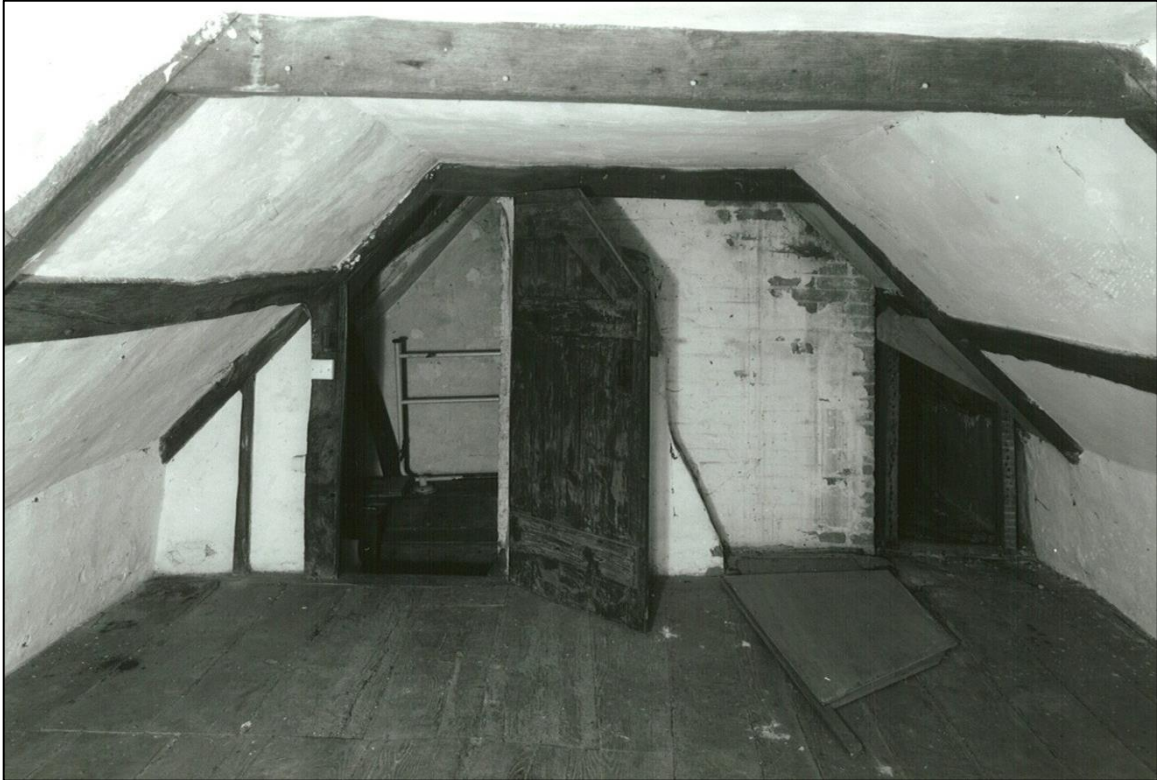
The attic room.
