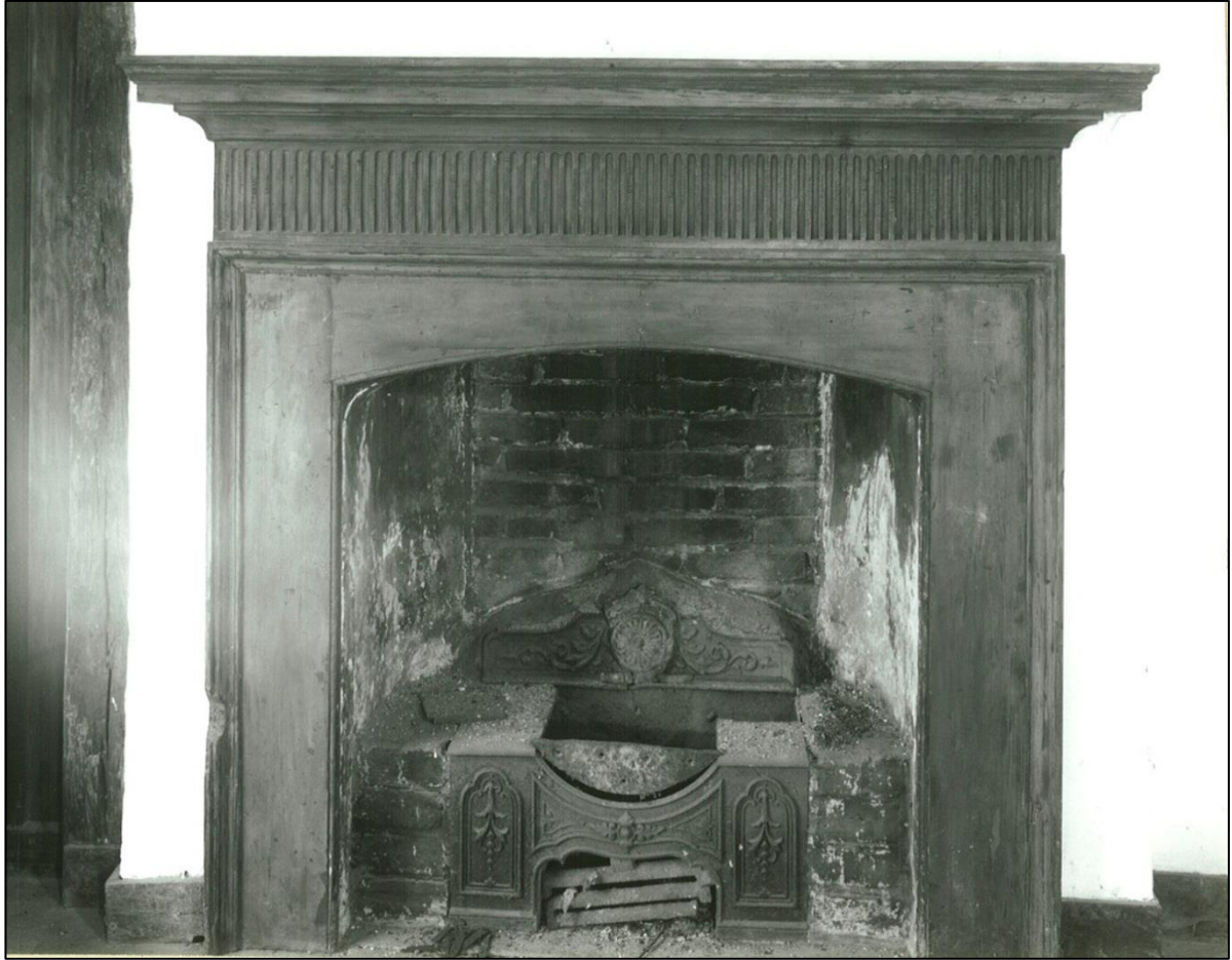
The fireplace in the south-east bedroom.
