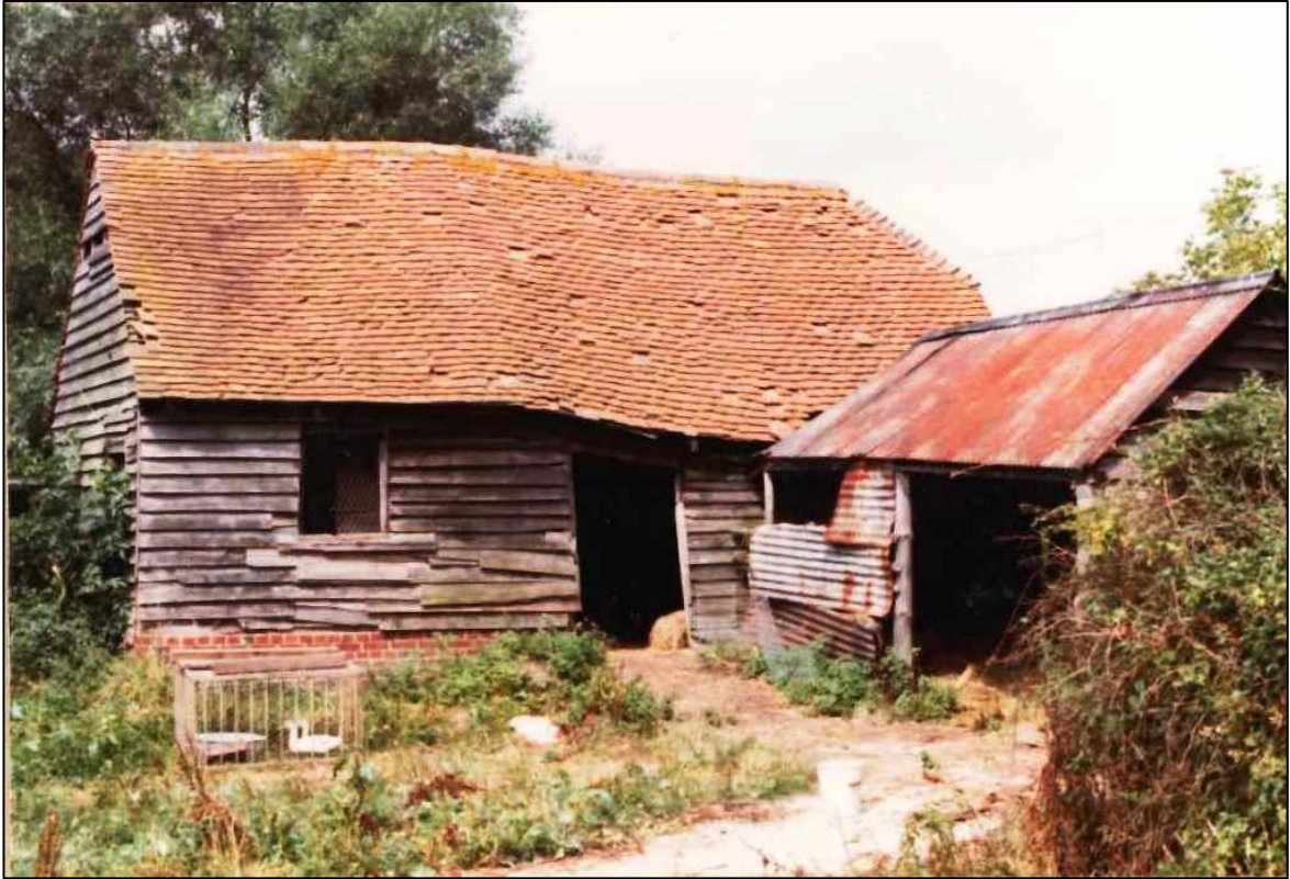
The cow byre with attached shed.
