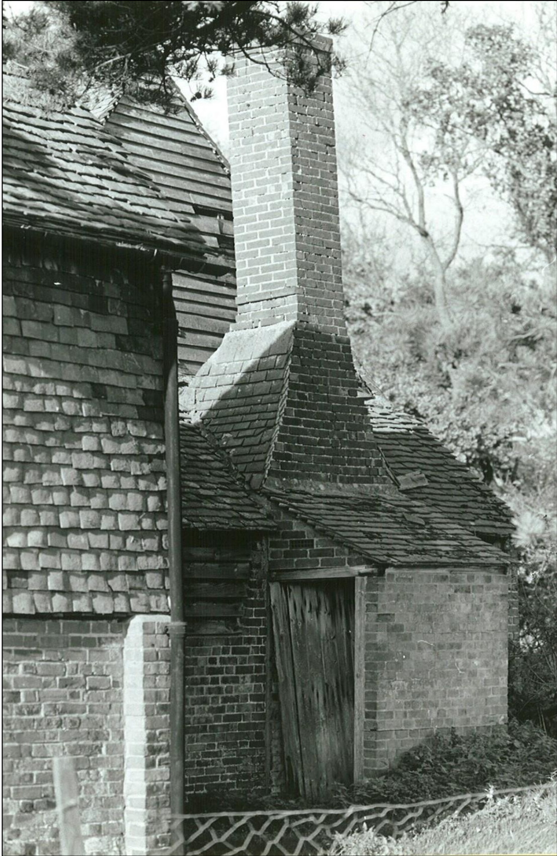
The chimney of the bakehouse (now reduced) and the demolished privy.
