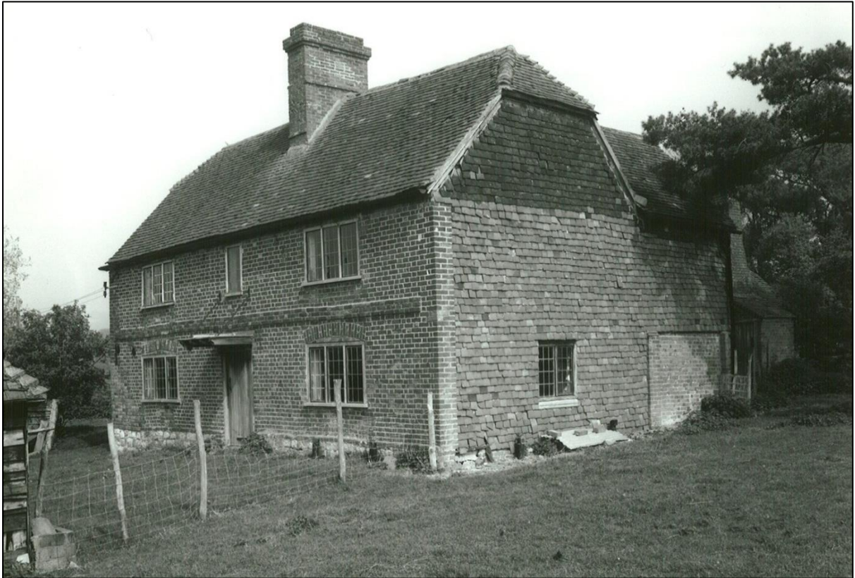
The east elevation before the first floor window was reinstated.
