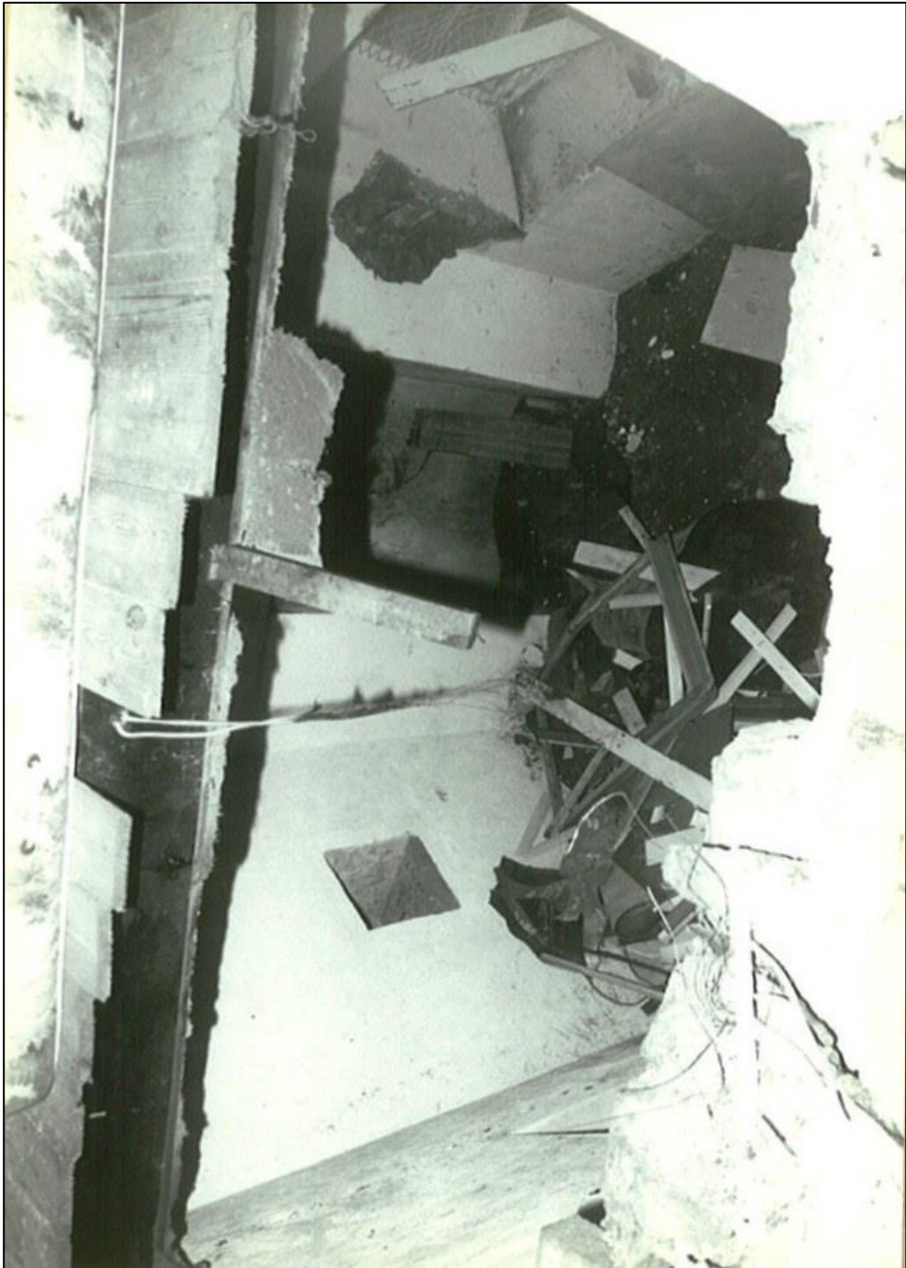
Looking through the hole in the first floor towards the ground floor
