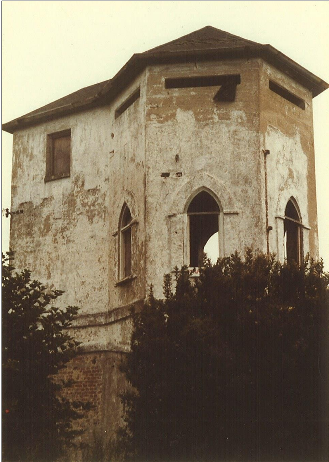
Nicolle Tower – the roof of imitation slates was removed
