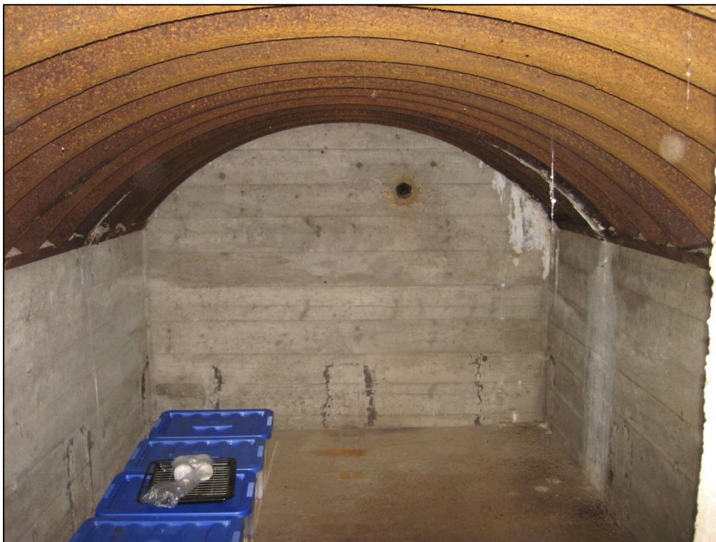
Bunker 4 is a larger Wellbech type shelter and originally had steps going down into it from the front door of the Tower, the steps remain but the entrance is now blocked. This was for troops to quickly access, in case the Tower was attacked.
