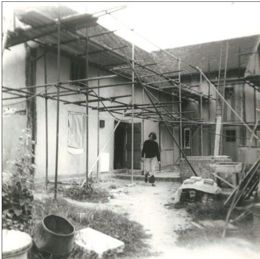
Restoration of the rear nearing completion.
