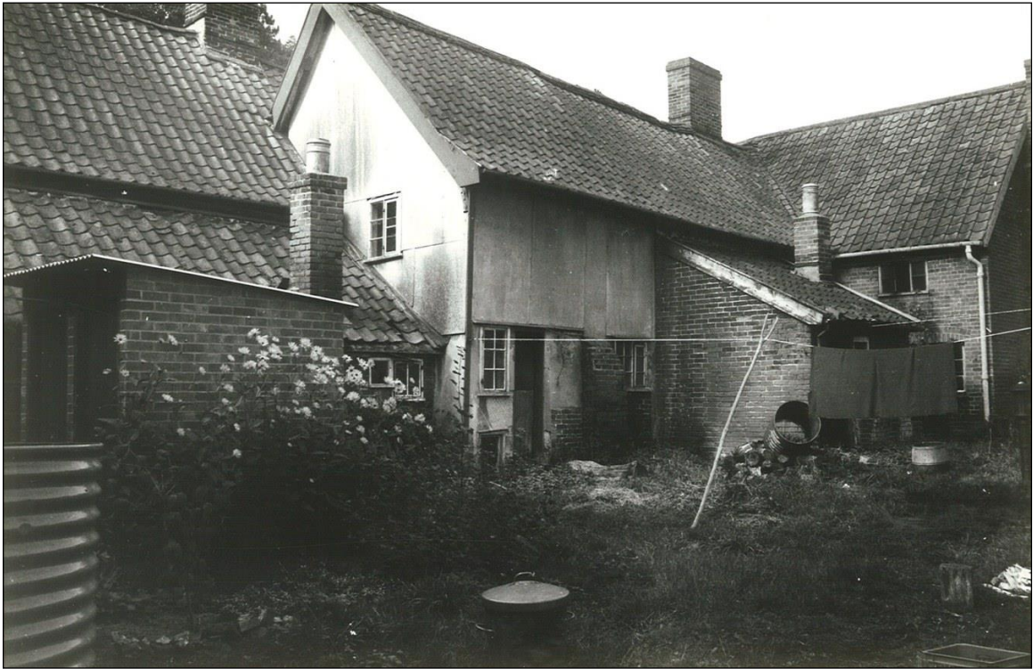
The back of the New Inn before it was restored. The brick lean-to was removed.
