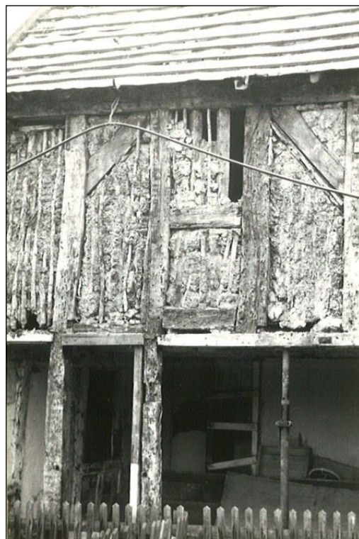
The same wall showing the complete window.
