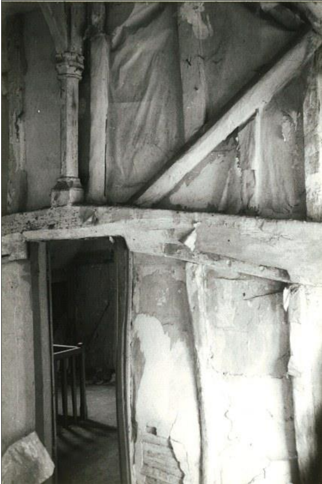
Crown post and tie beam of the hall before repairs. The tie beam beneath the crown post has been cut to give head room and the crude work of the inserted partition on the line of the open truss can be seen very clearly to the right of the crown post.
