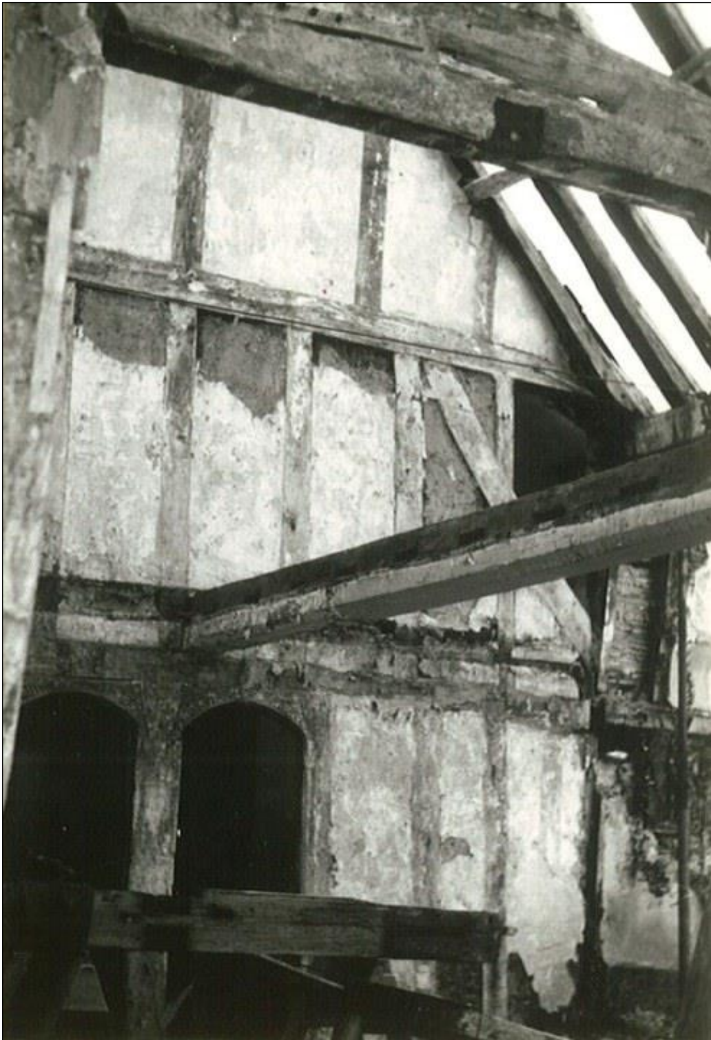
The interior of the hall during restoration looking towards the low end, with an iron girder that latterly supported the first floor still in situ. Panels of 15 th -century wattle and daub were retained in this wall.
