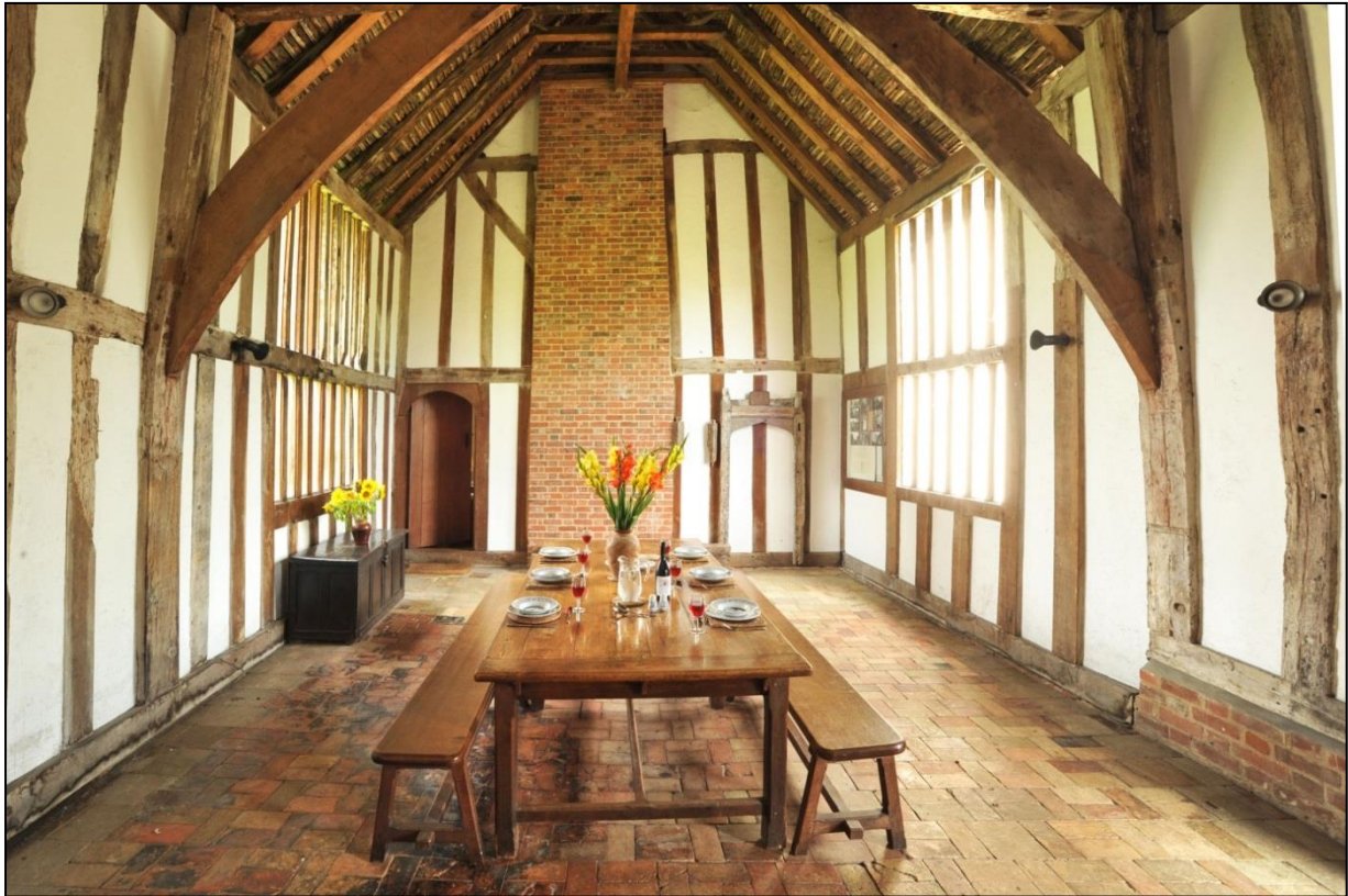
The hall at New Inn before the 2013 refurbishment. Note the underside of the clay roof tiles open between battens between the rafters. The brick panel indicates where the lost inserted stack cut through the timber frame – and, like it, helps support the building.
