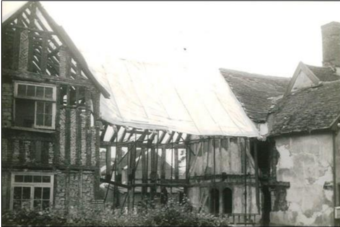
The hall stripped back to its frame. The service doors to the low end can be seen in the right hand wall. Note the neat brick infill to the first floor panels.
