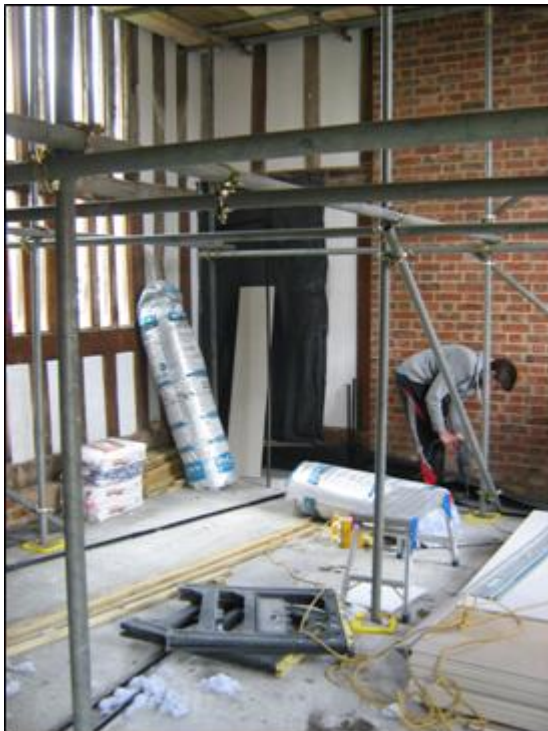
To gain access to the roof structure in 2013, the whole hall had to be scaffolded and a 'floor' once more inserted – but this time only a temporary one.
