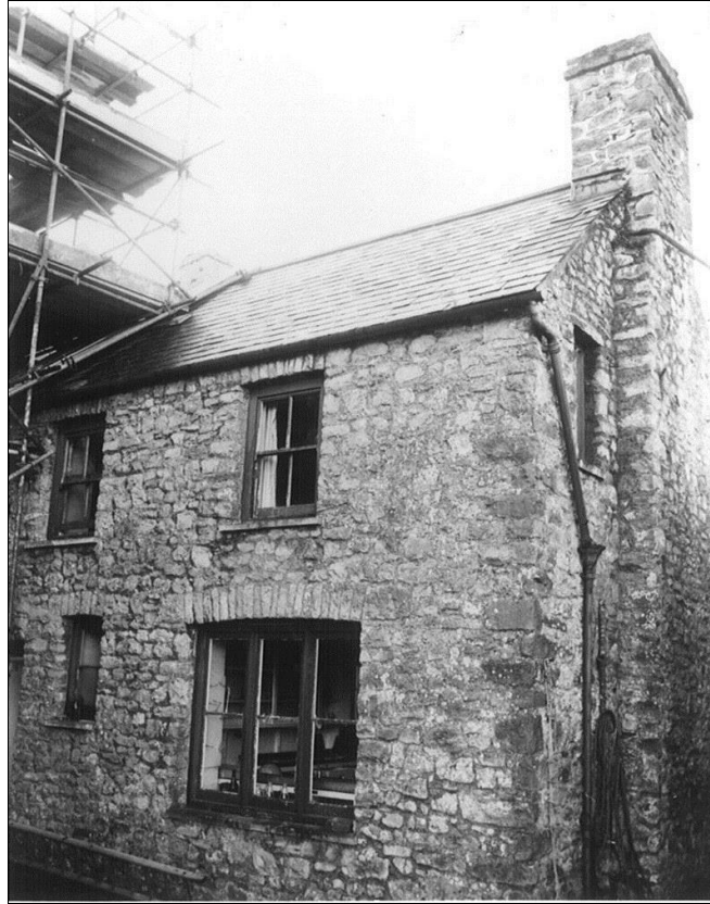
Demolished north west wing form the courtyard.
