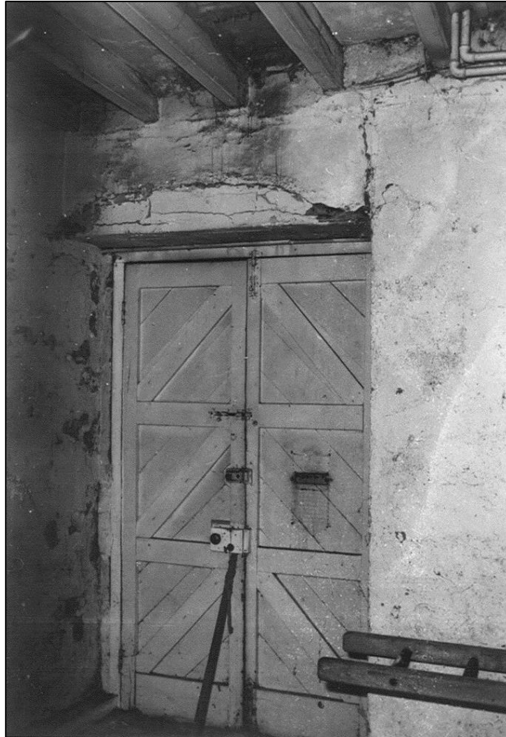
The former front door in the south east wing. You can see damp penetrating the walls causing damage to the plaster
