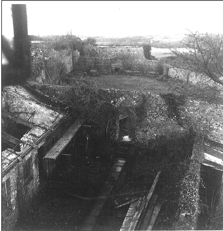
Demolished potting sheds.
