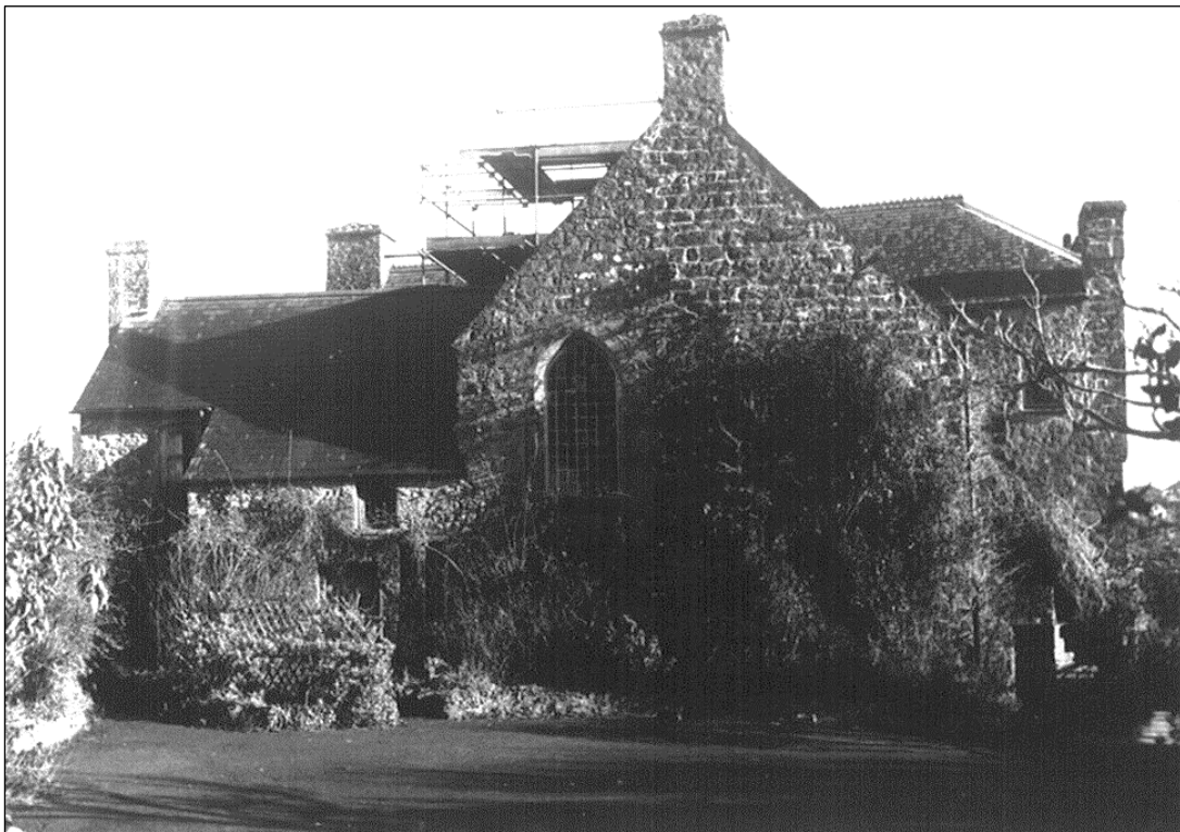
View from the west, with the demolished wing on the left and the former entrance into the SE wing on the right.
