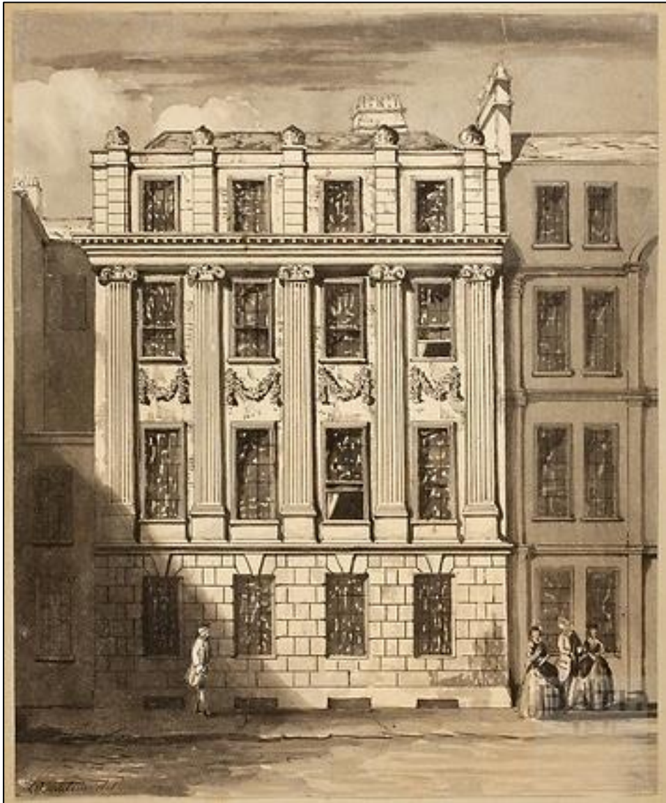
An imaginative (and quite incorrect) reconstruction of the ground floor, drawn by Lansdown in the mid 19 th century.
