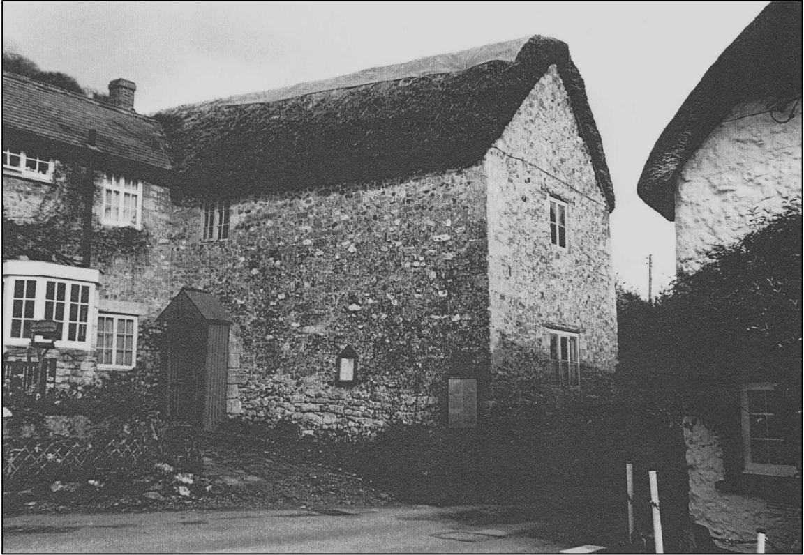
From the north west. The corrugated iron porch was removed.
