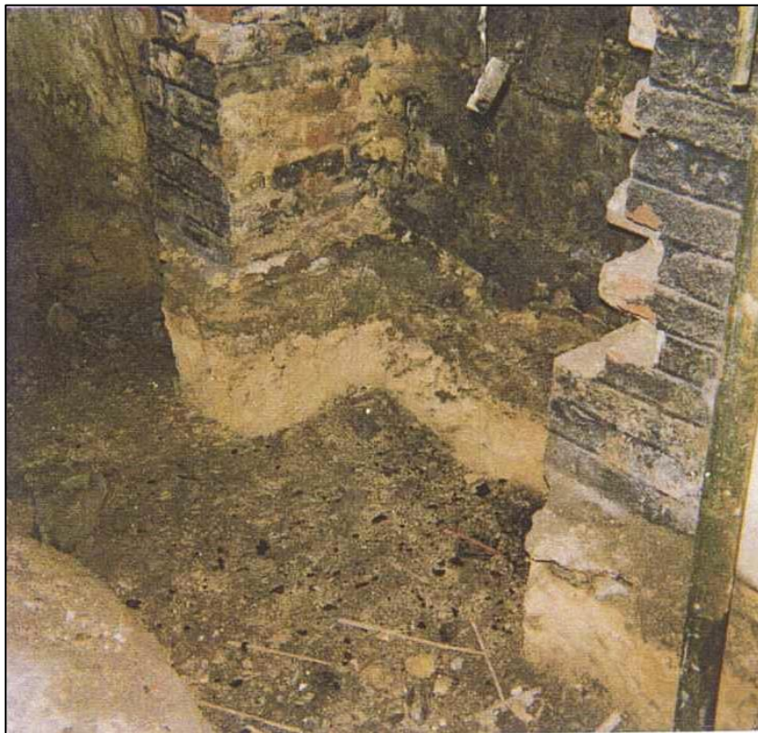
Opening up the kitchen fireplace.
