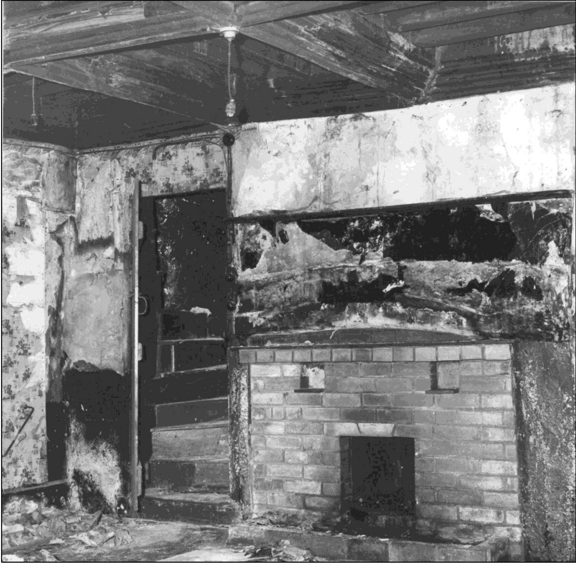
The bricked up fireplace in the sitting room.
