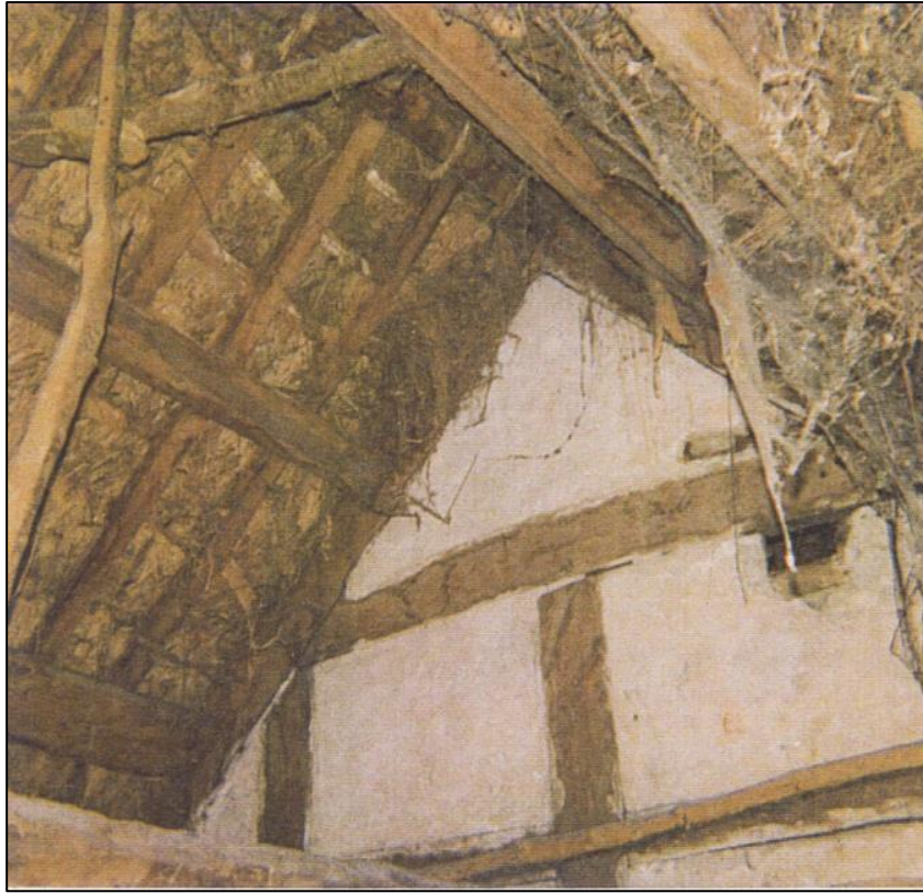
The underside of the thatched roof.
