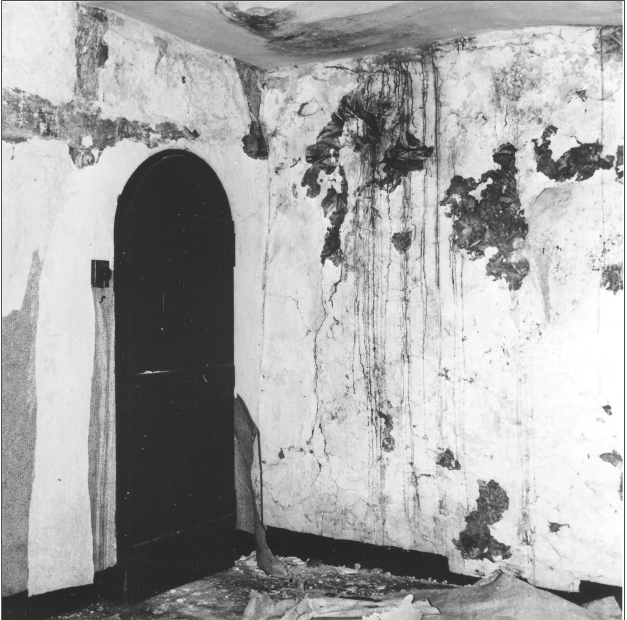
Traces of the wall painting in the south bedroom before restoration. The ceiling is visible at the top. (C L Hines).
