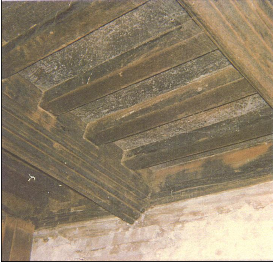
The sitting room ceiling
