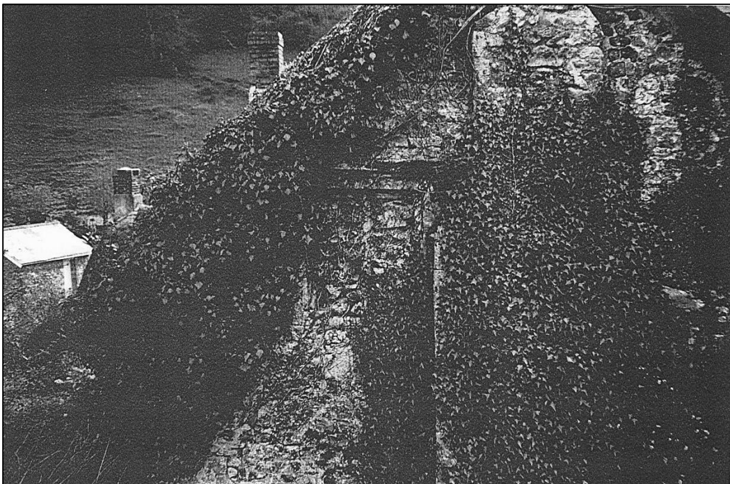
The blocked up east window
