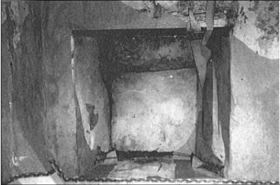
The blocked up east window from inside
