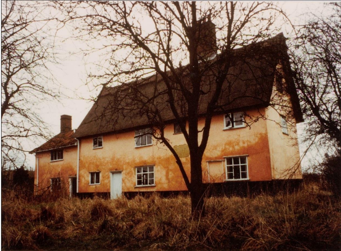
Manor Farm in 1979. The clay plaster had suffered from damp and was breaking up in a number of places.
