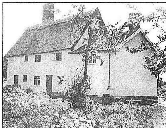
Manor Farm after the completion of repairs.
