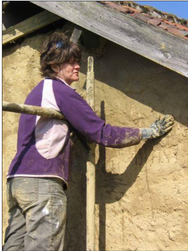
Kate Edwards daubing the gable and barn still to receive its tarred finish (below).
