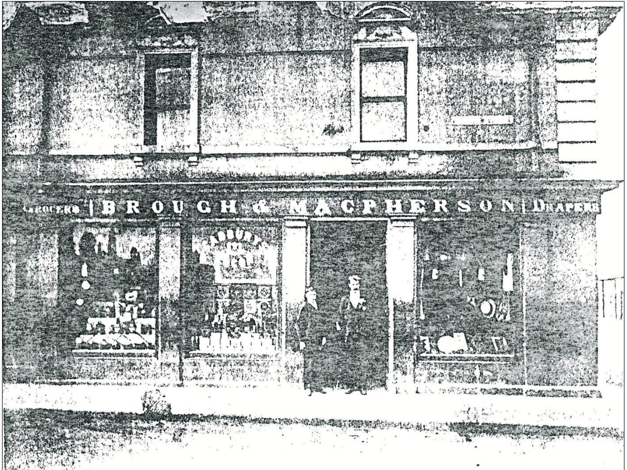
(1.2(c)) Detail of shopfront.
