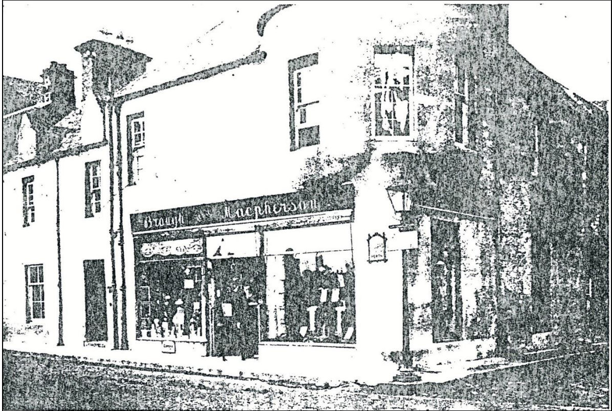
(1.3(a)) Early photograph of building (above). (1.3(b)) General view from across the river Earn (below).
