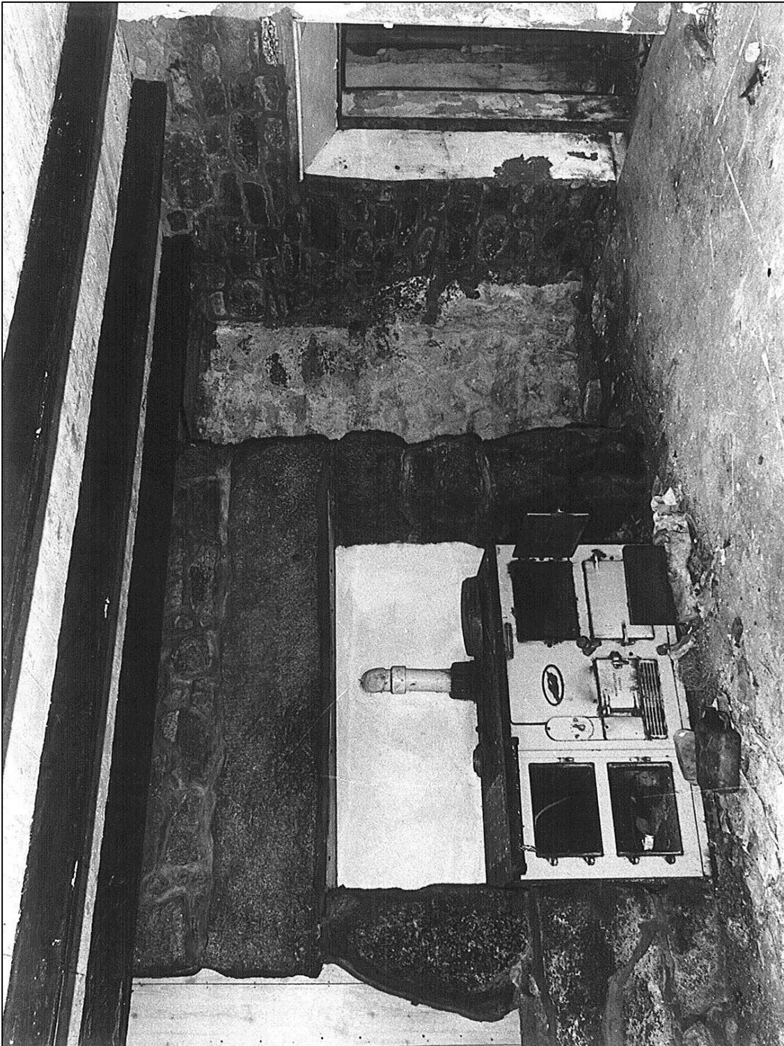
The great stone fireplace lintel is characteristic of many Penwith houses; this one has now been tamed with a wooden surround. The door into the dairy (more recently scullery) has been blocked.
