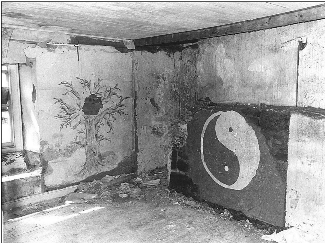
The west bedroom. Squatters had been living in the house and left behind their rather superior graffiti
