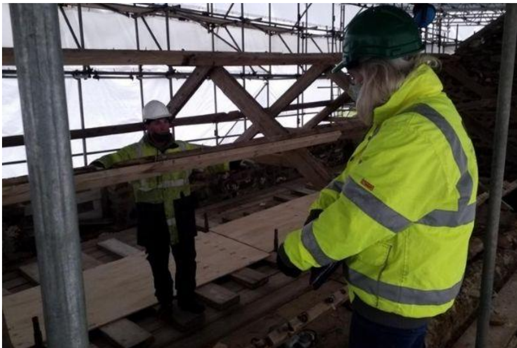
Contractor Paul Carter and structural engineer Kathy Gee in conversation under the scaffolding that enclosed the roof structures.
