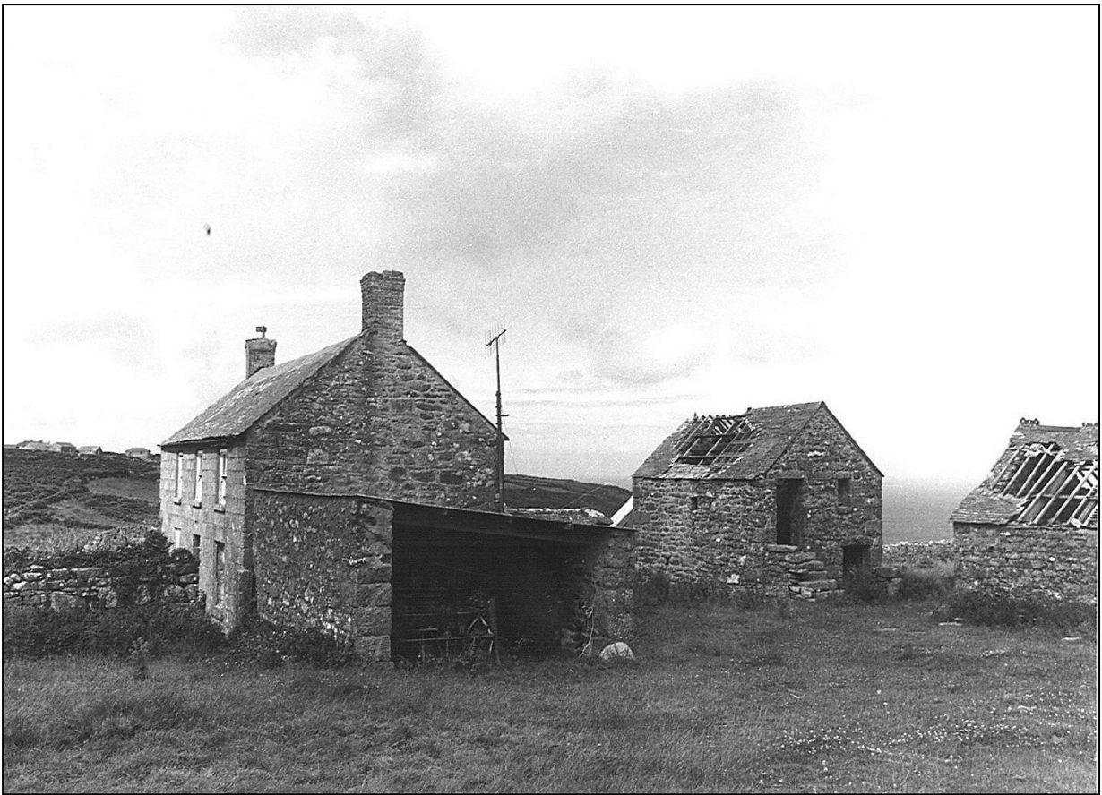
Robert Berryman's barn and (on the right of the picture) Four-house, with cart-house on the end of the Inside House, taken down in 1988
