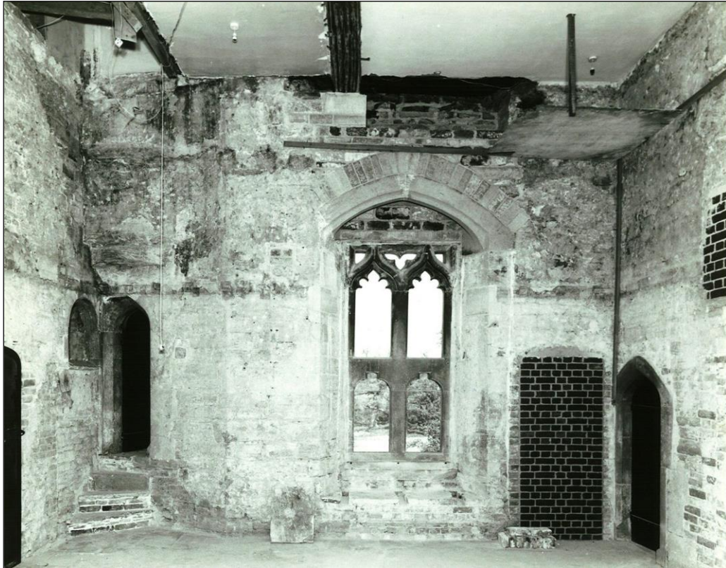
The partly restored King's room, with later openings blocked, the window arches renewed but the walls bare of all except medieval plaster. The line of the hacked off corbel table can be seen above, disappearing above the attic floor.
