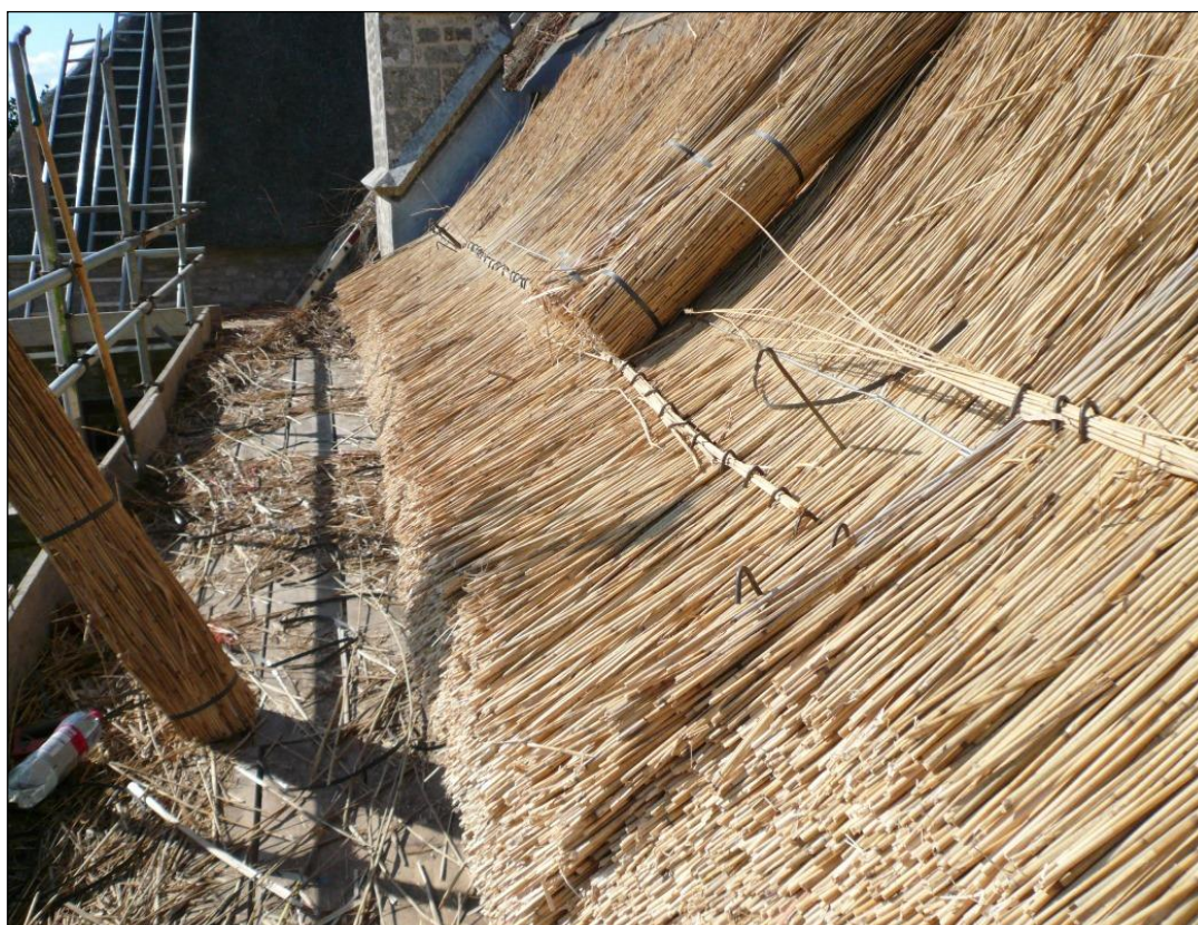
Re-thatching work in 2009. The total depth of the thatch is 350mm.
