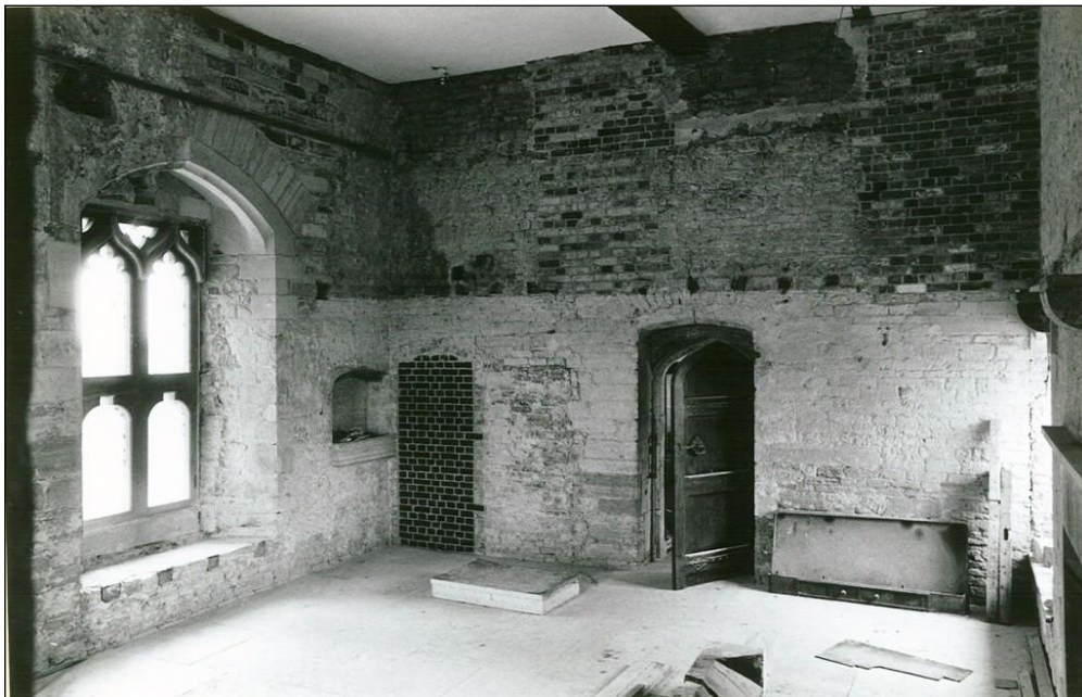
The partly restored King's room, with later openings blocked, the window arches renewed but the walls bare of all except medieval plaster. The line of the hacked off corbel table can be seen above, disappearing above the attic floor.
