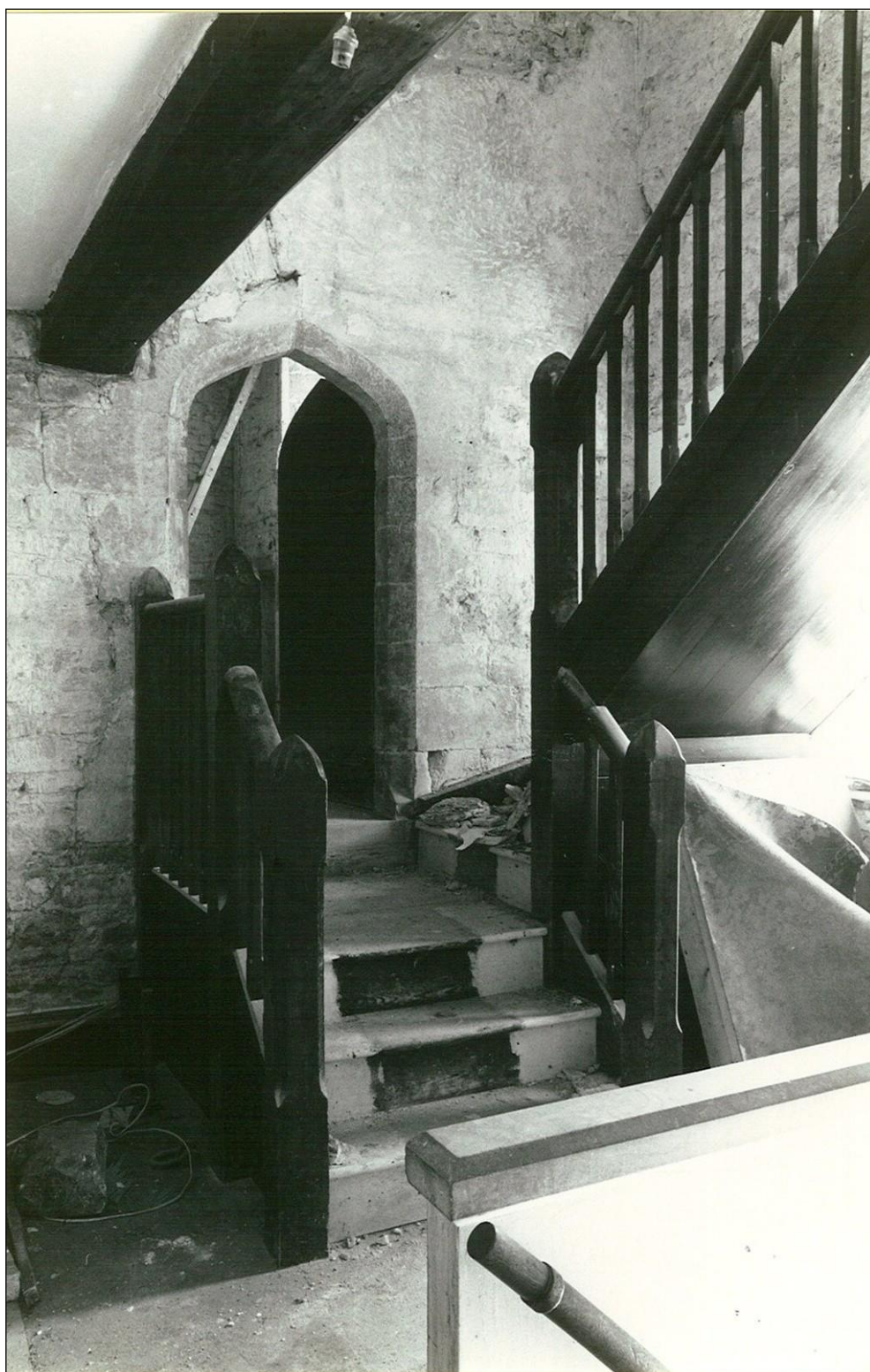
Hick's staircase in the chapel lobby
