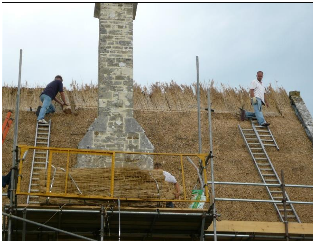
Re-thatching work in 2009. The total depth of the thatch is 350mm.
