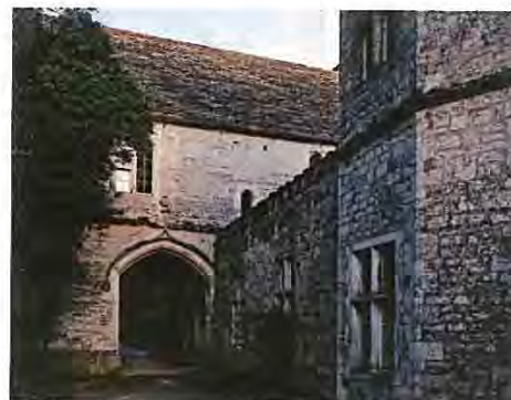
2—The interior façade of the gatehouse, viewed from the courtyard of the house
