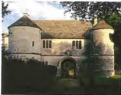
1—The exterior façade of the gatehouse. The roofs and towers give the house a French air
