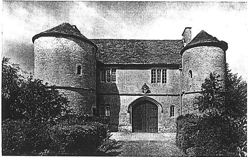
1.—THE GATEHOUSE, WITH ITS TWO DRUM TOWERS, FROM THE EAST
