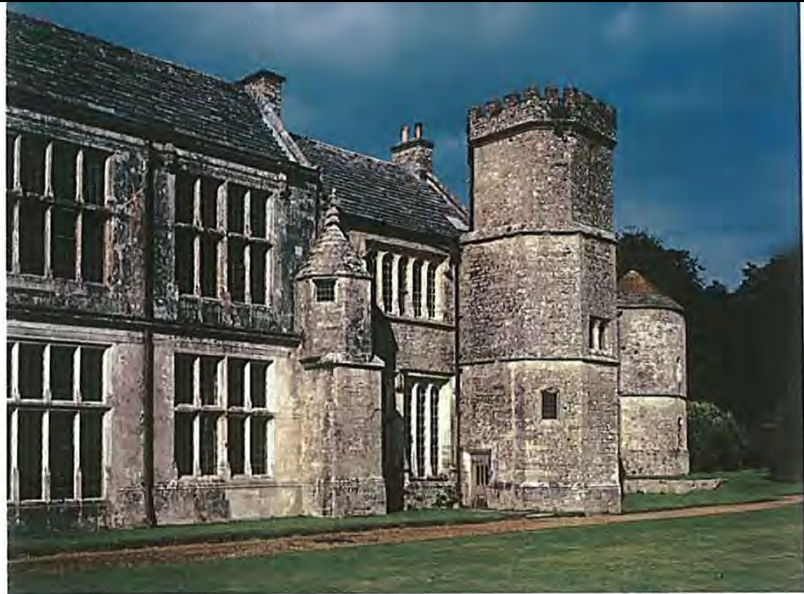
4—View of the south range. To the right are the latrine and stair towers of the 1530s house
