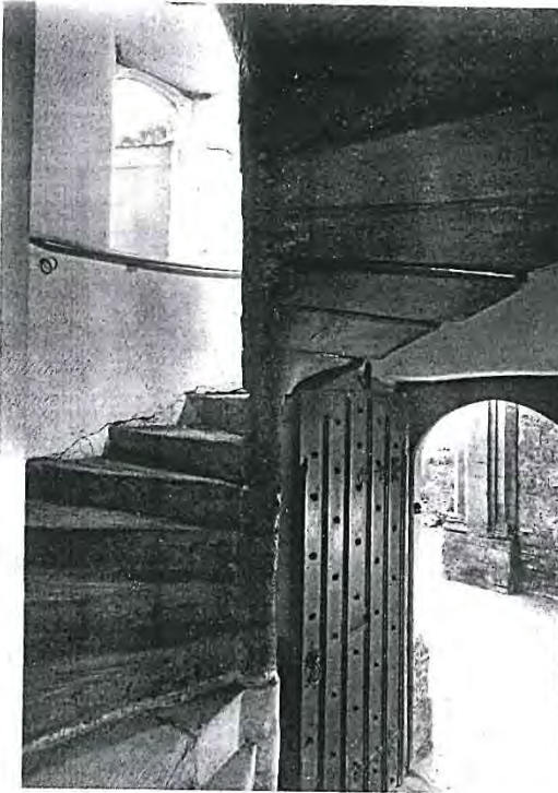
7.—WINDING STAIR MADE OF BLOCKS OF OAK IN THE GATEHOUSE
