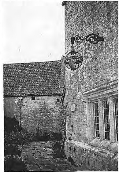
South face of the 17/18th century end of the house.
