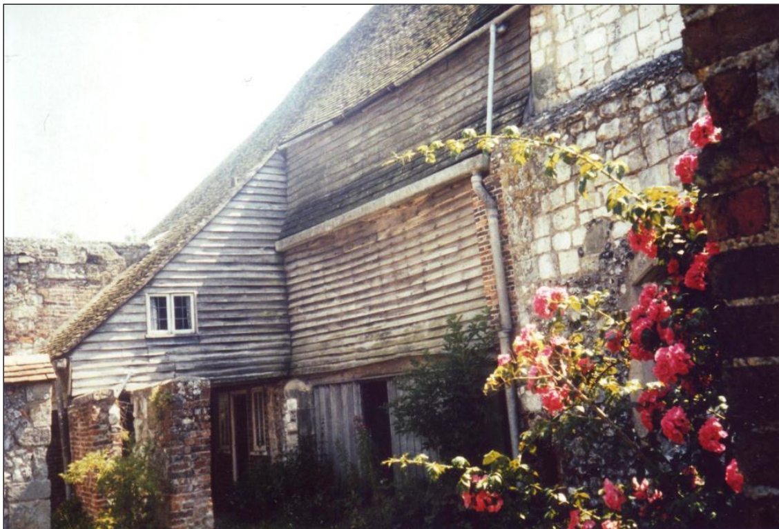
The north wall of the kitchen before alteration
