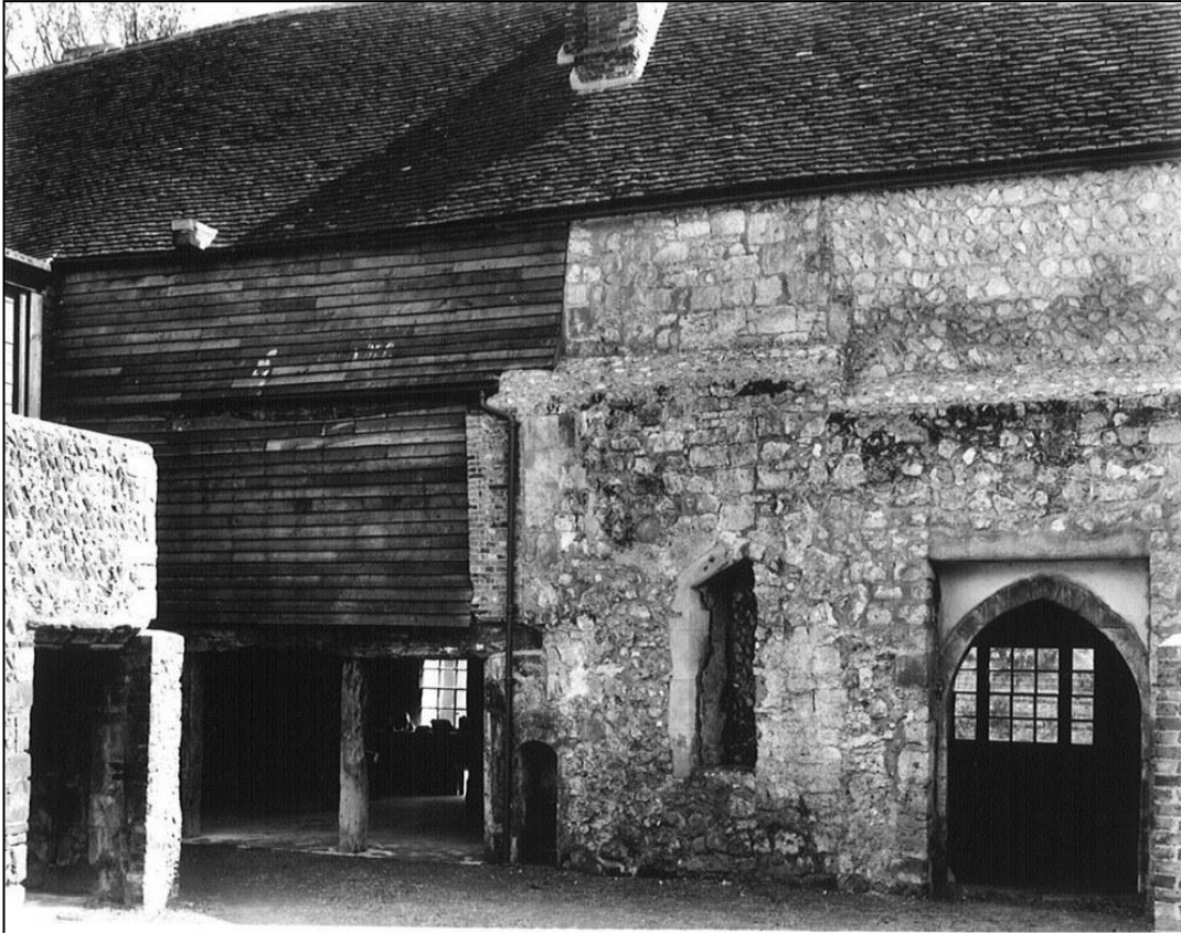
In the centre is part of one of the original south windows of the old hall. The offset above marks the original height of its walls (NMR)
