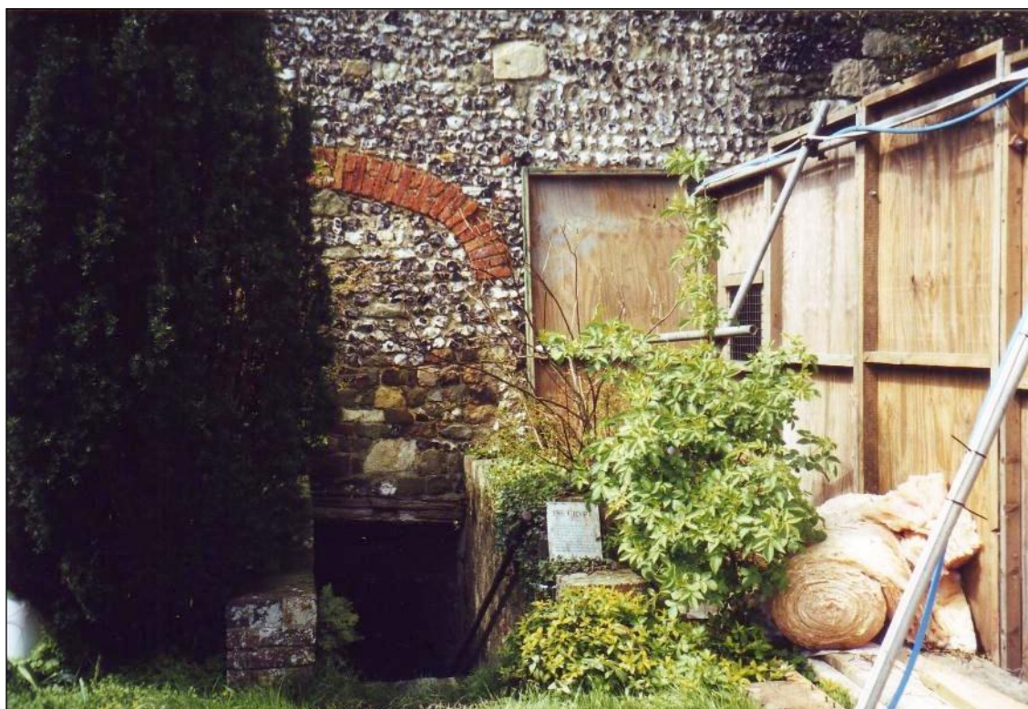
The stairs to the undercroft created by Walter Godfrey in 1925
