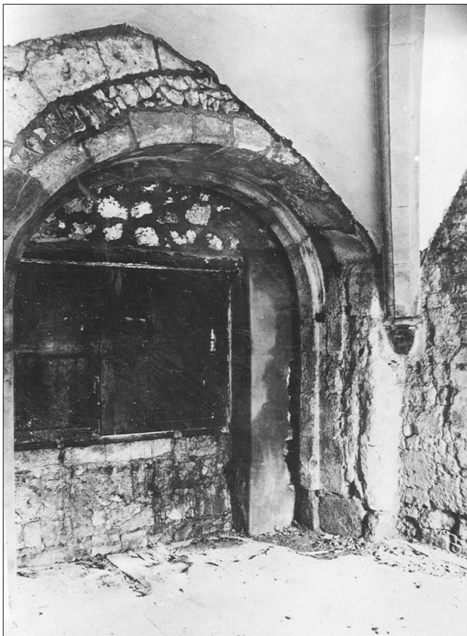
The interior of the original entrance into the porch. It shows how the later vault cuts across the entrance arch (NMR)
