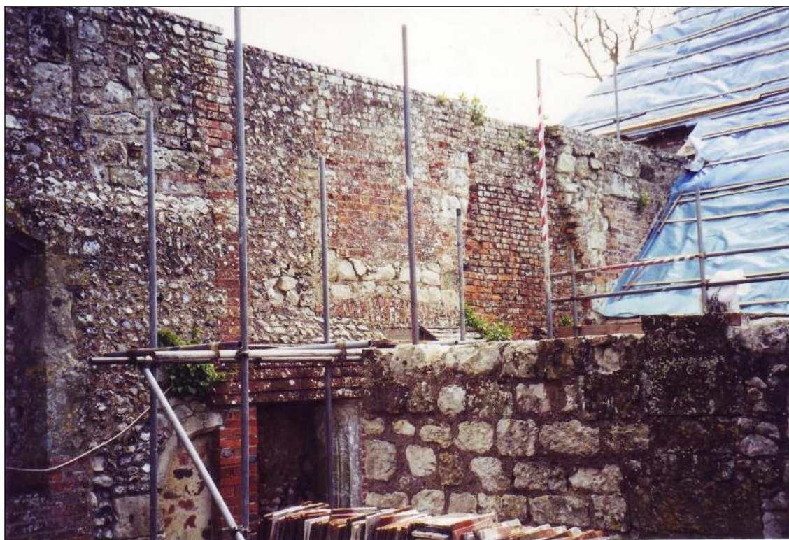
Well House Court showing the original entrance to the undercroft
