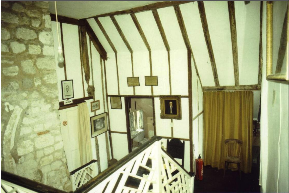
The landing before removal of the custodian's bathroom
