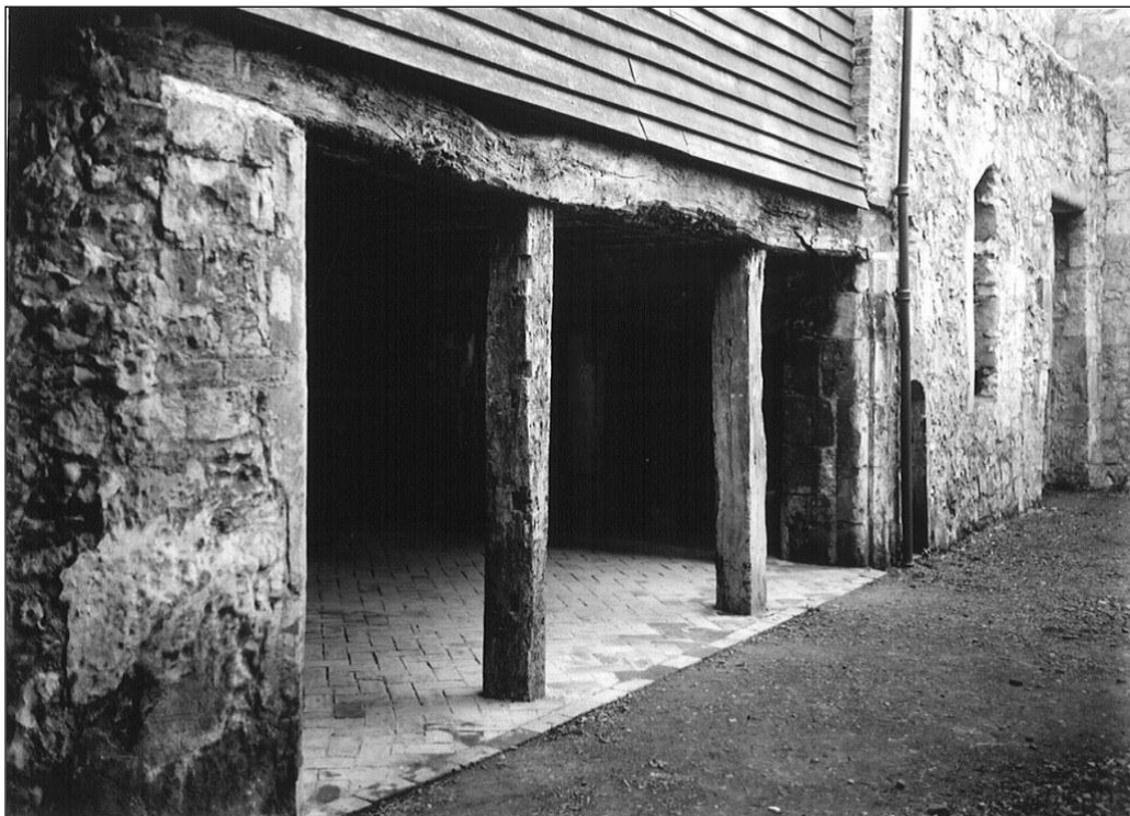
The kitchen wall before the museum was created (NMR)
