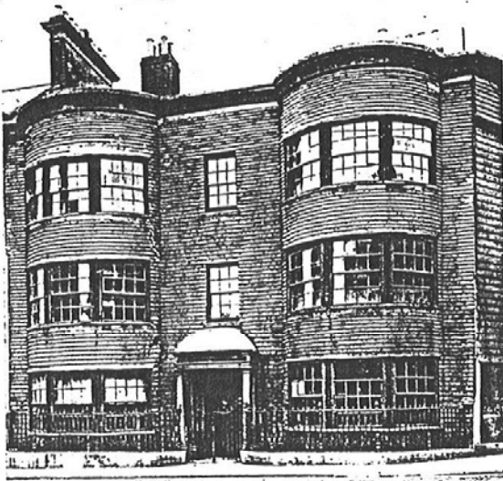
NELSON HOUSE, ST. AUBYN STREET, DEVONPORT. 1775.
