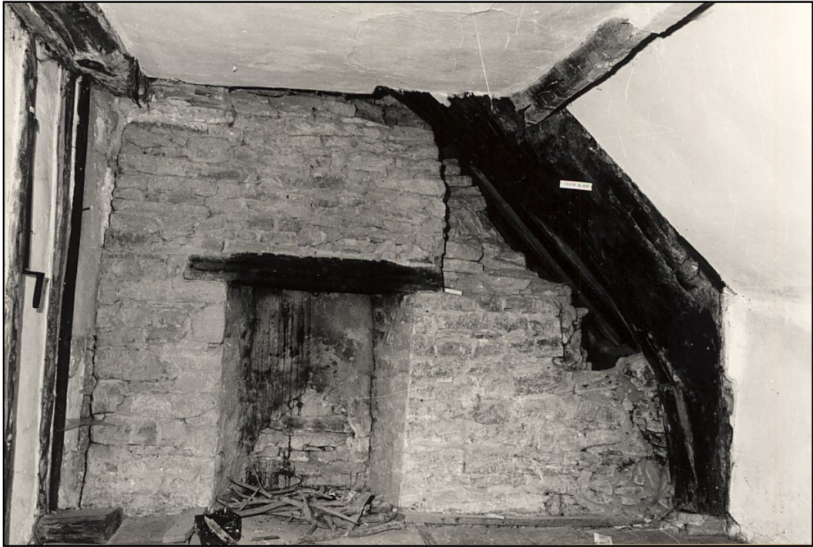
The Men's Room – chimney wall
