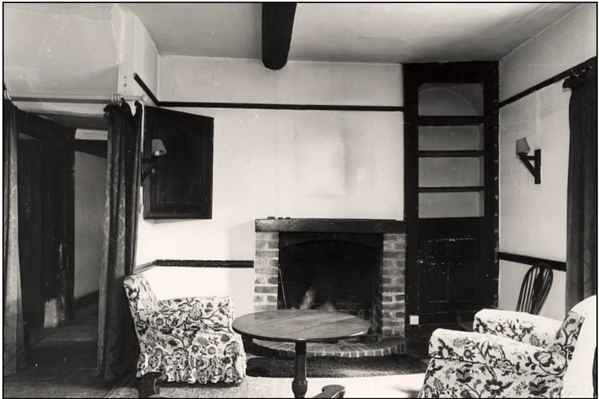
The sitting room – the partitions have been reinstated.
