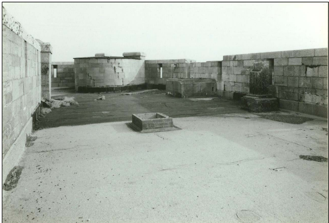
The concrete mount for the 3 pounder Q.F. gun is against the parapet on the right (NMR)
