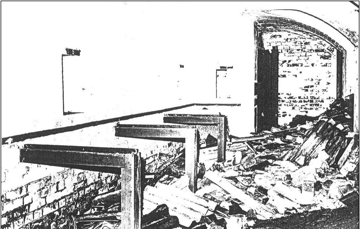
Interior of the shell store of B3, 6 inch magazine
