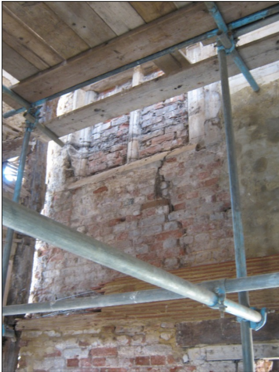
Left: The façade had severe cracking, which required tile-stitching inside and out. Right: The unusually stout surviving laths used to reinforce security of the ground floor. When such panels failed, they had been replaced in the past with brick.
