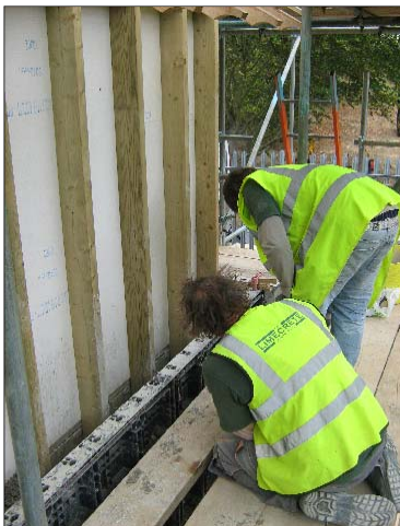
The hempcrete walls of the rear extension rise between plastic 'shutters', used to form the structure as the mixture of lime and hemp hardens. This new generation of sustainable building material offers excellent insulation, as well as breathability.
