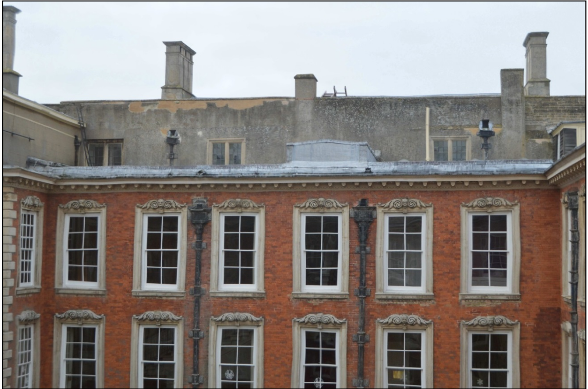
Kimbolton Castle, south elevation of the inner courtyard refaced by Henry Bell, 1690s. The high level windows are now the only fabric of the works to the Castle in the 1620s and 30s left visible by Bell's and later alterations.
