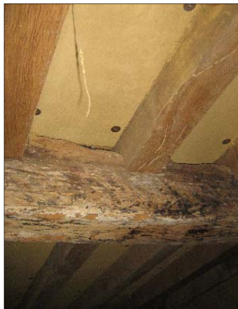
L to R: Clayboard floor above new oak ground floor joists; second coat plaster on the first floor; heaters prevented frost damage as the internal plaster dried during the winter. Below L to R: top flight of stairs going in; jamb to door onto porch; plastering the bedroom.
