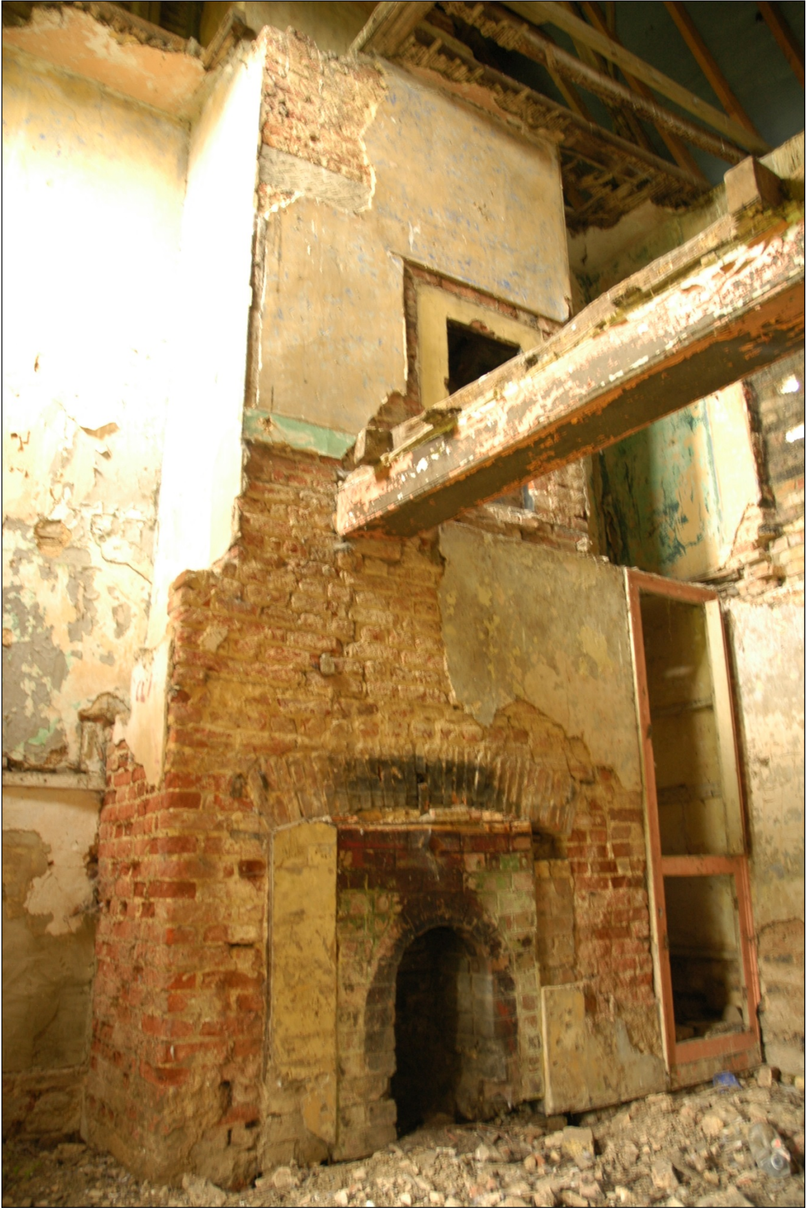
Inside the Warren House before restoration.
