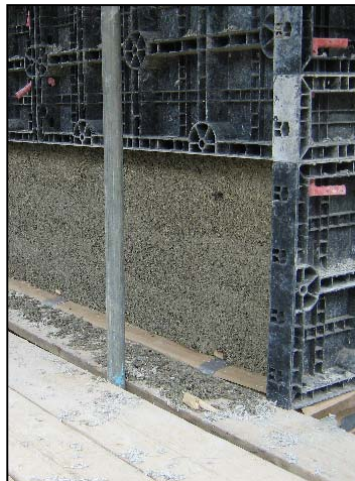
The hempcrete walls of the rear extension rise between plastic 'shutters', used to form the structure as the mixture of lime and hemp hardens. This new generation of sustainable building material offers excellent insulation, as well as breathability.
