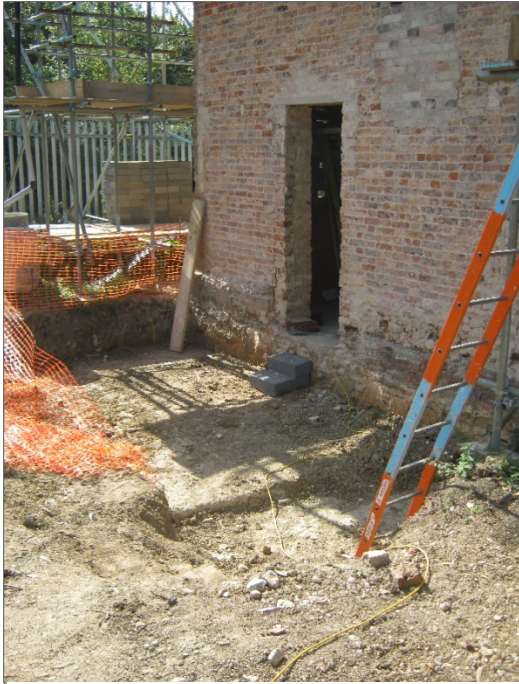
Excavations for the footings of the rear extension; bales of hemp shives; hempcrete mixed, and the kit for doing the mixing.
