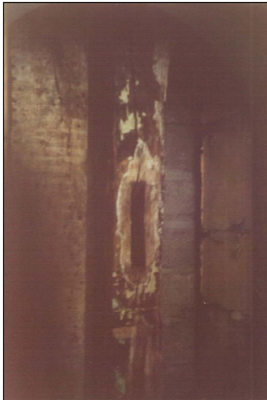
The possible late 14th-century aisle post, with its mortise slots, found in the Great Chamber. It would have been one of a series of such posts supporting the hall of the roof, and thus allowing a wider span.
