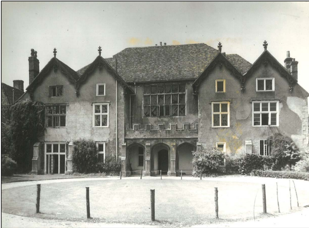
The Wardrobe in 1942, when occupied by the ATS. The 19th-century rendering was removed after the war. Some of the pendants and pinnacles of the 'ornamented' gables have also disappeared. During Landmark's restoration, windows were put back in place of French windows and the front door (NMR).
