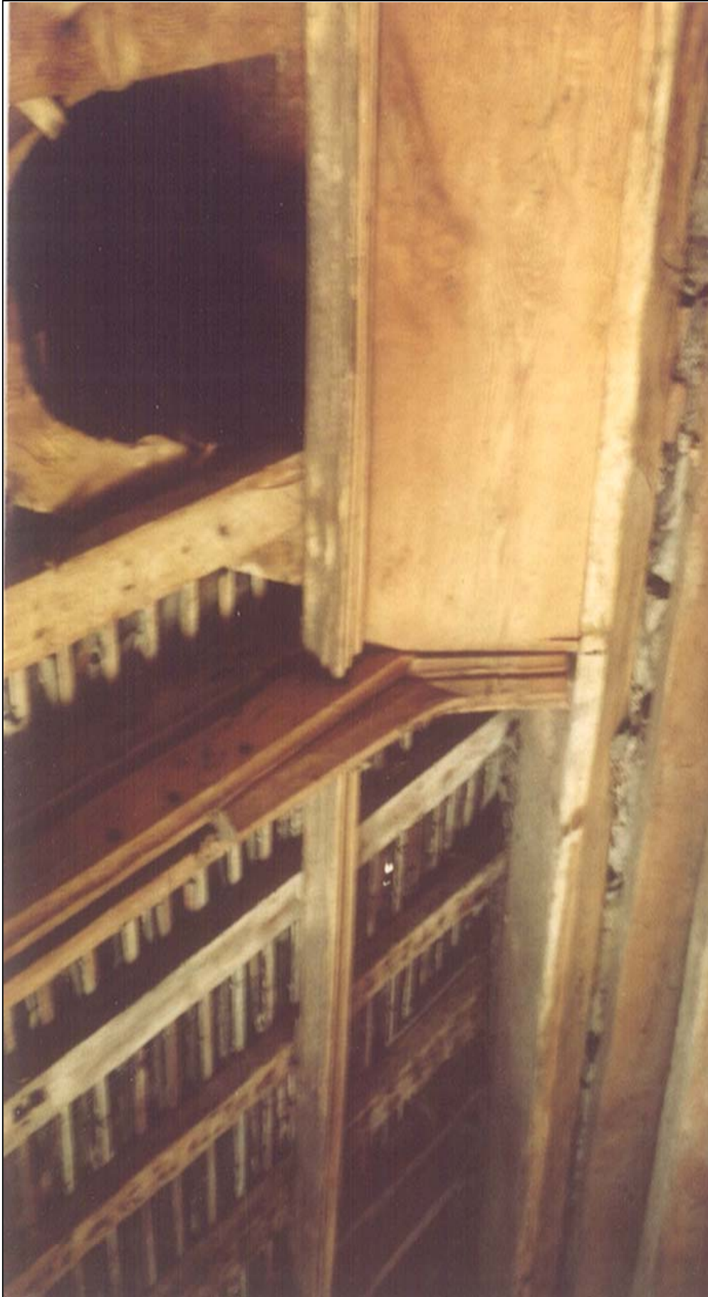
A section of the late medieval roof in the north wing, which shows the moulding on the beams, and a piece of wainscoting. This would have formed the ornamental open roof of the upper parlour.
