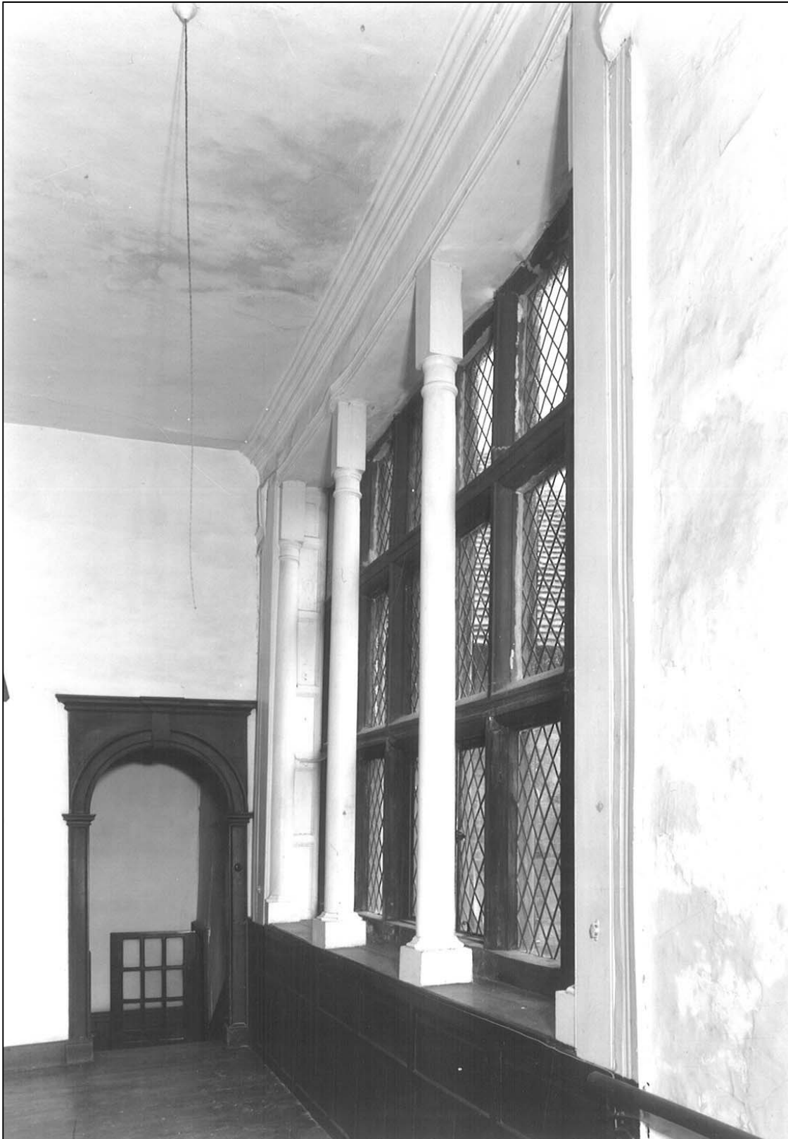
The width of the window in the Great Chamber was too much for its lintel, which had begun to sag in the 18 th century, and needed the support of columns (NMR).
