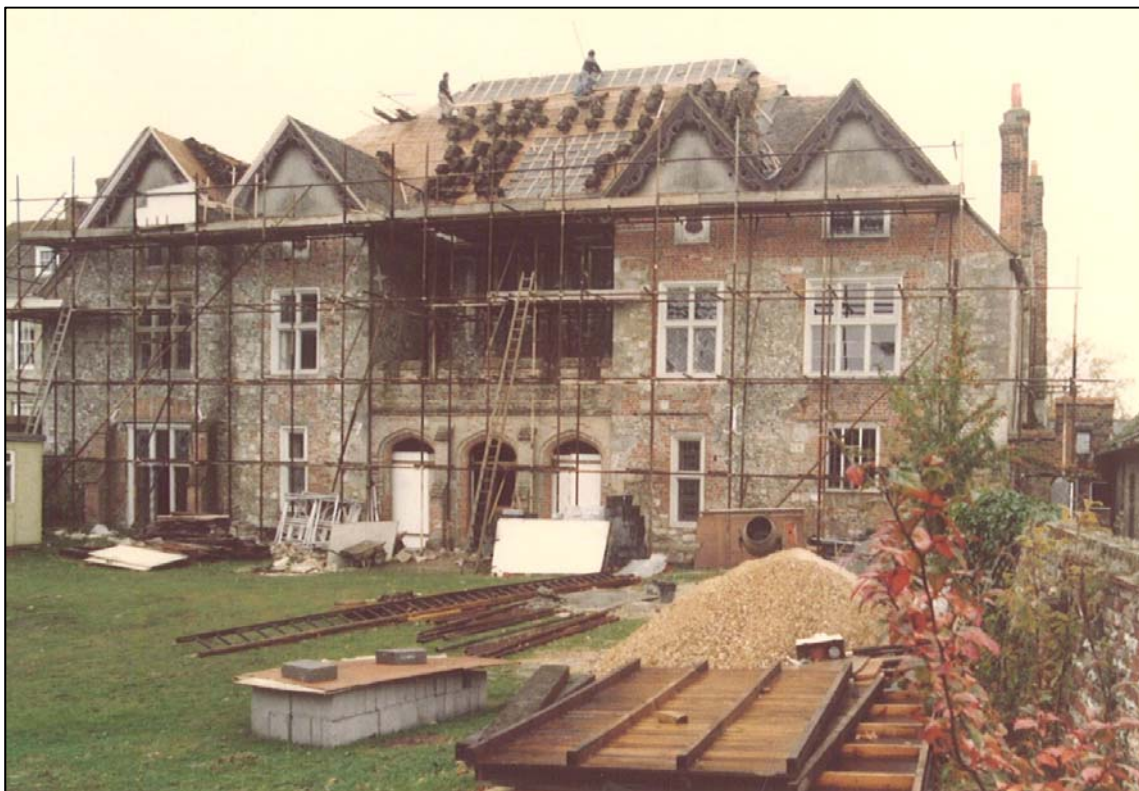
The roof undergoing repair.
