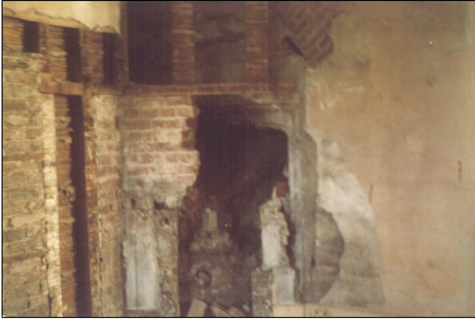
The original 17th-century fireplace was uncovered when the 18th century partitions were removed in the Great Chamber.
