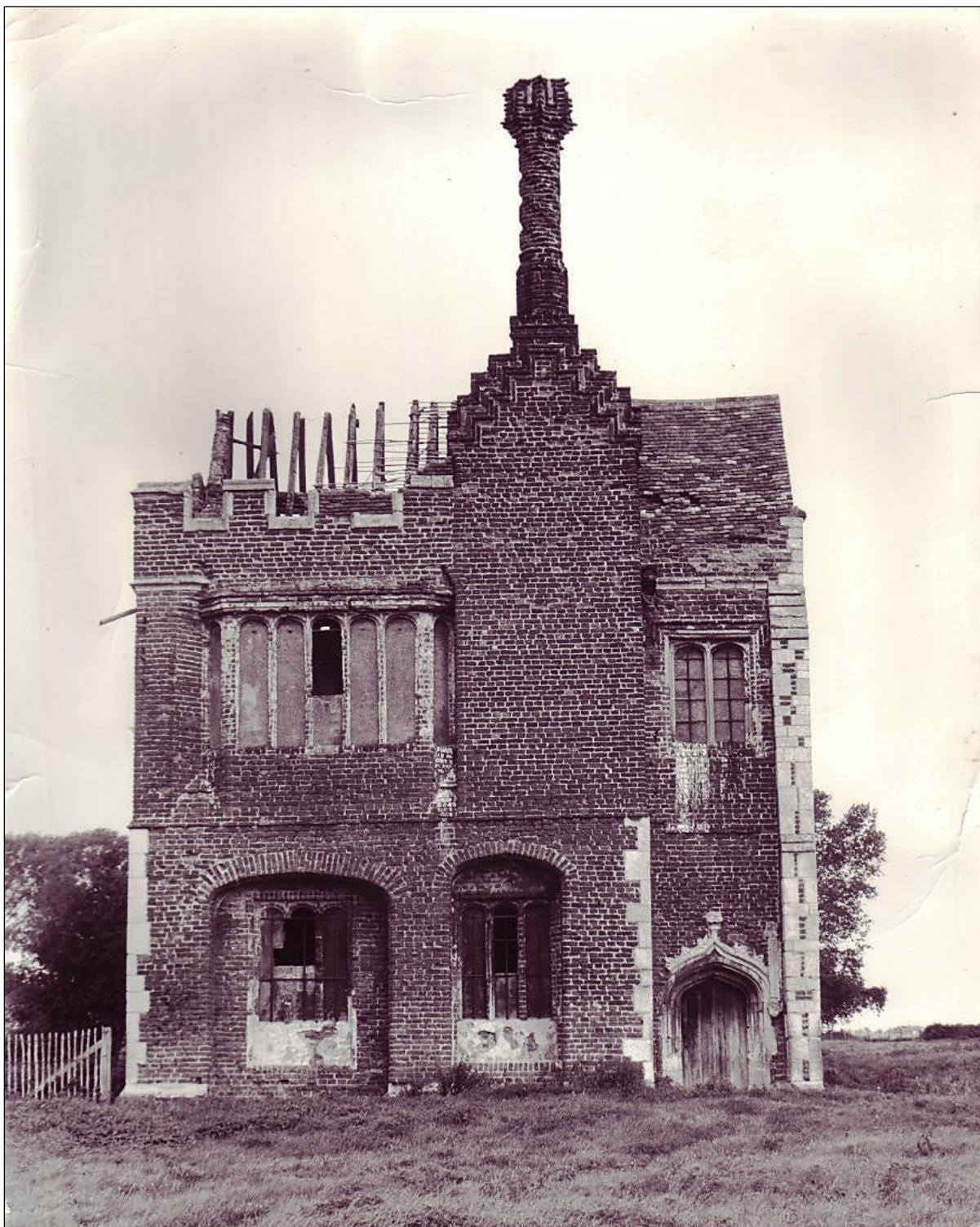
The south front in 1974 before work began. (BCC)
