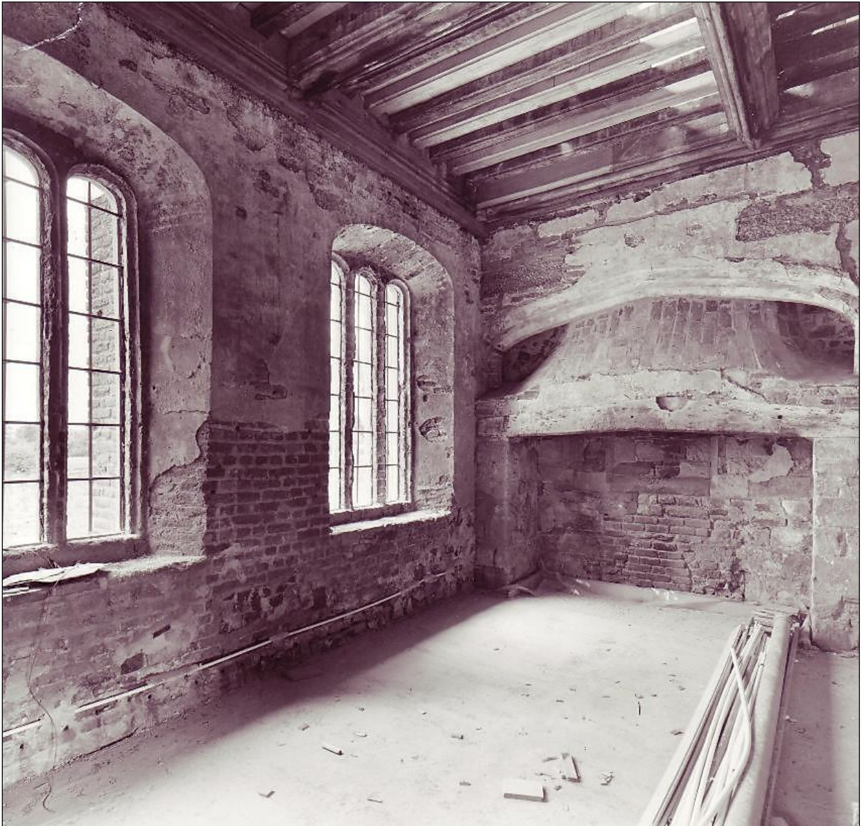
The sitting room during the renovation of Warden Abbey (BCC)
