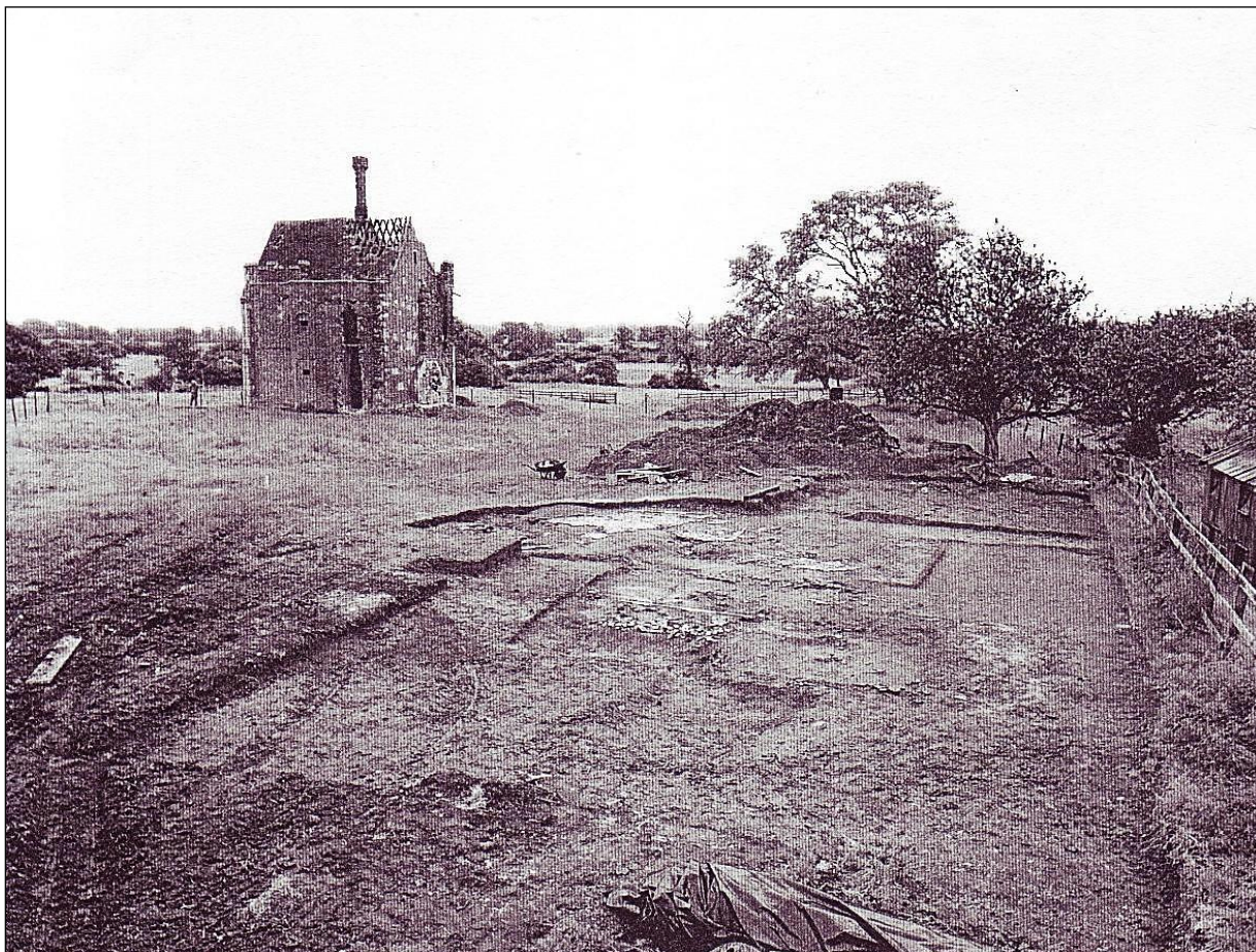
The first excavation of the abbey church in 1961. The roof was damaged by a fire in the late 1950s. The corner of the garderobe tower had collapsed (BCC)
