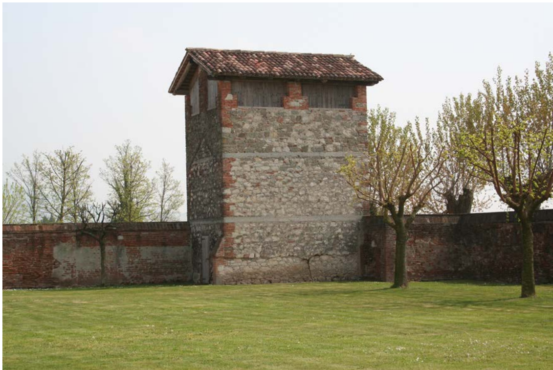
The silo tower, straddling the corte wall in the southwest corner.
