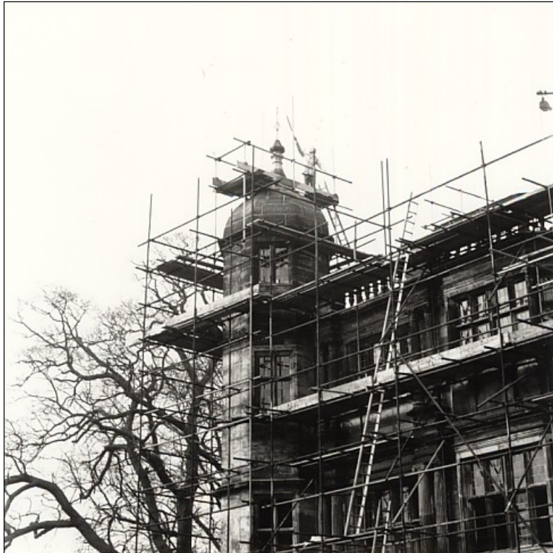
Trying out the stem of the new weather-vanes on a repaired cupola.
