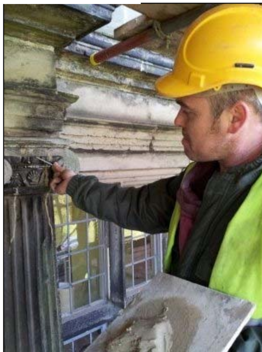
The ashlar blocks are beautifully dressed and fitted with very tight joints, making repointing a painstaking process.
