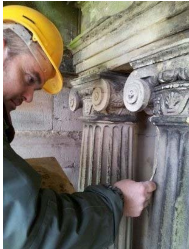
Cracking in the carved stonework called for fine grain filling with lime mortar.
