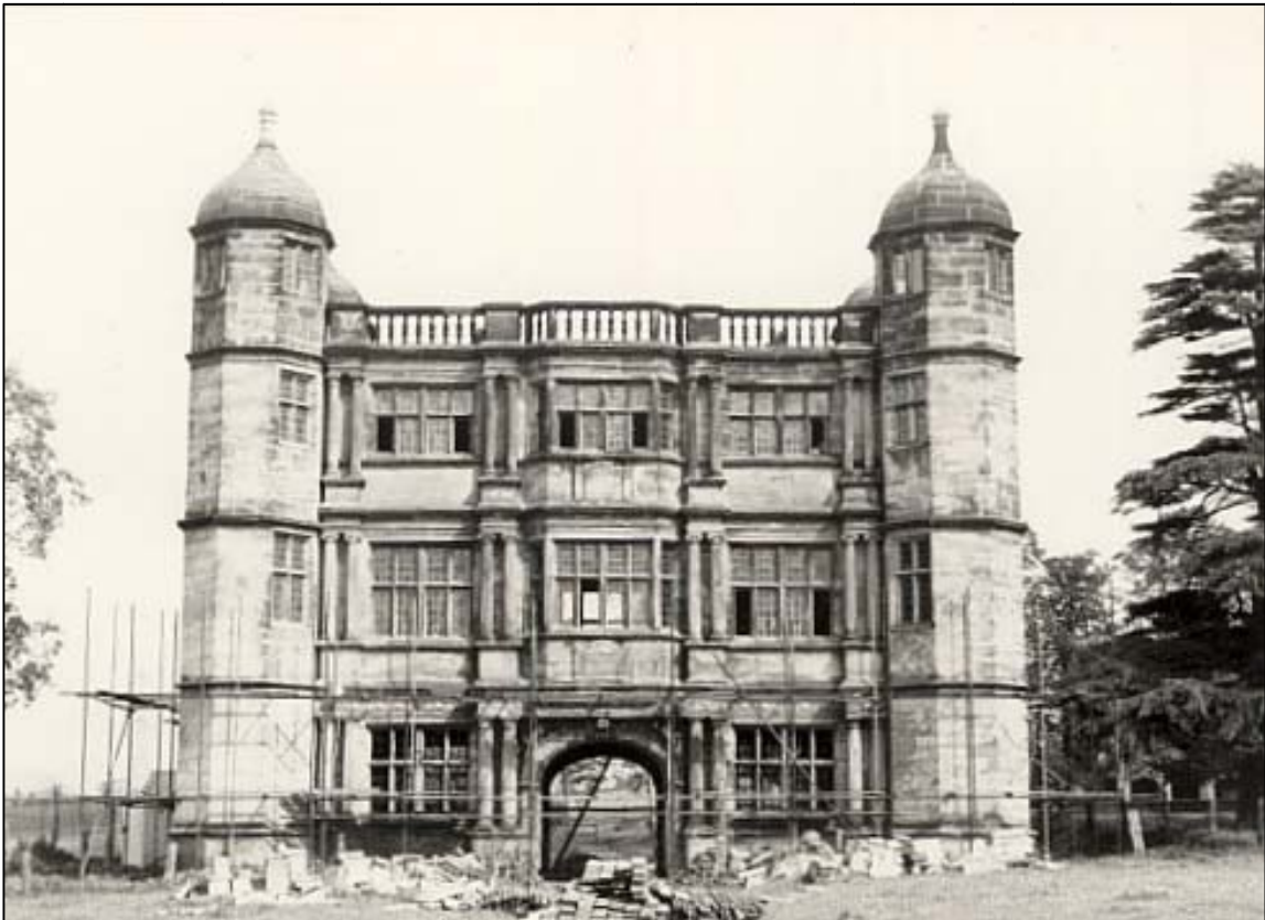
Scaffolding down, but some casements still to be fitted.
