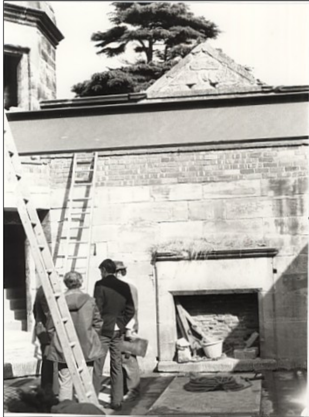
The second floor is finished and now awaits the roof.
