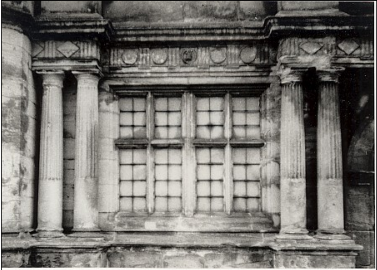
The ground floor windows had all been carefully blocked with Tixall stone.
