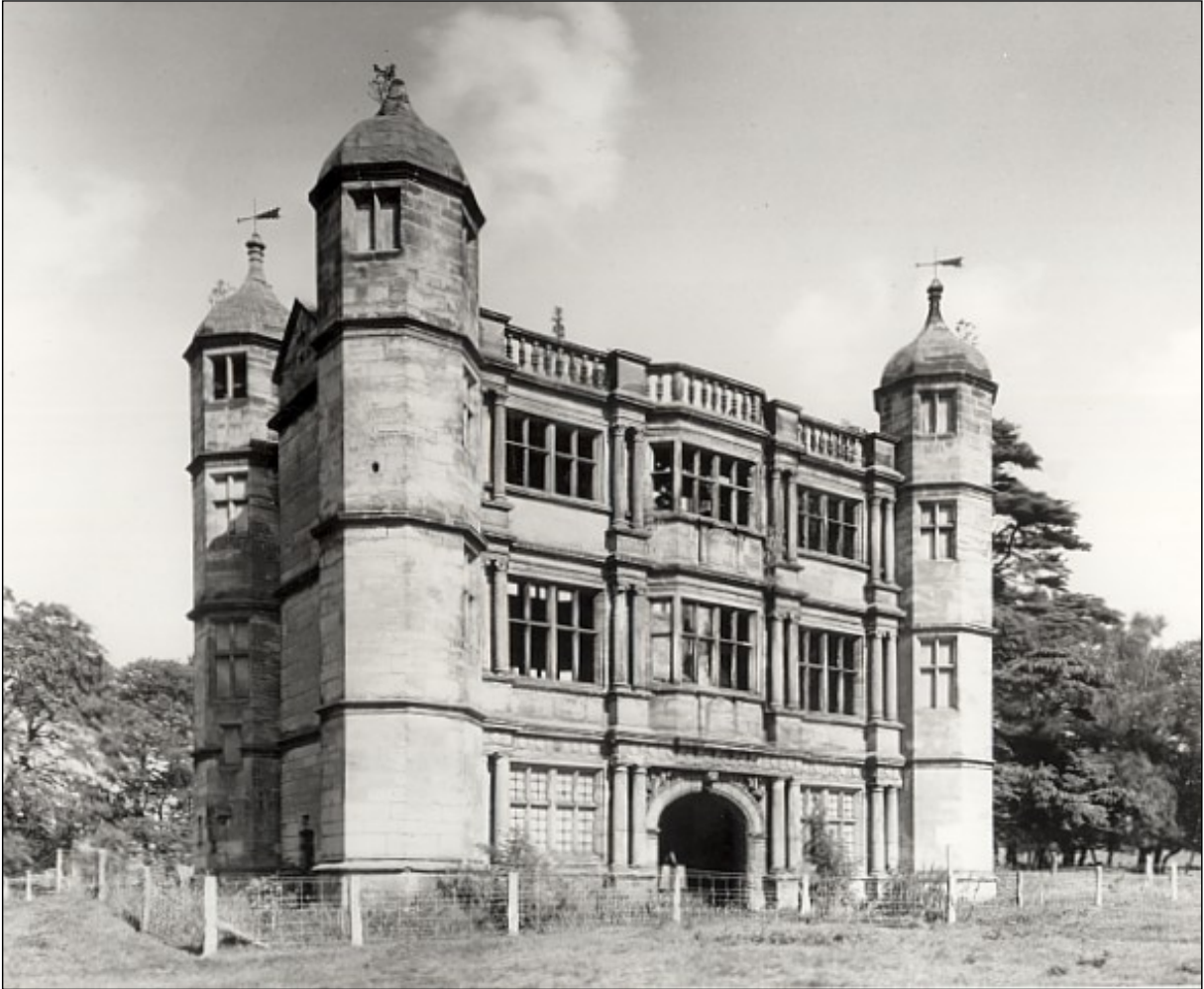
The Gatehouse in 1961, roofless and floorless as a consolidated ruin.
