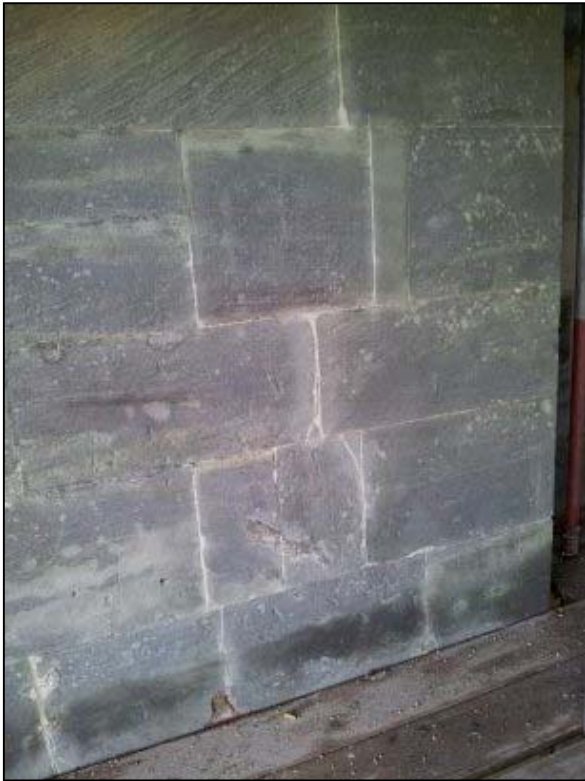
The ashlar blocks are beautifully dressed and fitted with very tight joints, making repointing a painstaking process.
