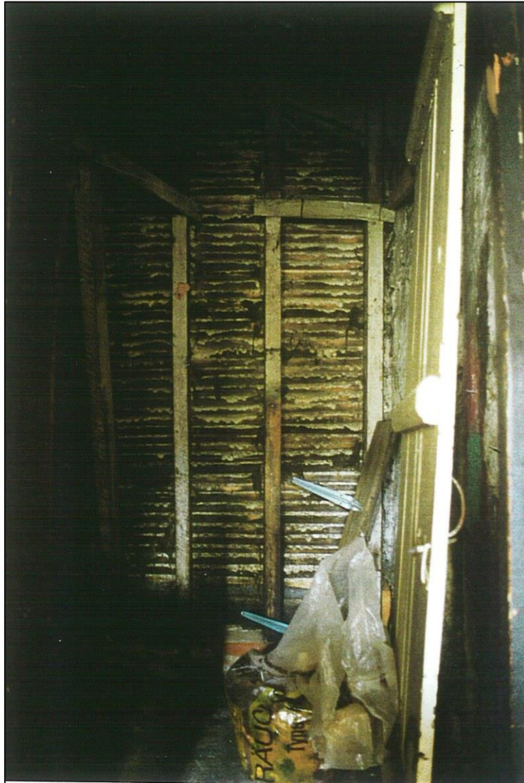
The back of the blocked front door before re-opening.
