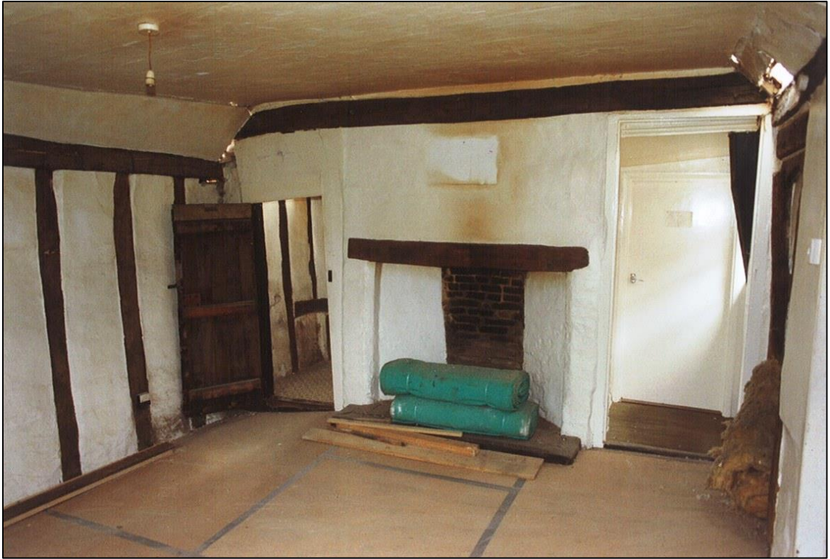
The chamber with its ceiling in the lowered position.
