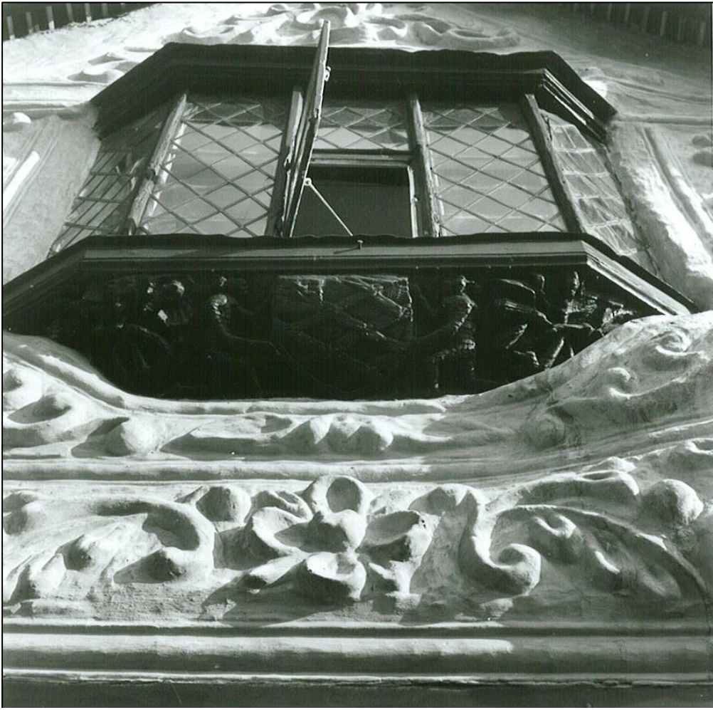
Carved bracket to the first floor oriel window showing the Hameldon shield supported by woodwoses.
