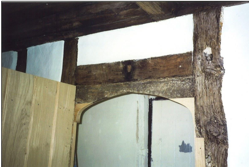
The original doorhead re-exposed and repaired.
