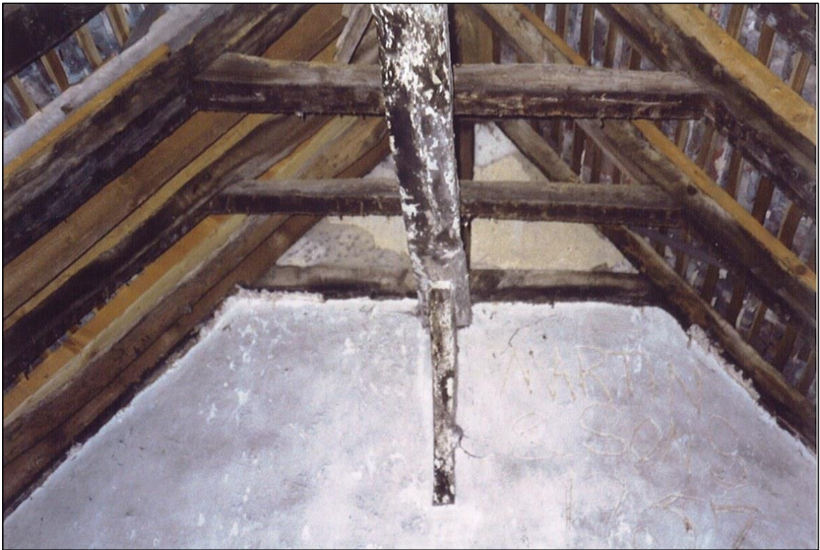
The collar purlin and ties exposed during repairs.
