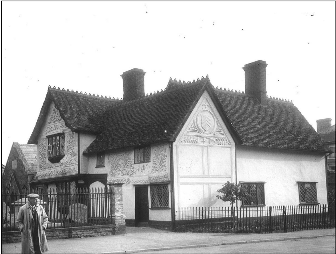
The 14 th -century 'high end' cross wing is in the centre; the late 15 th -century 'show' wing is on the left; on the right is the 17 th -century wing that replaced the earlier house (with its service wing which became a garden). (RCHME)
