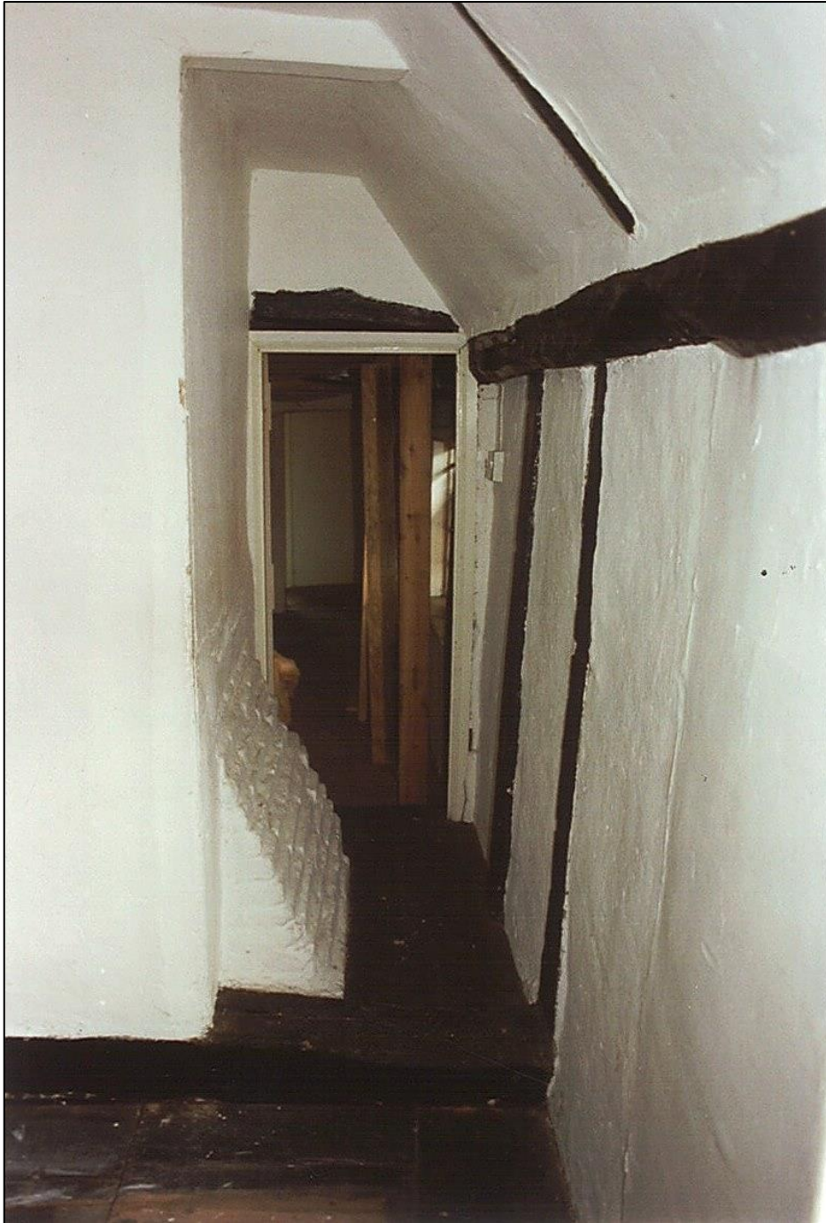
The passage way past the chimney stack above the Museum.
