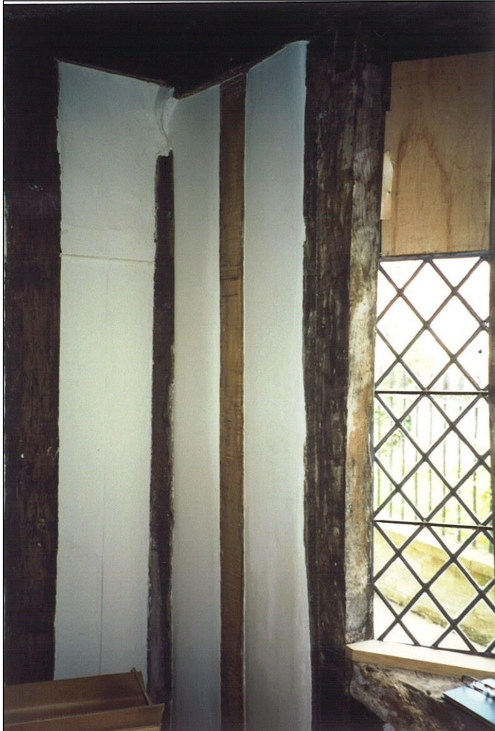
The old front door blocked and a new stud inserted.
