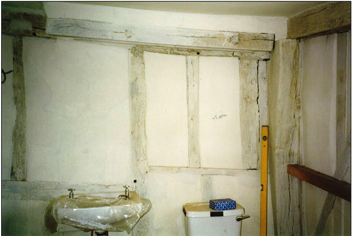
The east facing window in the bathroom was blocked up as below.
