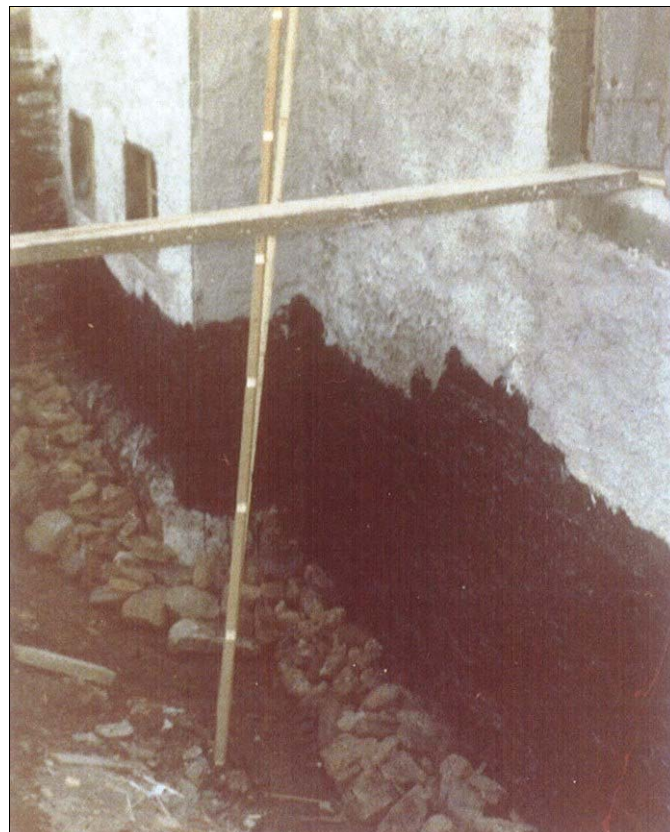
The trench at the front and external damp proofing
