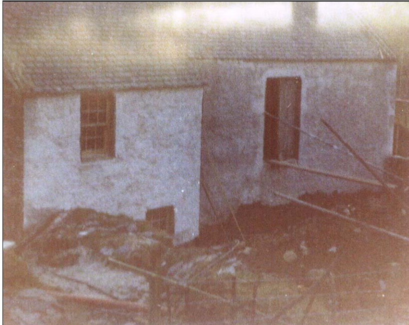
The trench at the front and external damp proofing
