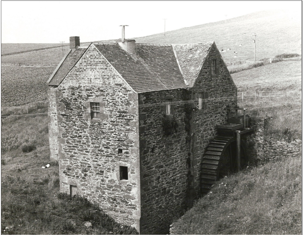
The mill before restoration
