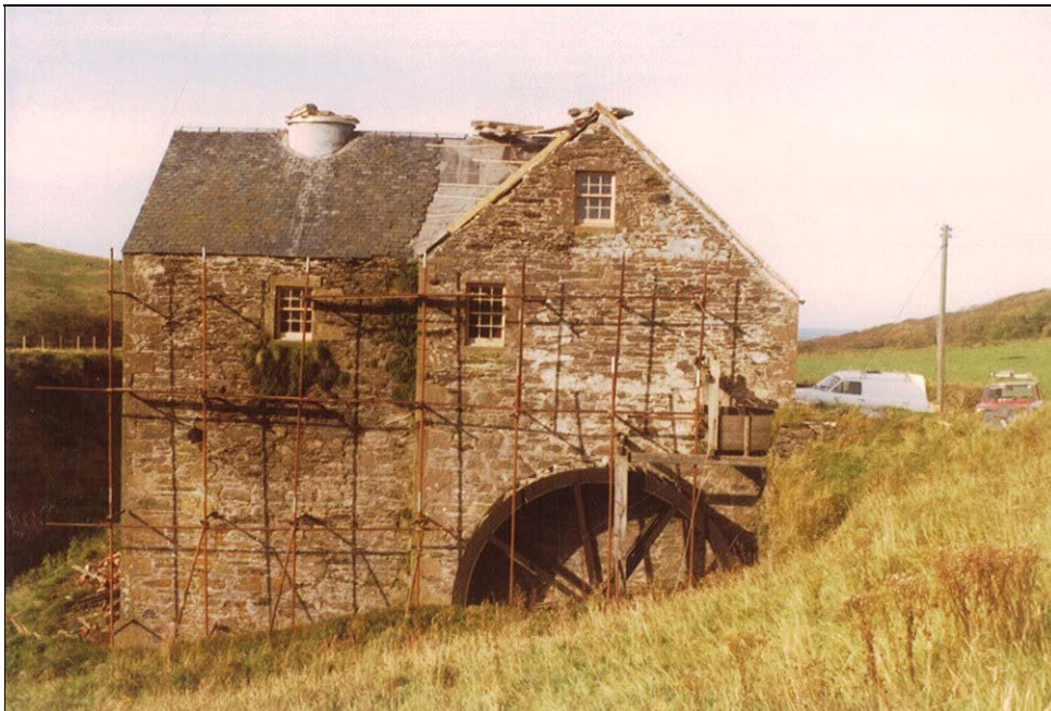
Tangy Mill at the start of renovation
