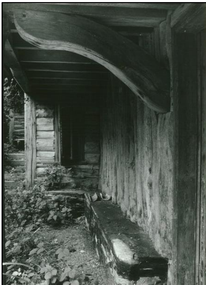
The fixed external bench during restoration
