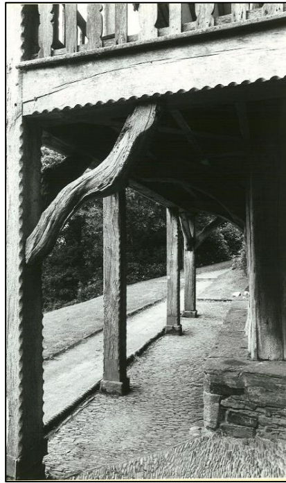
The ground floor timber supports to the veranda, and the pathway made of vertically laid pebbles.
