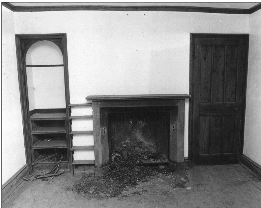
The attic bedroom before restoration
