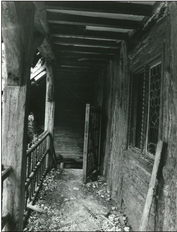
The top of the external stairs in 1977.
