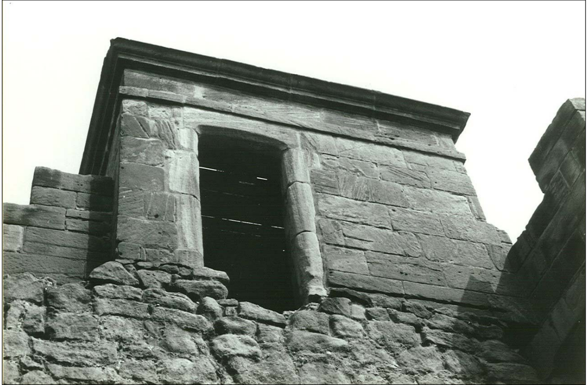
Doorway into east turret (the bathroom), in 1983.
