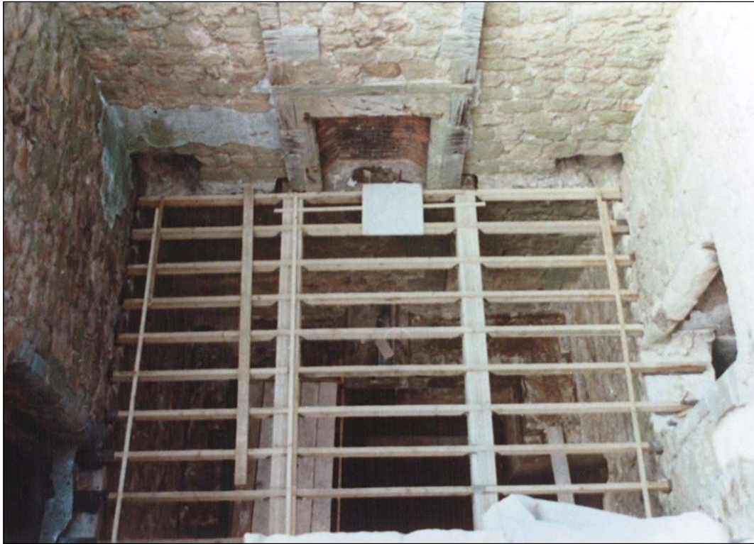
The new floor frame, resting in the old pockets.
