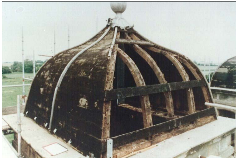
The carpentry of the turret roofs was of poor quality, and in poor condition.
