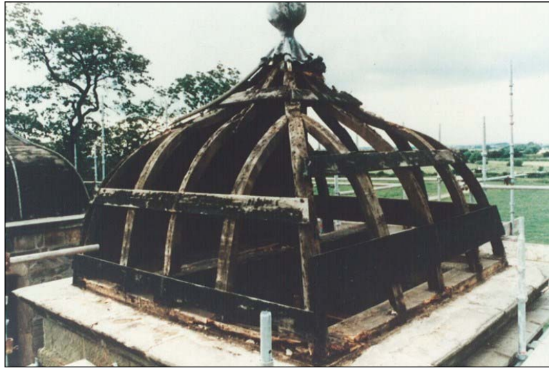
The carpentry of the turret roofs was of poor quality, and in poor condition.
