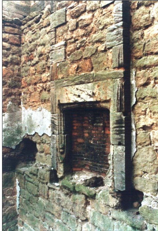
Traces of the original plaster can still be seen beside the fireplace, and in the turret (below). The joist pockets show the original floor height.
