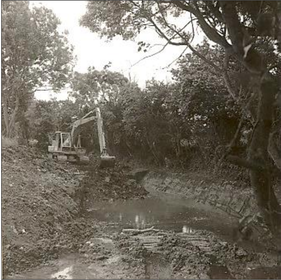
Digging the moat.
