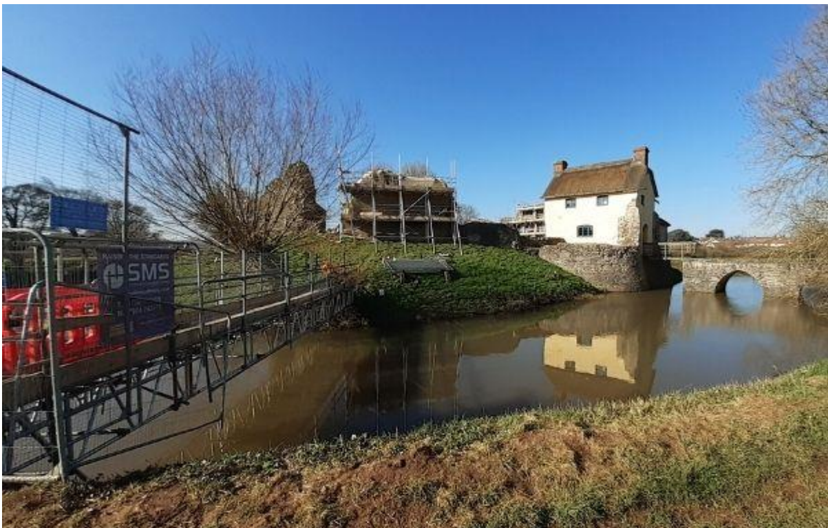
Stabilisation works underway at Stogursey in winter 2020.
