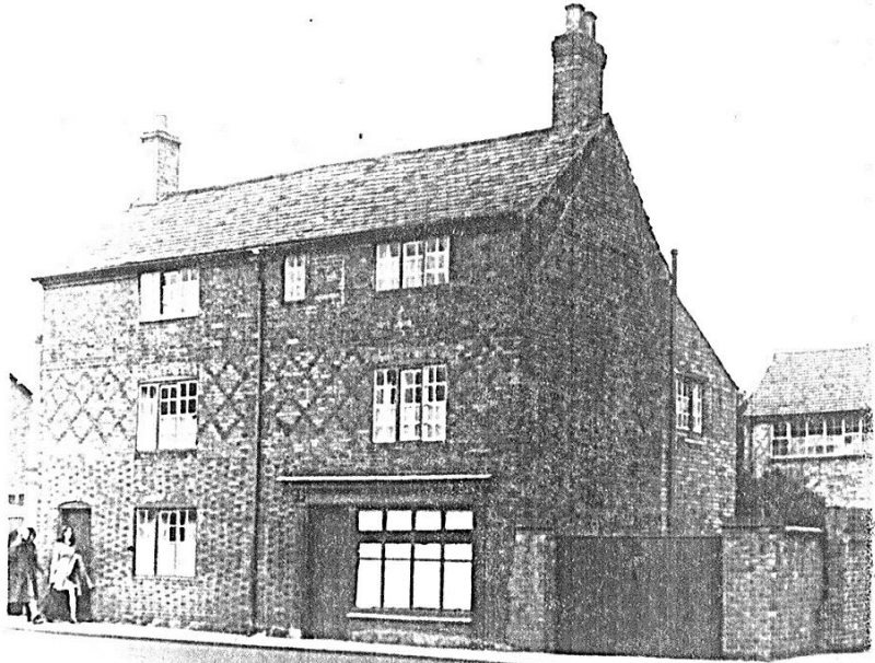
1—A FORMER KNITTERS' HOUSE AT WIGSTON, NEAR LEICESTER, SHOWING THE ALTERED BRICKWORK TO THE TOP, WHERE KNITTING WAS DONE. The frameshop behind the house was built for the knitters in the 1880s, and last used about 1914
