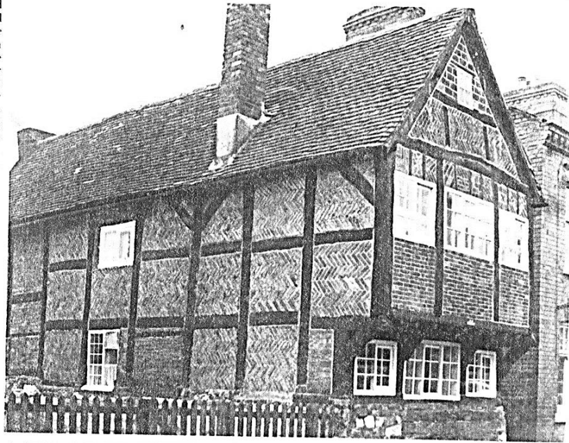
4—HOUSE AT SUTTON BONINGTON, NOTTINGHAMSHIRE. ONE OF THE OLDEST HOUSES IN THE MIDLANDS TO HAVE BEEN ADAPTED FOR FRAMEWORK KNITTING. "The brickwork on the front indicates where windows have been enlarged"
