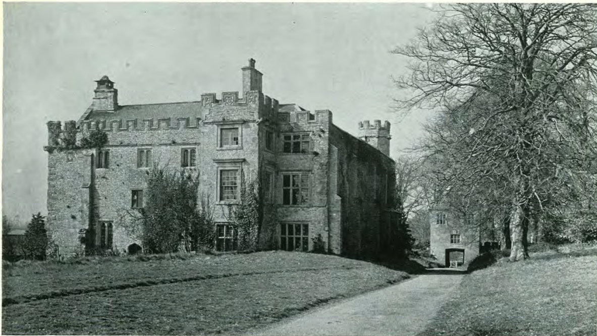
3.—THE EAST ELEVATION OF HOUSE AND GATEWAY. The portion to the left is Sir William Bonville's manor house, c. 1380; the dark buttressed side marks the position of the additions pulled down c. 1785
