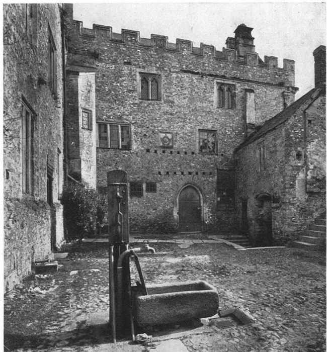
4.—THE COURTYARD, LOOKING EAST. On the right, the gatehouse abutting on to the high range containing hall and kitchen
