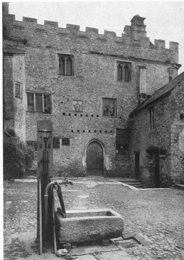
4.—THE WEST SIDE OF THE BONVILLE HOUSE OF c. 1380, FROM THE COURTYARD. The original entrance gatehouse is seen on the right
