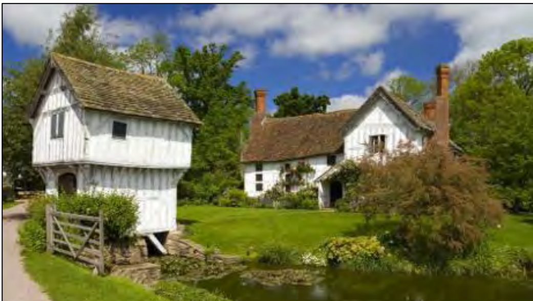
Lower Brockhampton Gatehouse, is late 15th-century. (National Trust).
