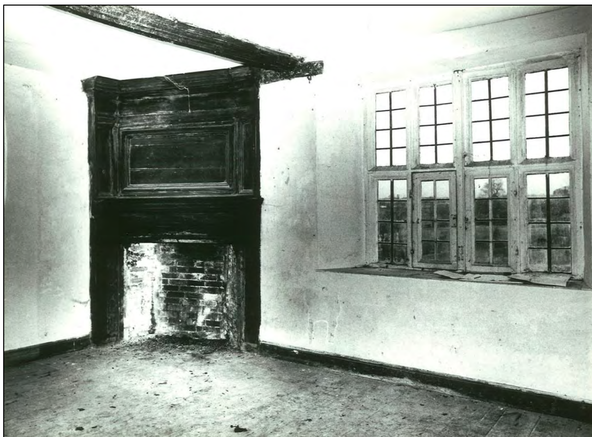
A fireplace with a late 17th-century surround and overmantel had been inserted into the first floor turret in what was then the main room. It looked as if it might have come from old Shute House, perhaps in the 1780s or in the course of the 19th century. Sadly it had become so rotten that it was beyond repair.
