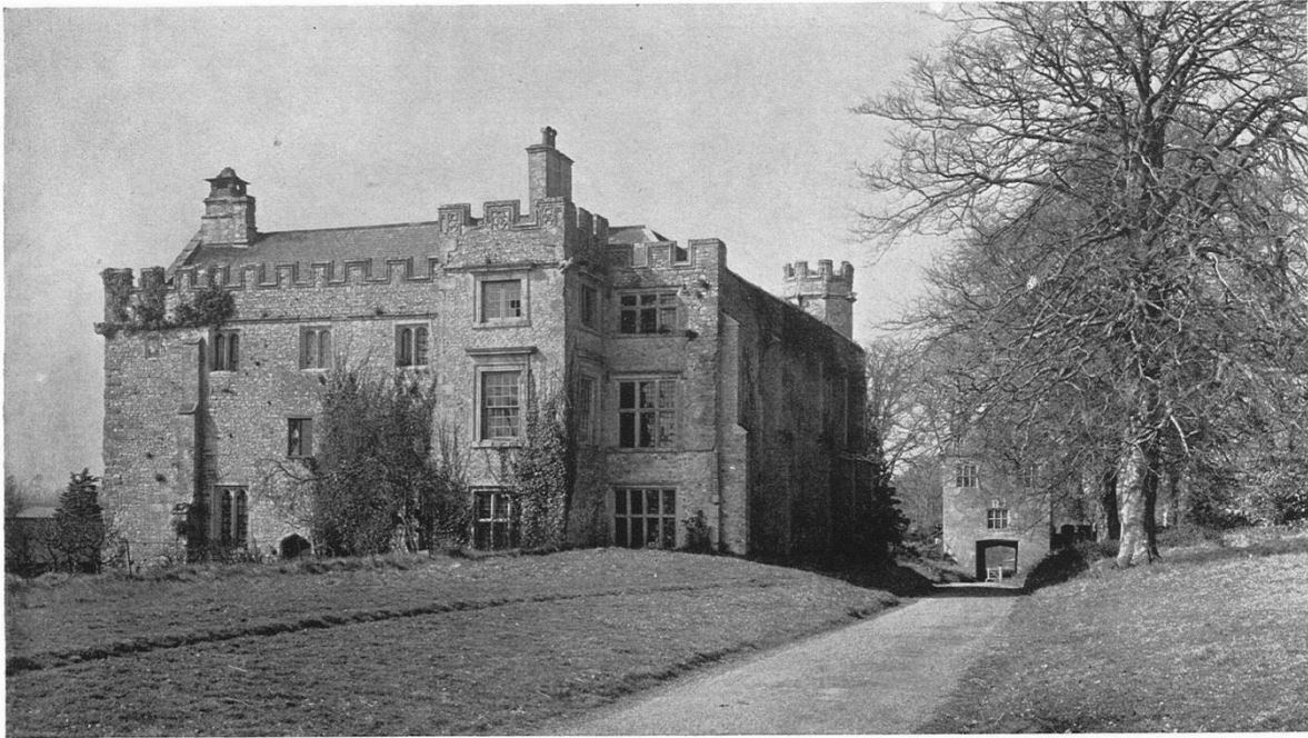
3.—THE EAST ELEVATION OF HOUSE AND GATEWAY. The portion to the left is Sir William Bonville's manor house, c. 1380; the dark buttressed side marks the position of the additions pulled down c. 1785
