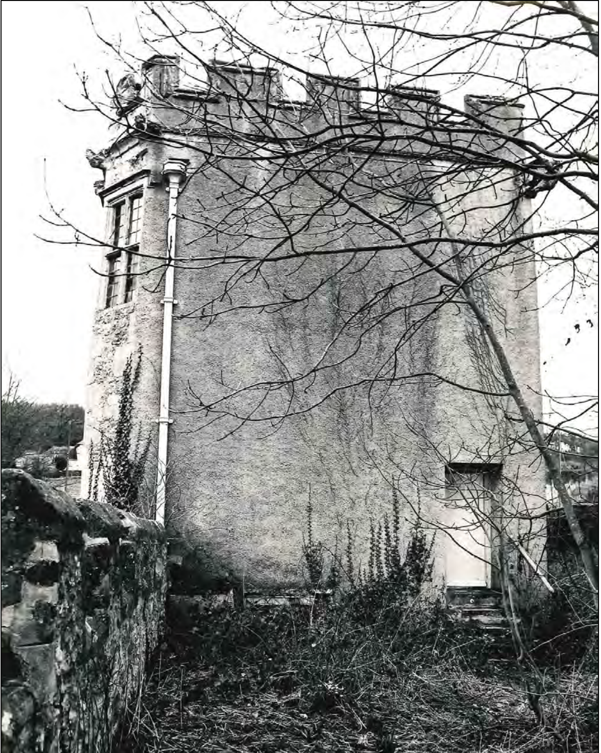
The door on the right was turned into a window by Landmark in 1980.
