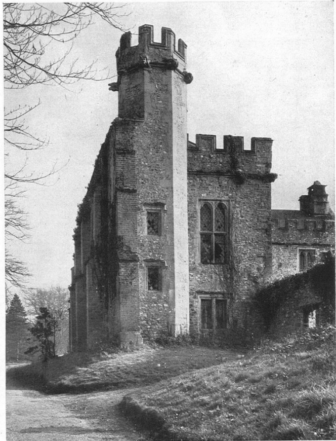
9.—A STAIRCASE TURRET AND THE WEST END OF THE NORTH RANGE. Early 16th-century. The buttresses c. 1785
