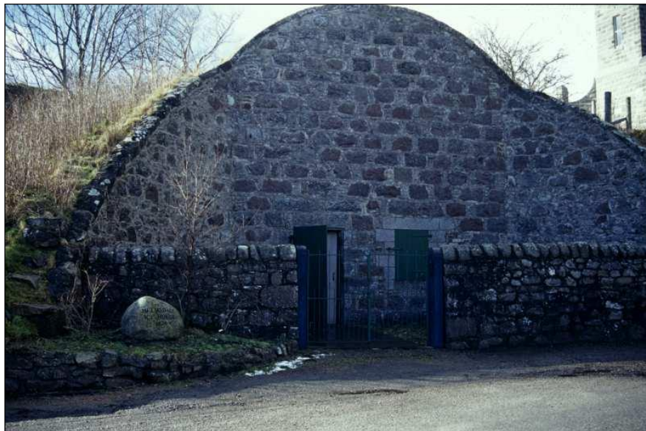
The Berriedale icehouse (its interior of well-dressed stone with carefully laid pebble floor, as shown above) is typical of many built in Caithness in the 19 th century. The example below is in Helmsdale, built in 1824. While larger, it is not dissimilar in form. Ice would be harvested in winter from the lochs inland.
