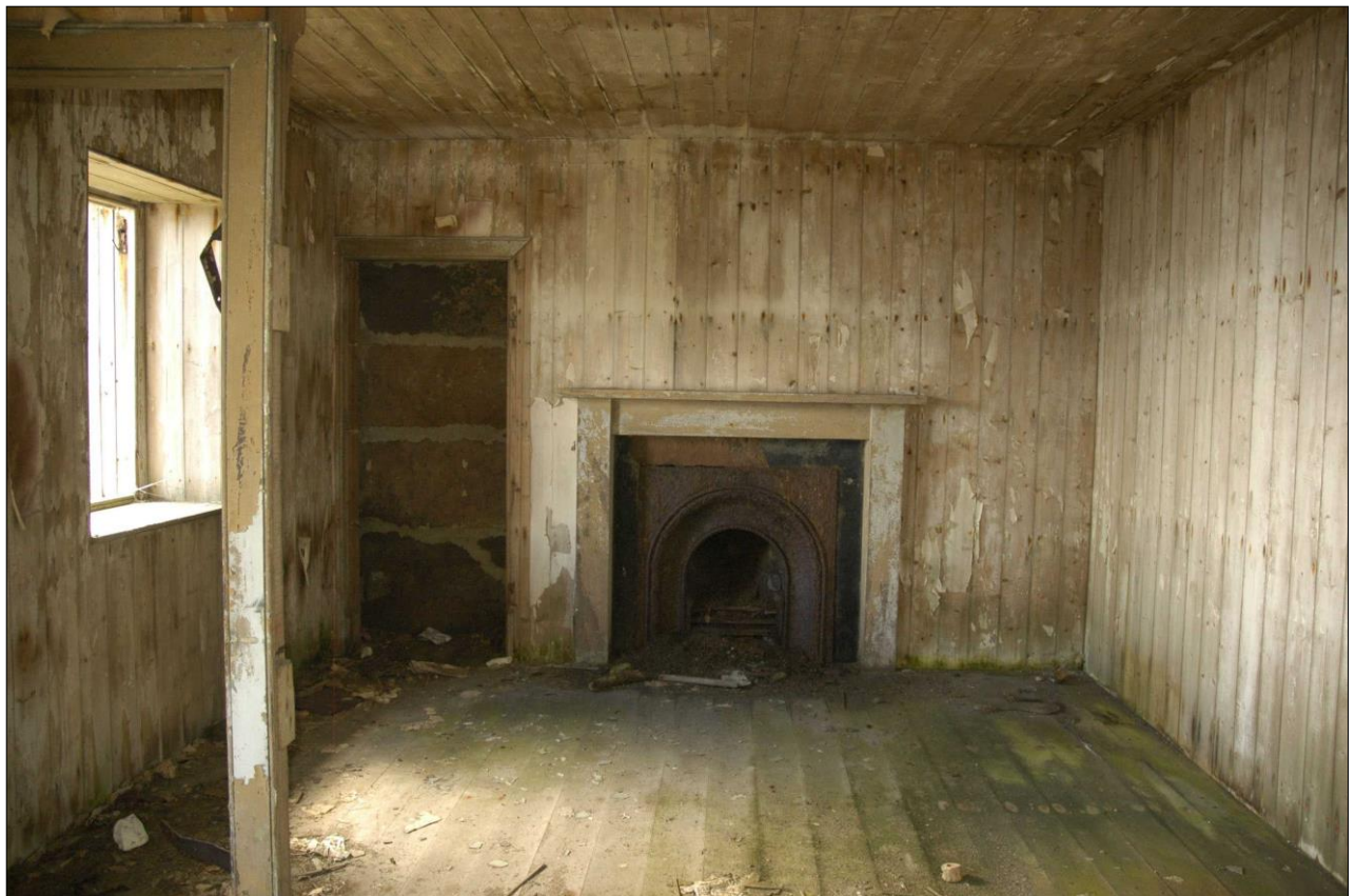
Interiors before restoration. Note the wooden partitions between the two principal rooms (top), and the matchboard wall lining put up in the 1884.
