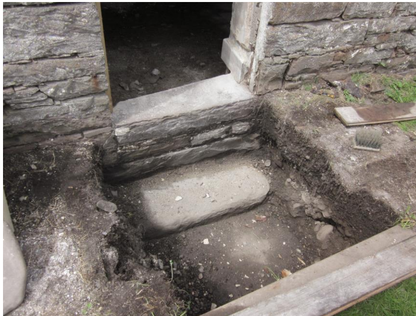
An original step to the front door and the raising of the threshold.
