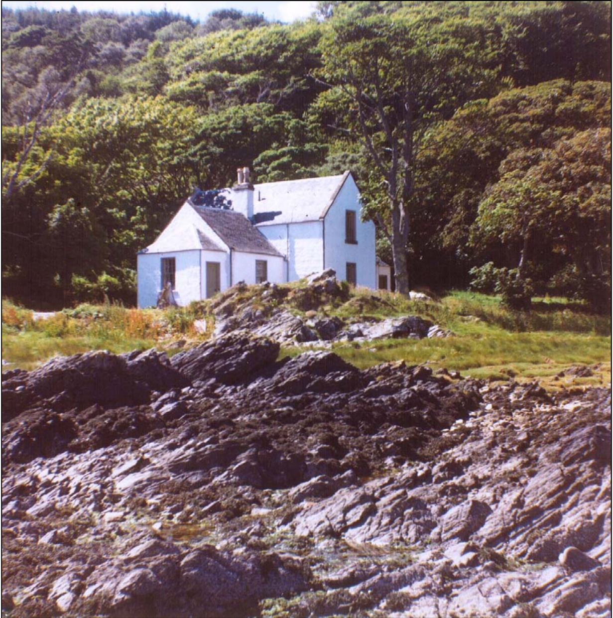
Shore Cottage after restoration.
