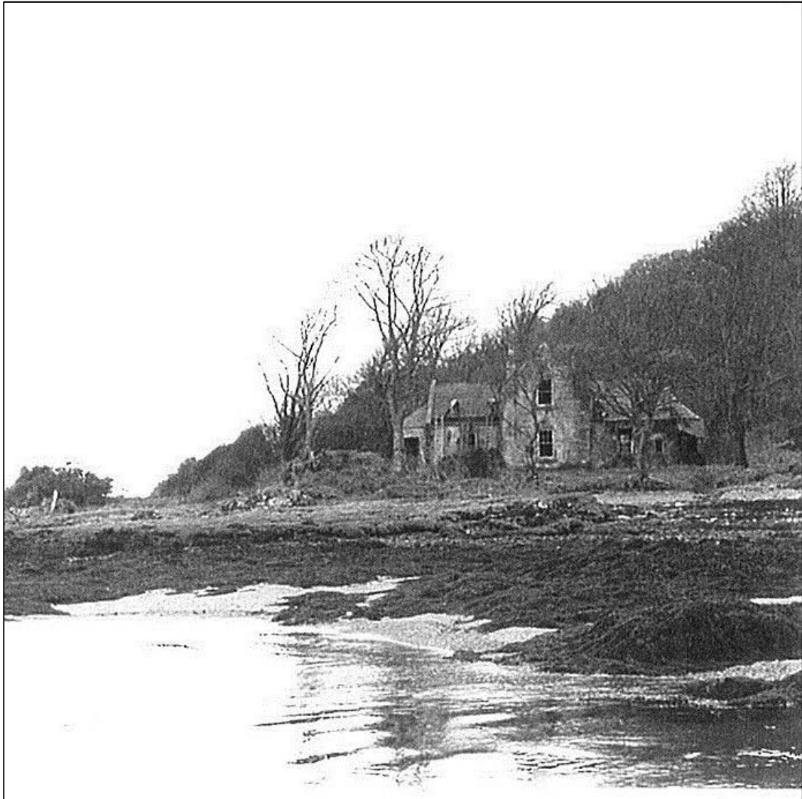
Shore Cottage before restoration
