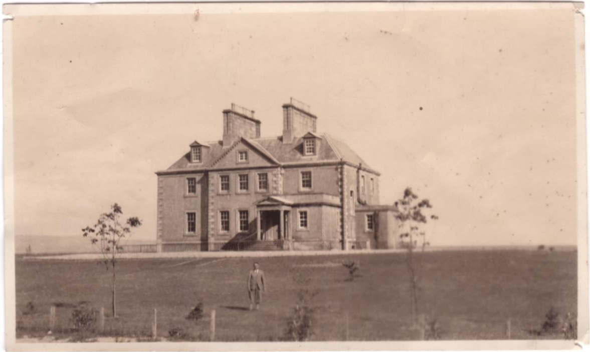
Saddell House shortly after its acquisition by the Moretons, with signs of their new planting apparent.
