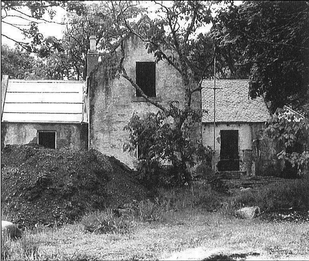
The north east side, work in progress
