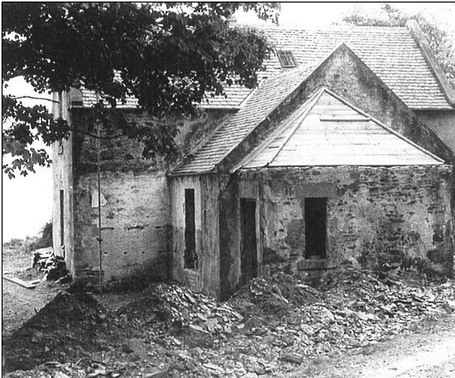
Work in progress round the front door.
