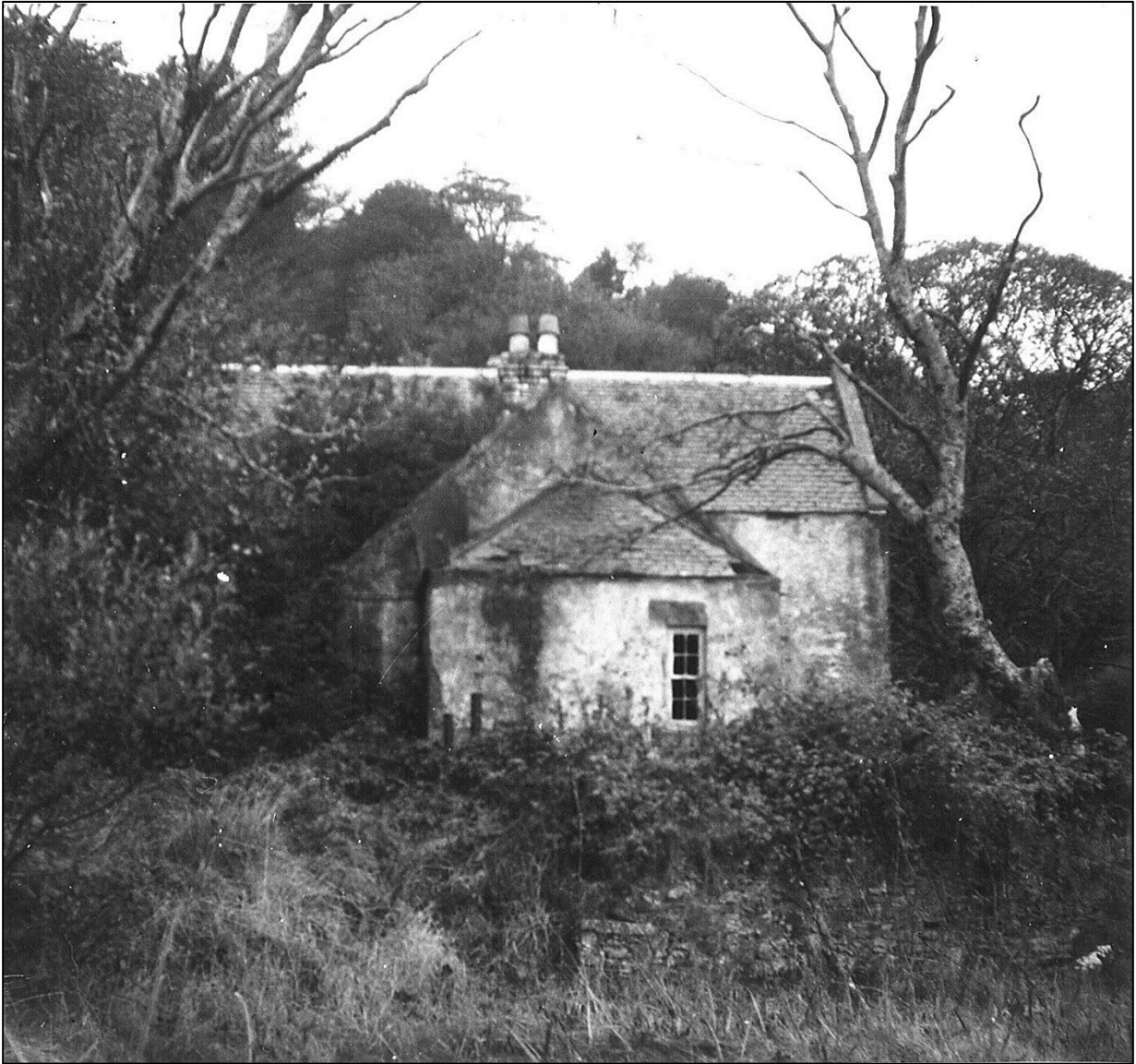
The south east side before restoration. The sitting room chimney, seen here, was harled with the rest of the house.
