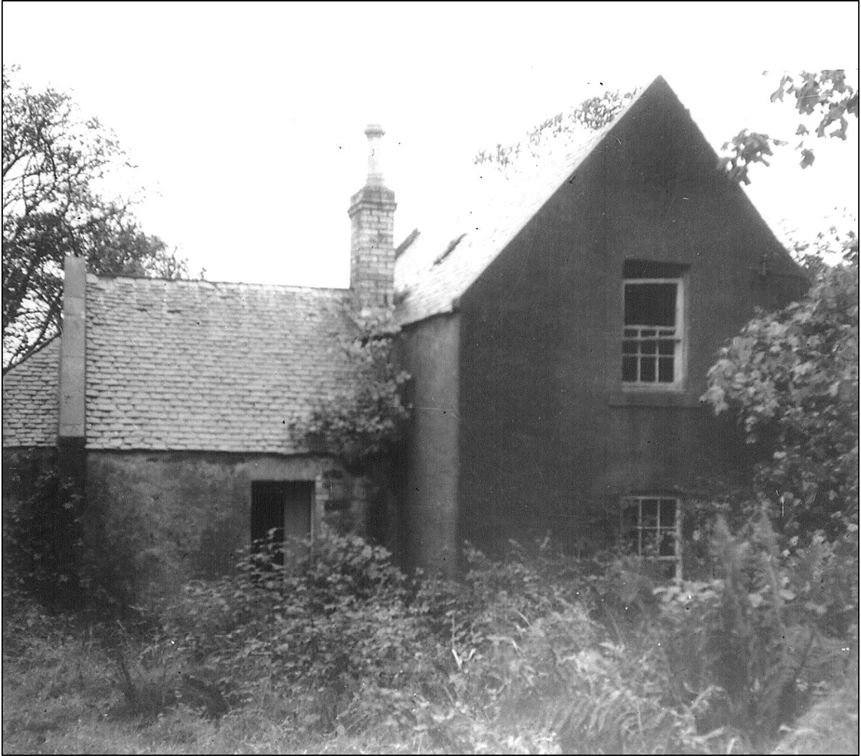
The south west side. Windows were repaired or re-made to match.
