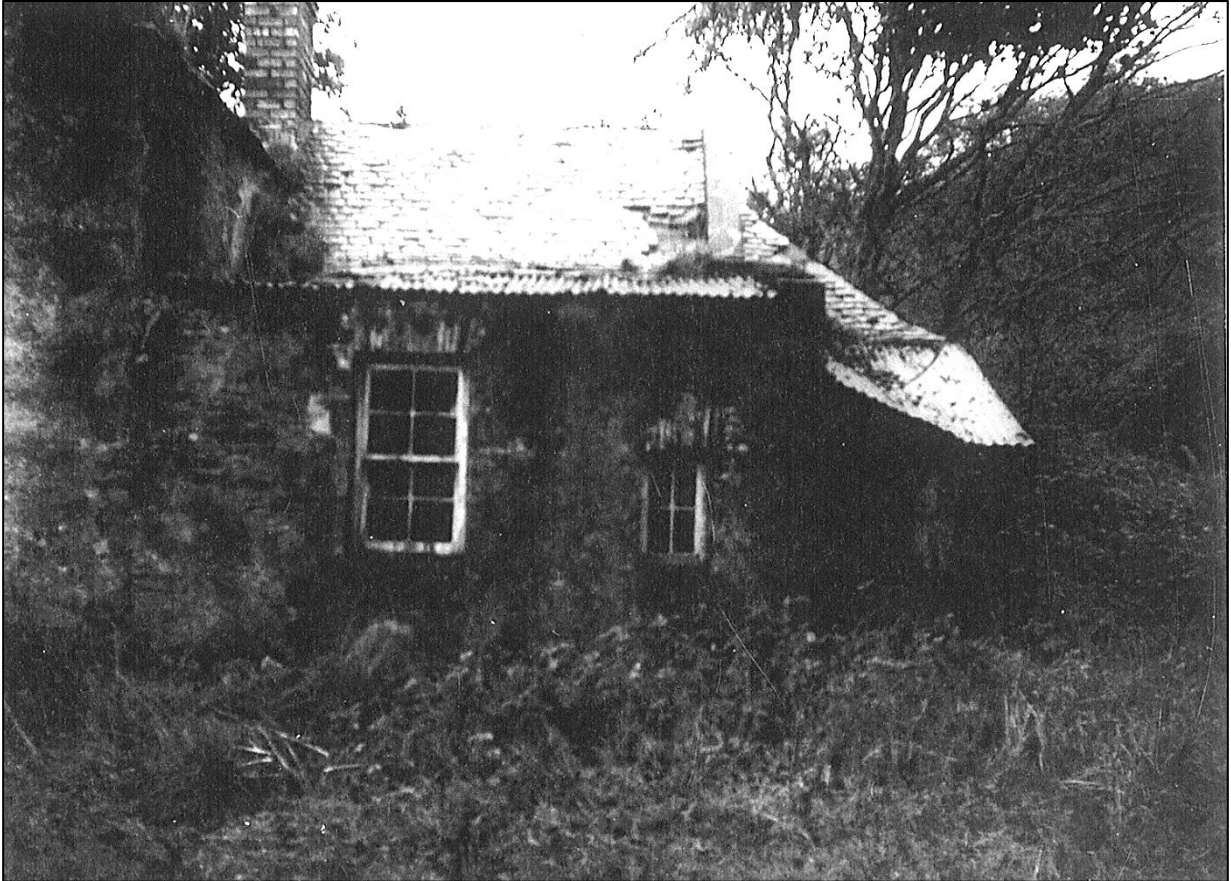
The kitchen chimney, seen here, was no longer needed and was removed.
