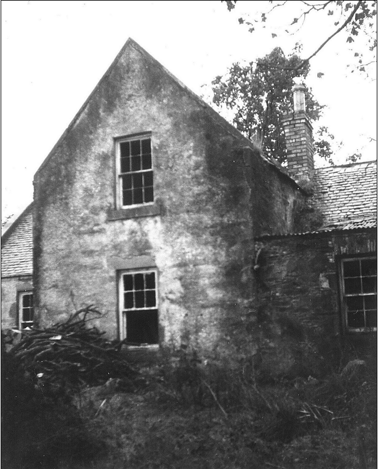
The north east side before restoration.
