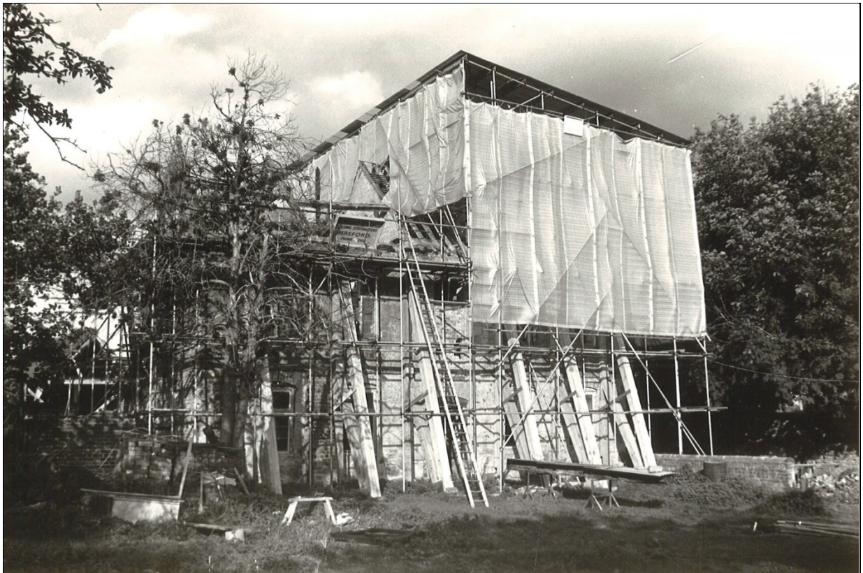
Shelwick Court with temporary shoring in 1982
