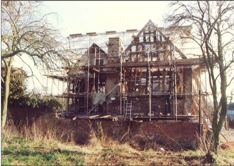
The medieval wing was protected by a temporary roof while work was carried out
