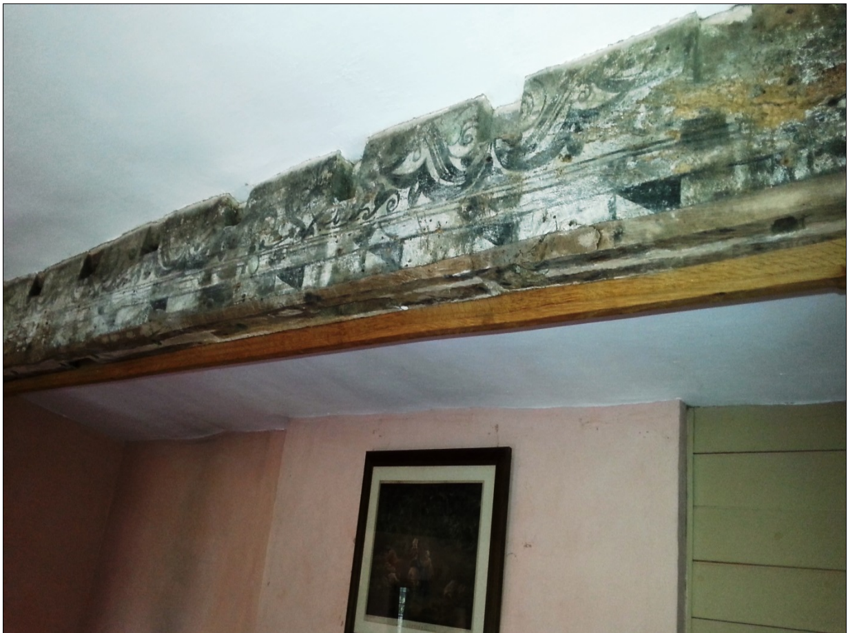
Exposed 16 th C beam
