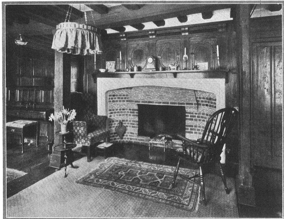
This picture shows the original stone fireplace, discovered behind a Victorian grate, and now restored, with red Tudor bricks and a red-tiled hearth.
