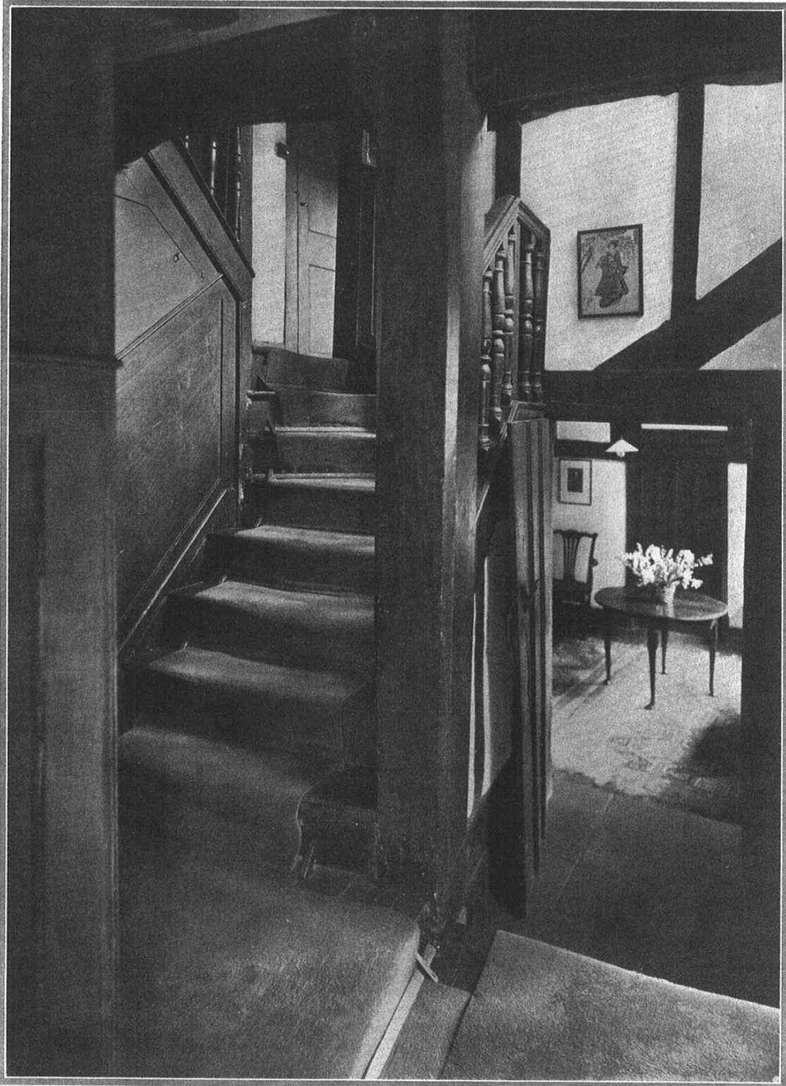
Seen from the hall. Note the turned balusters and slab doors.
