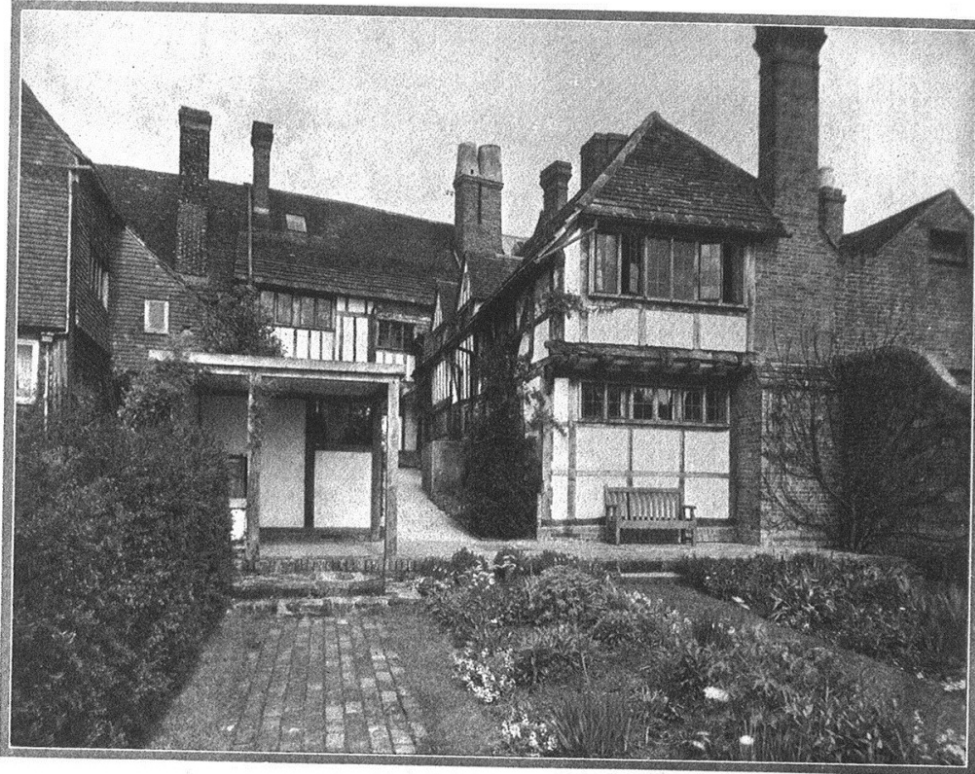
The south wing has been added to, but in keeping with the rest of the house. The Horsham stone of the roof merges into weathered Sussex tiles above. The little garden shelter is open to the south.
