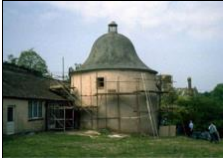
The Dovecote during recent repairs
