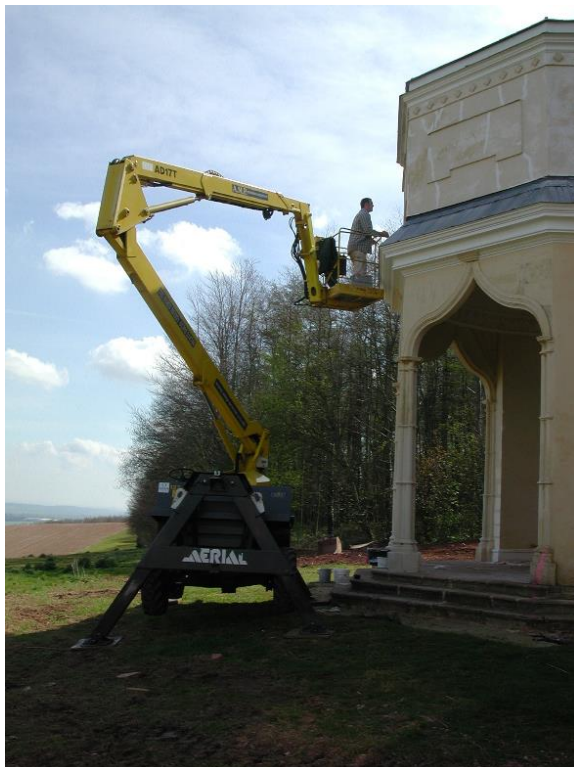
Inspecting the flashing above the umbrello.
