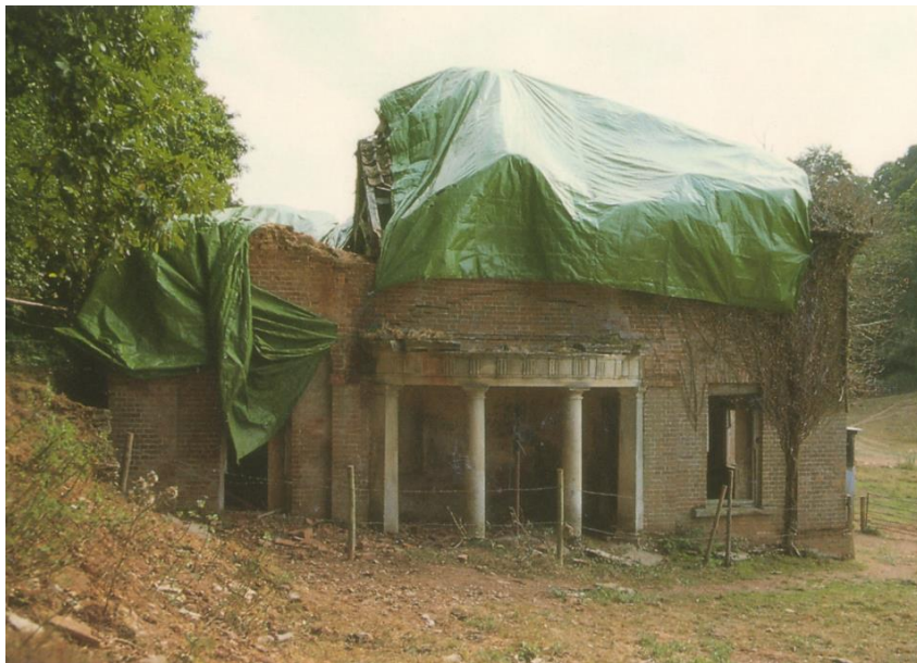
The Temple of Pan before restoration as a private house.
