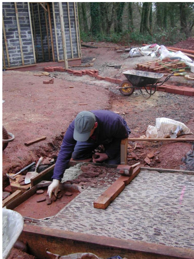
Labour intensive: sanding the coccio pesto floor (above) and bedding pebbles outside.
