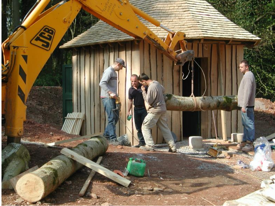
Positioning the ash trunks (from the woodland behind) which support the bathroom eaves. They stand on stone bases to prevent rot.
