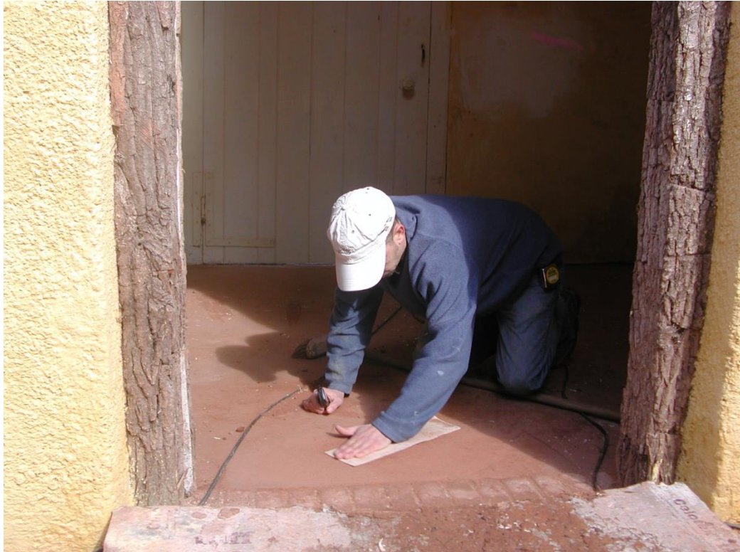
Labour intensive: sanding the coccio pesto floor (above) and bedding pebbles outside.
