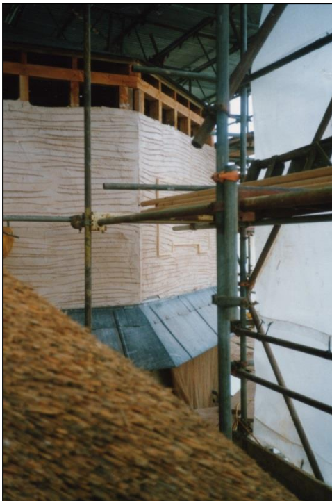
Left: Scratch coat of render and lead flashing. Right: The fragment of plaster work on which the frieze restoration was based.
