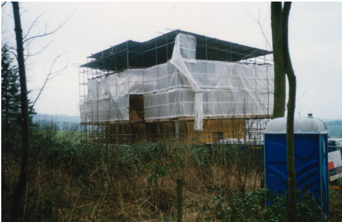
During repair by the SBPT.
