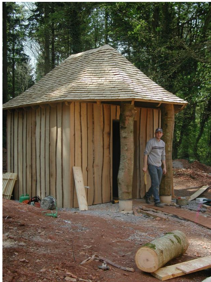
Positioning the ash trunks (from the woodland behind) which support the bathroom eaves. They stand on stone bases to prevent rot.
