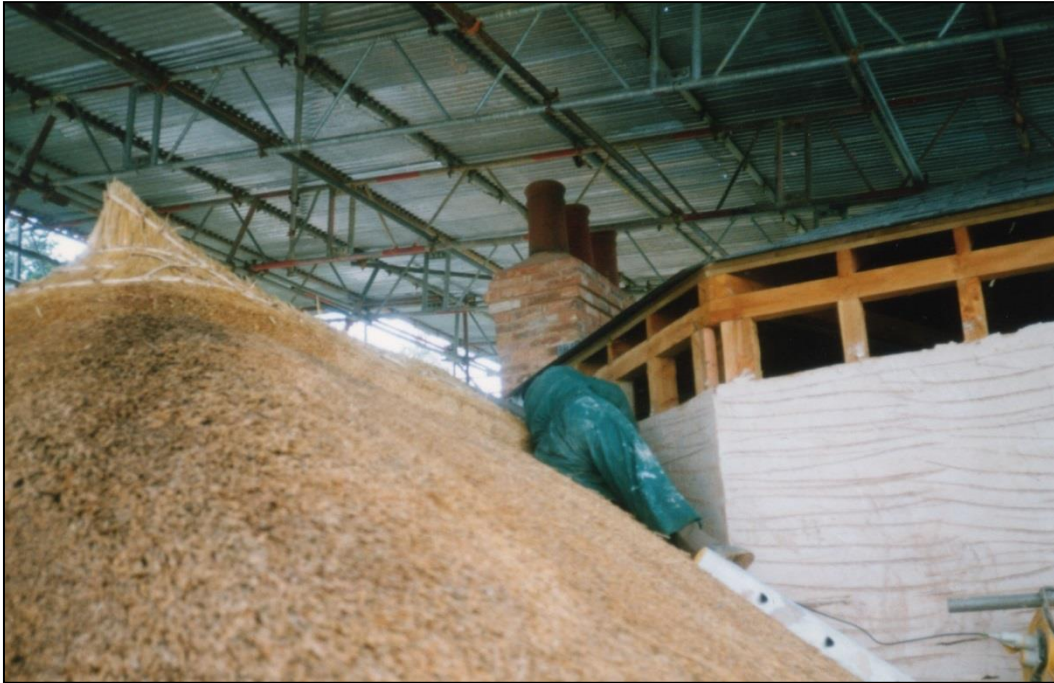
Rebuilding the roof above the umbrella.
