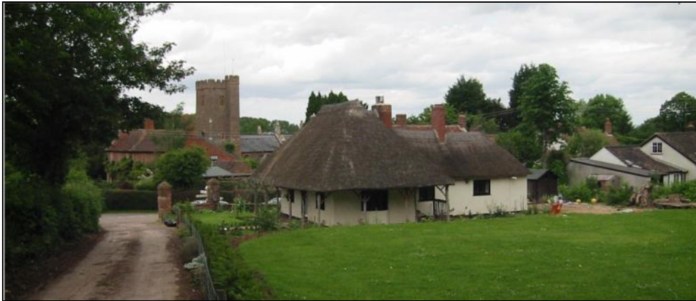
The gate lodge to Halswell House, with St Edward's Church beyond.
