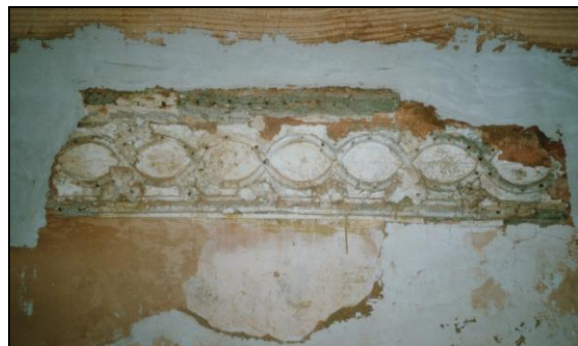
Left: Scratch coat of render and lead flashing. Right: The fragment of plaster work on which the frieze restoration was based.
