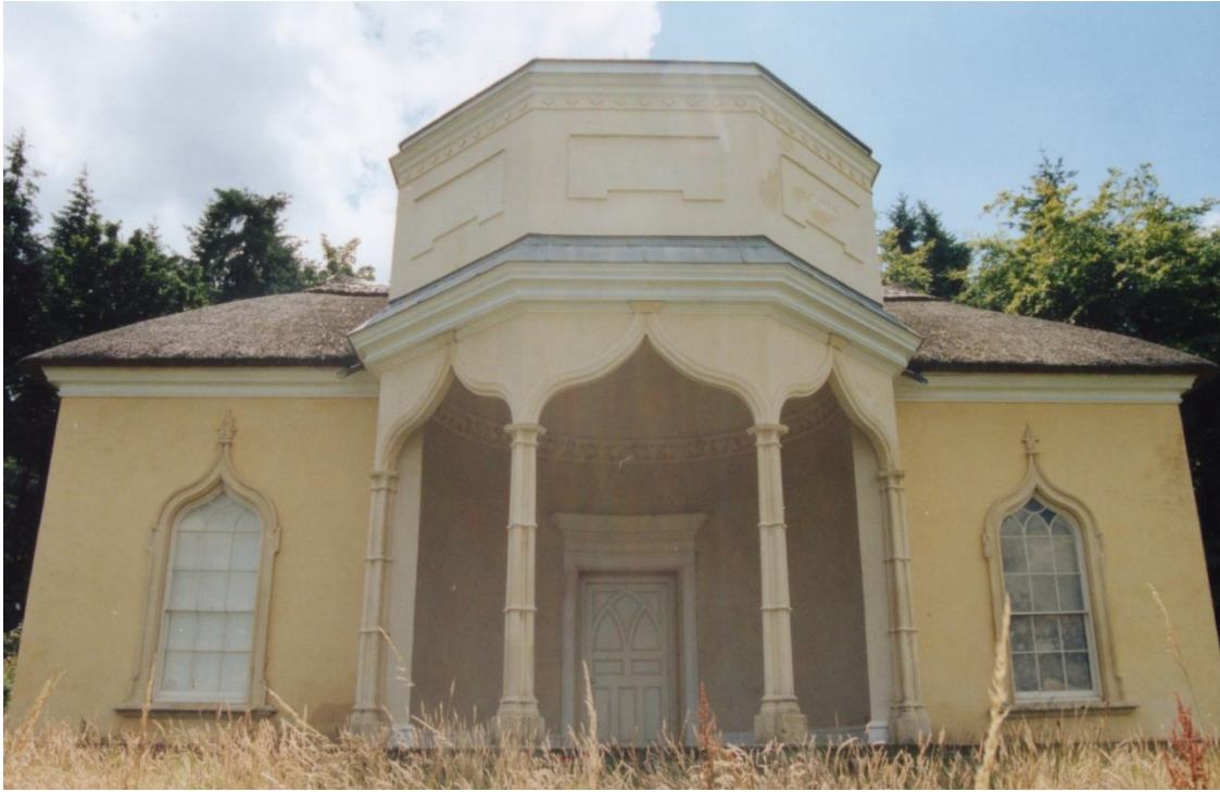
Robin Hood's Hut in 1998 after restoration by the Somerset Building Preservation Trust.
