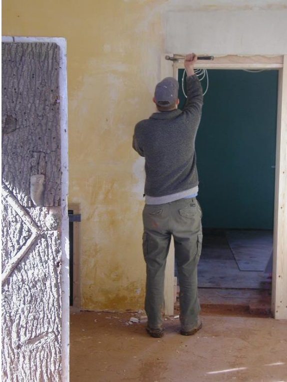
Finishing off the new door to the bedroom
