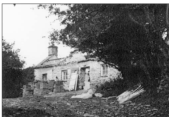
Ty Coch – work underway
