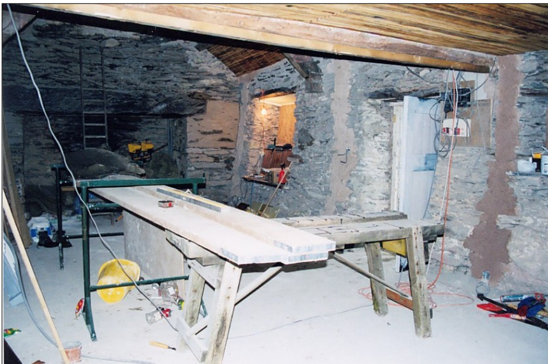
The croglofft extension removed, deep grouting and re-pointing underway.
