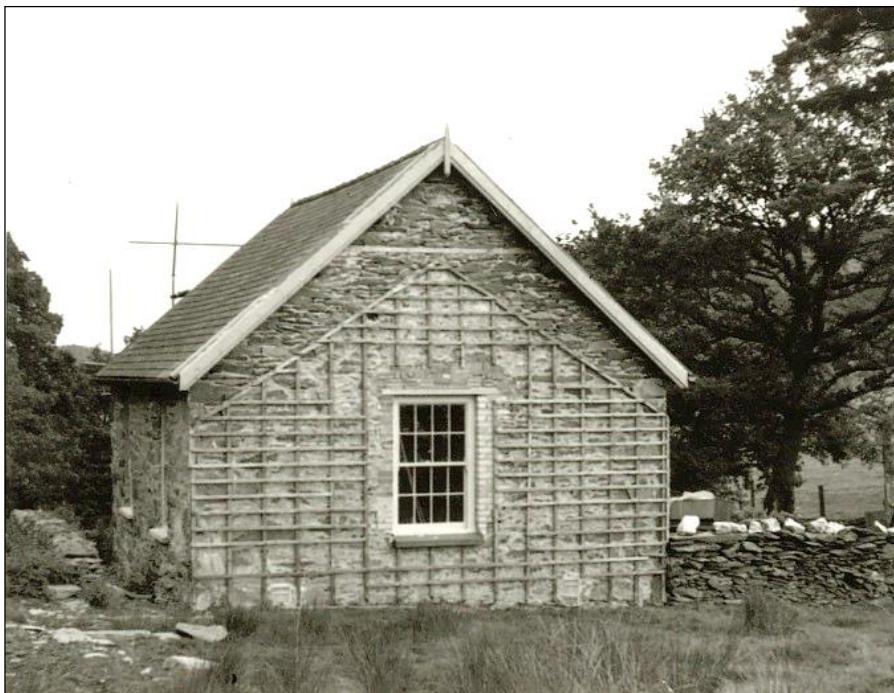
Under restoration, with the new window installed
