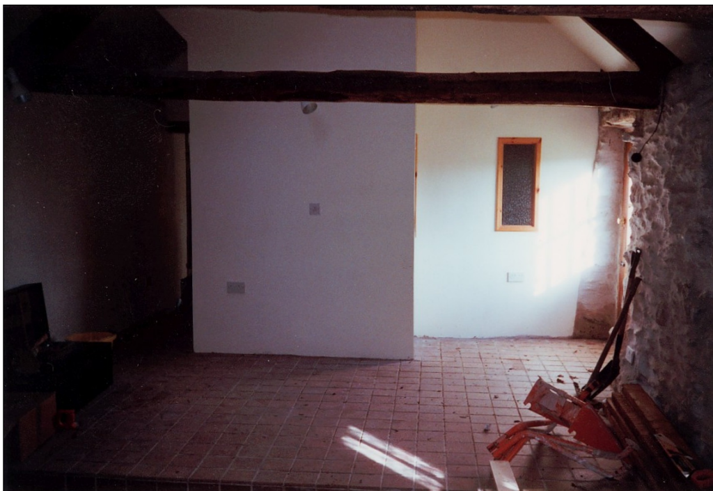
Looking into the byre from the cottage before work began, at what is now the bathroom and lobby.
