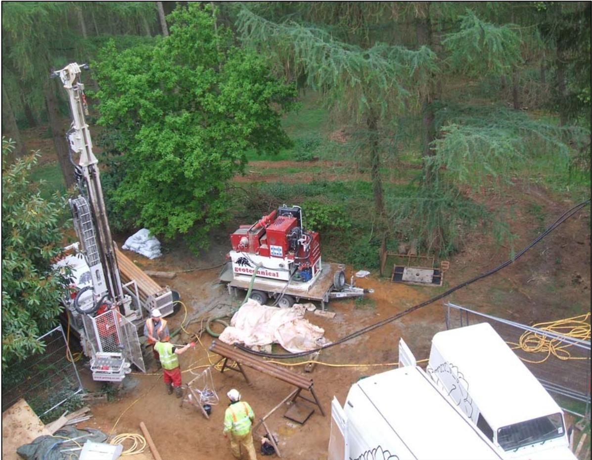
**Drilling one of the boreholes for the ground source heat system.**
