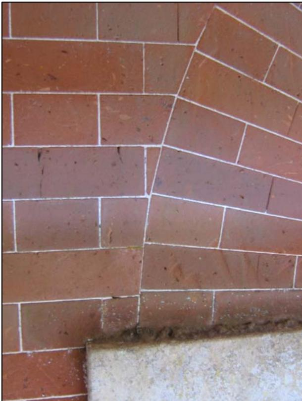
**The exceptional quality of the brickwork is striking, with joints only a millimetre or two wide. Note how carefully the triangular slip has been pieced in to complete the curve; also the grooves for the (then missing) *faux* pointing to maintain the rhythm.**
