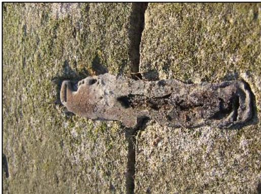
The NE turret coping stones uniquely showed cracking and discolouration, indicating fire damage in this area. One of the leads clamps holding the coping stones in place is dated 1865, perhaps the date of the fire. Note too the masons' marks for setting out.
