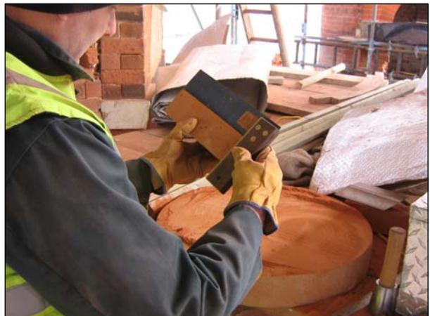
Other bricks, like those being laid out for a turret arch by Emma Simpson above, were cut and rubbed on site. The soft bricks cut easily. They were individually rubbed to shape and then carefully measured
