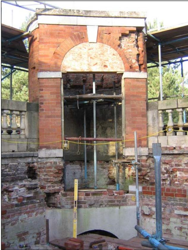
The remnants of the roof removed, this precarious turret illustrated the complexity of the task. All four turrets needed their fronts dismantling and rebuilding.
