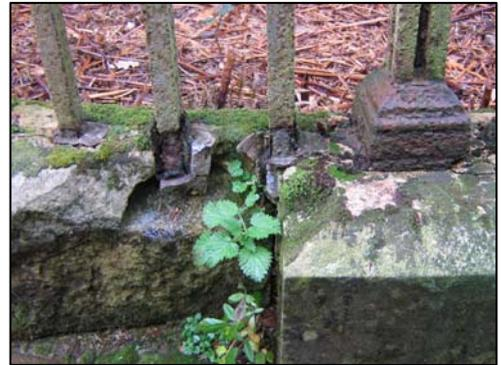
**The railings before repair. Where the lead plugs at their base had failed (above), the iron railings had corroded and fractured the stone plinth. Some uprights were missing altogether, others had lost their tips.**
