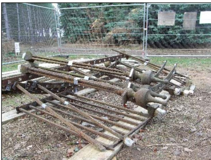
**In the end, most of the railings had to be cut to free them from the stone plinth. They were each numbered before being taken back to the forge for repair.**
