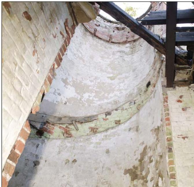
The main chamber was open to the sky through decaying rafters. The staircase timbers had collapsed into a pile in the basement, leaving only a paint scar and bearer sockets to show where it had formerly been.
