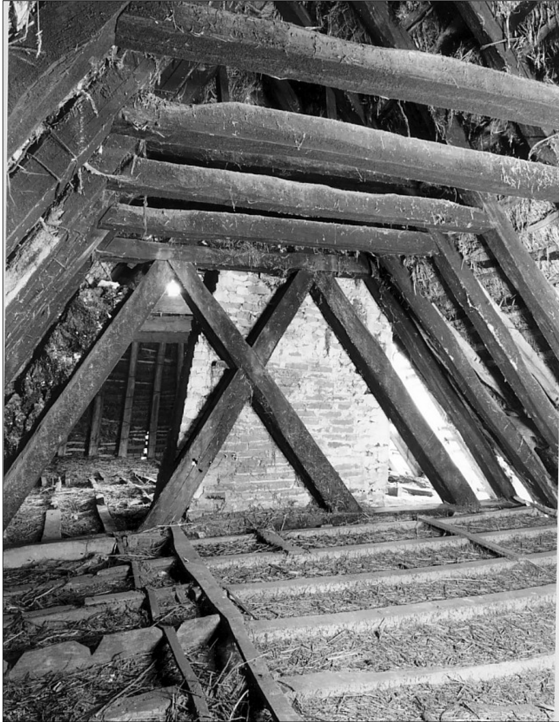
View of the roof to the south after removal of stack.
