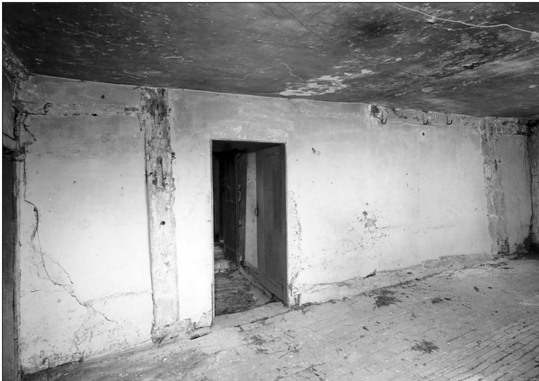
Ground floor room at the North end, looking south.
