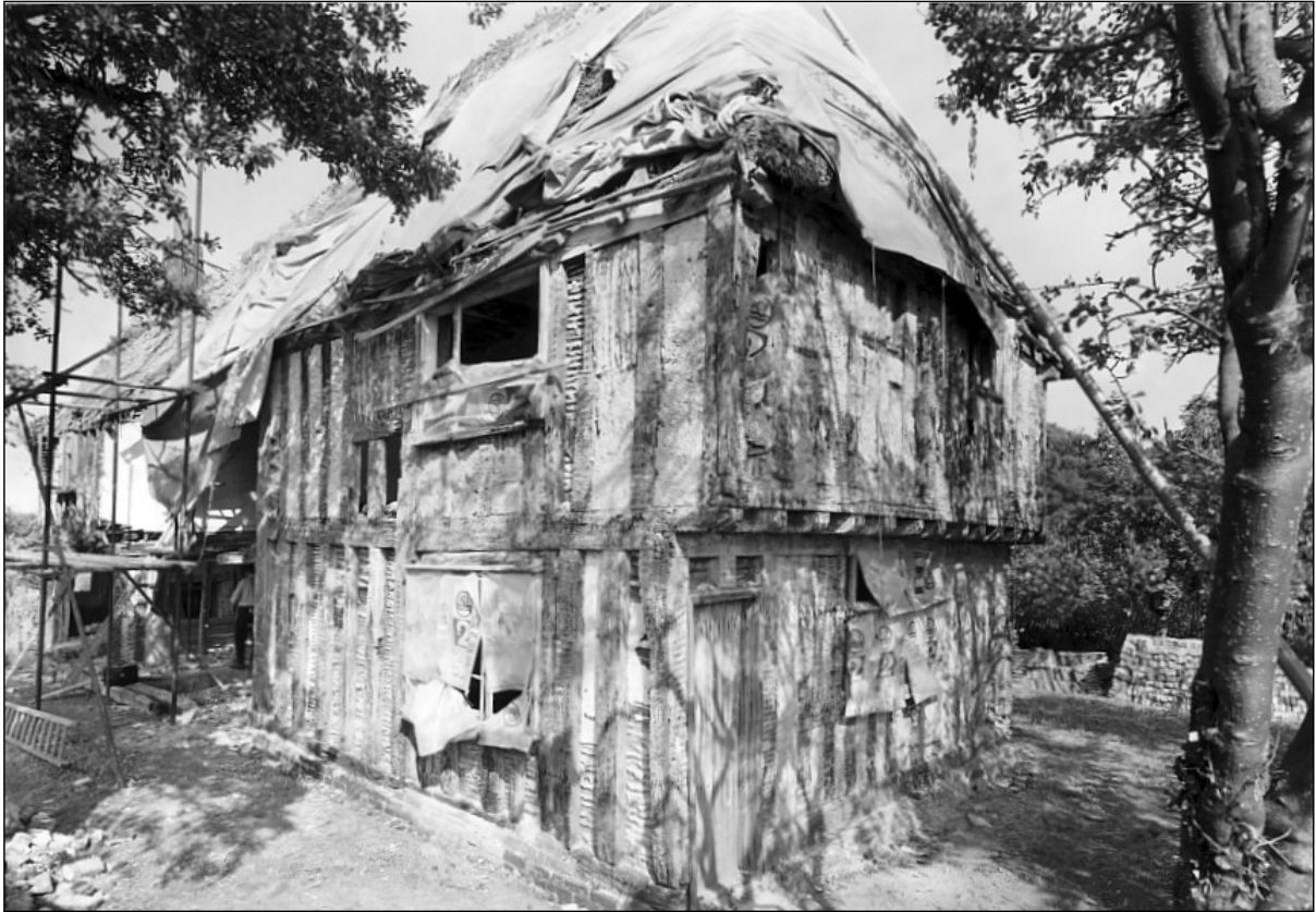
The exterior plaster removed, September 1970.
