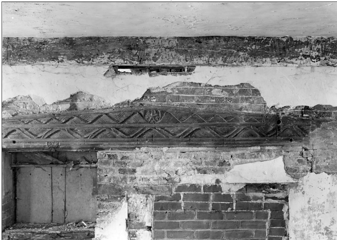
The very decorative fireplace lintel was discovered when plaster was stripped away and has been left in situ.
