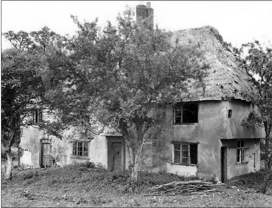
Purton Green in 1965, before restoration.
