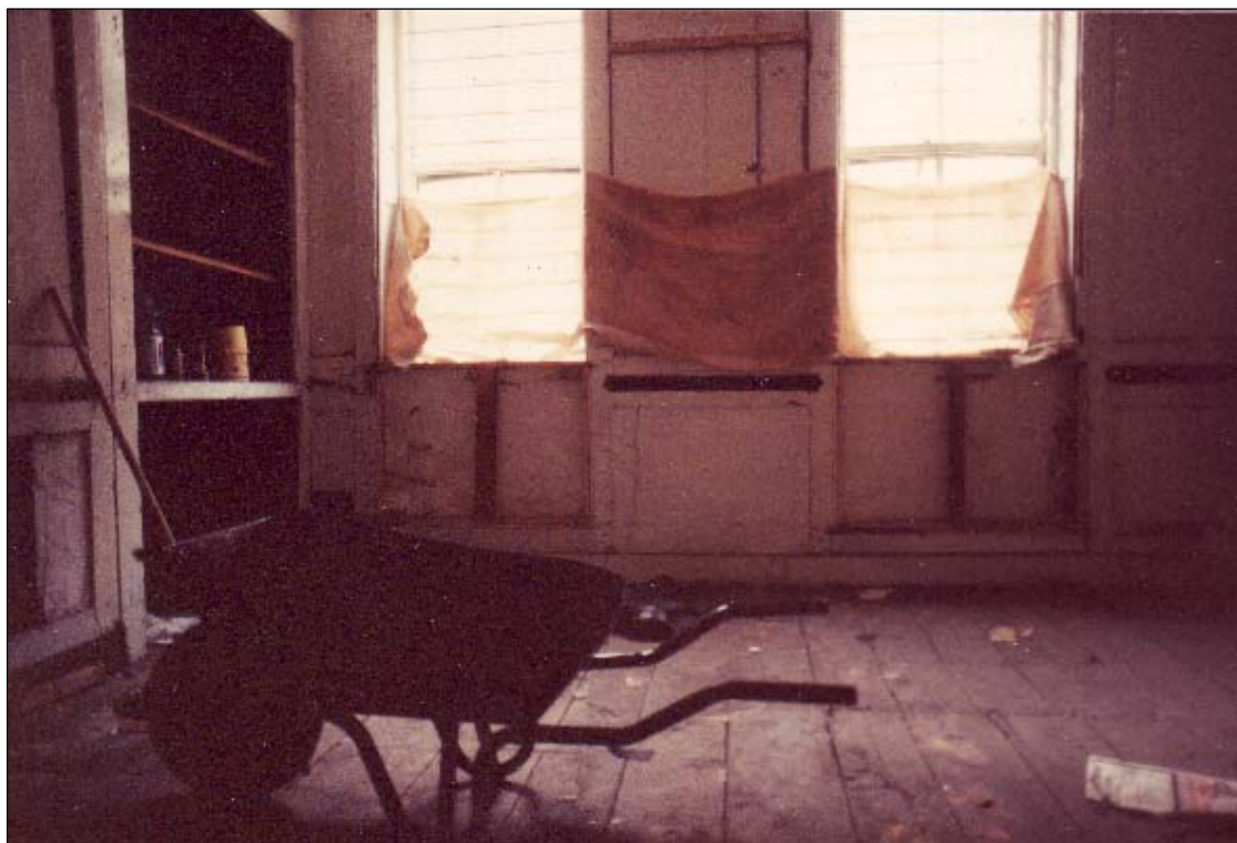
Ground floor, front room before restoration.
