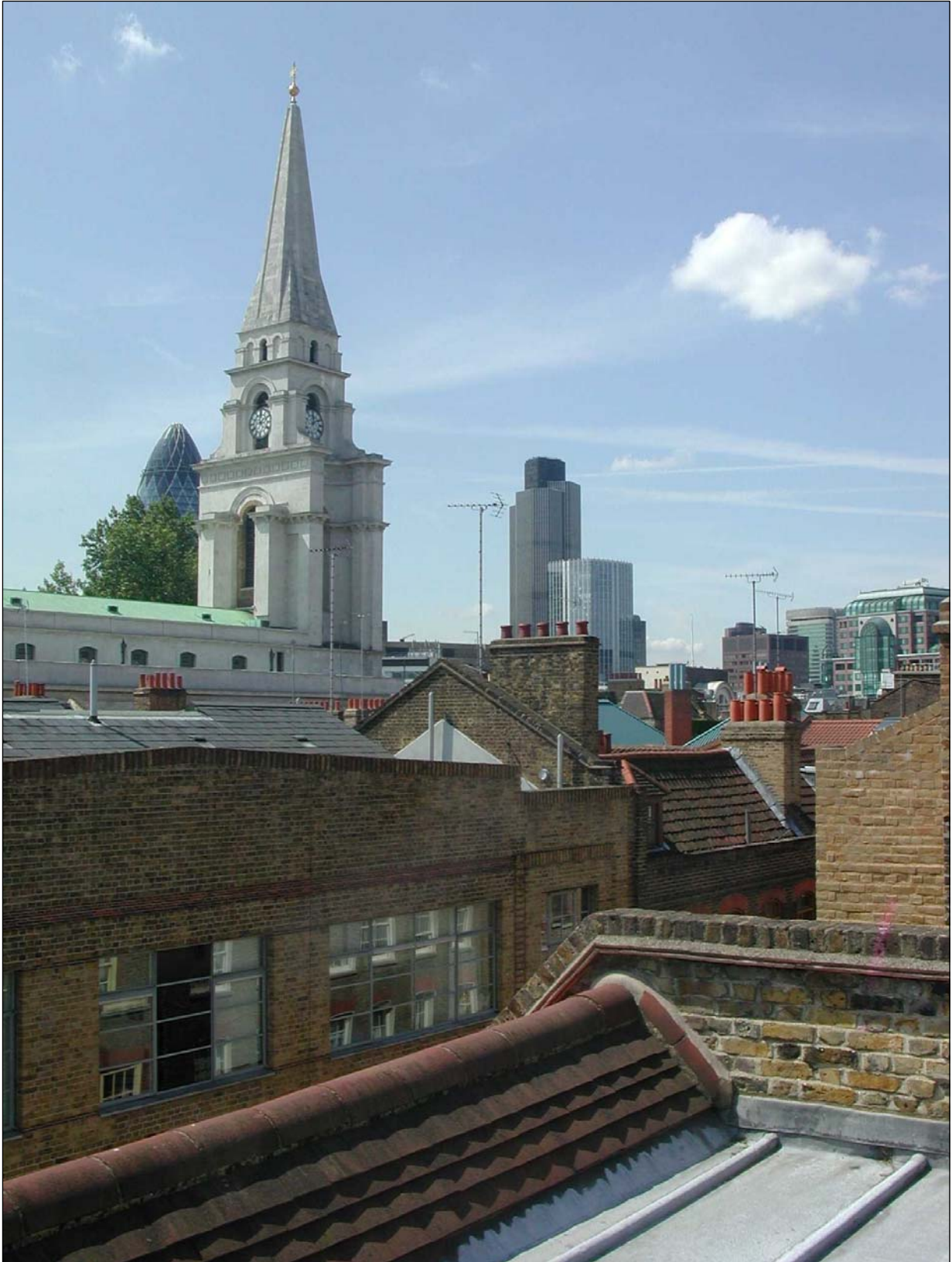
View from the roof of No. 13 Princelet Street
