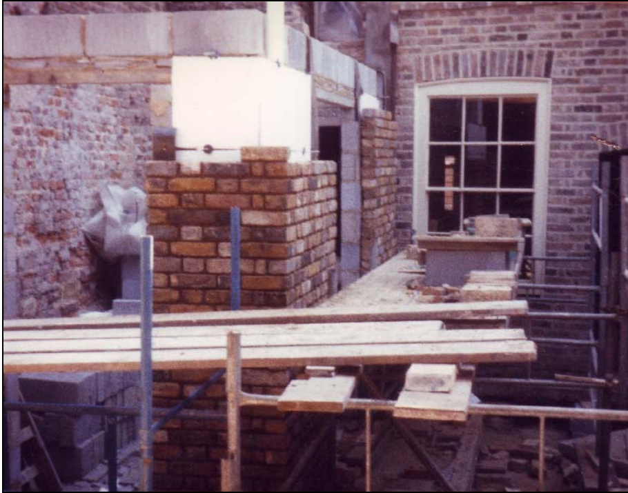
The new extension under construction, the rear elevation having been rebuilt.
