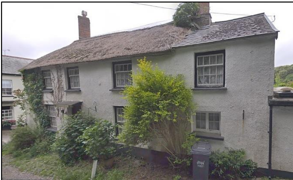
Georgeham: Millie's Cottage (? Church-house)
