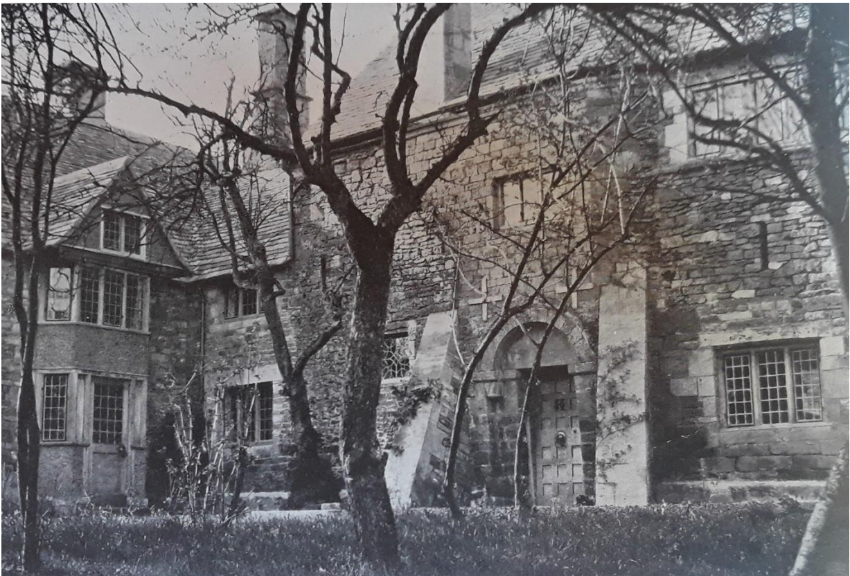
The Norman Chapel in Chipping Campden, also repaired by Ashbee, was given the same irregular buttresses as the Priest's House.
