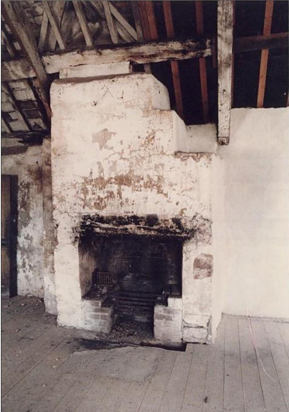
The first floor in 1983. Such integral fireplaces are a distinctive feature of church houses as civic buildings, at a time before they were still relatively rare in domestic dwellings. However, this one has probably been inserted at a later date.
