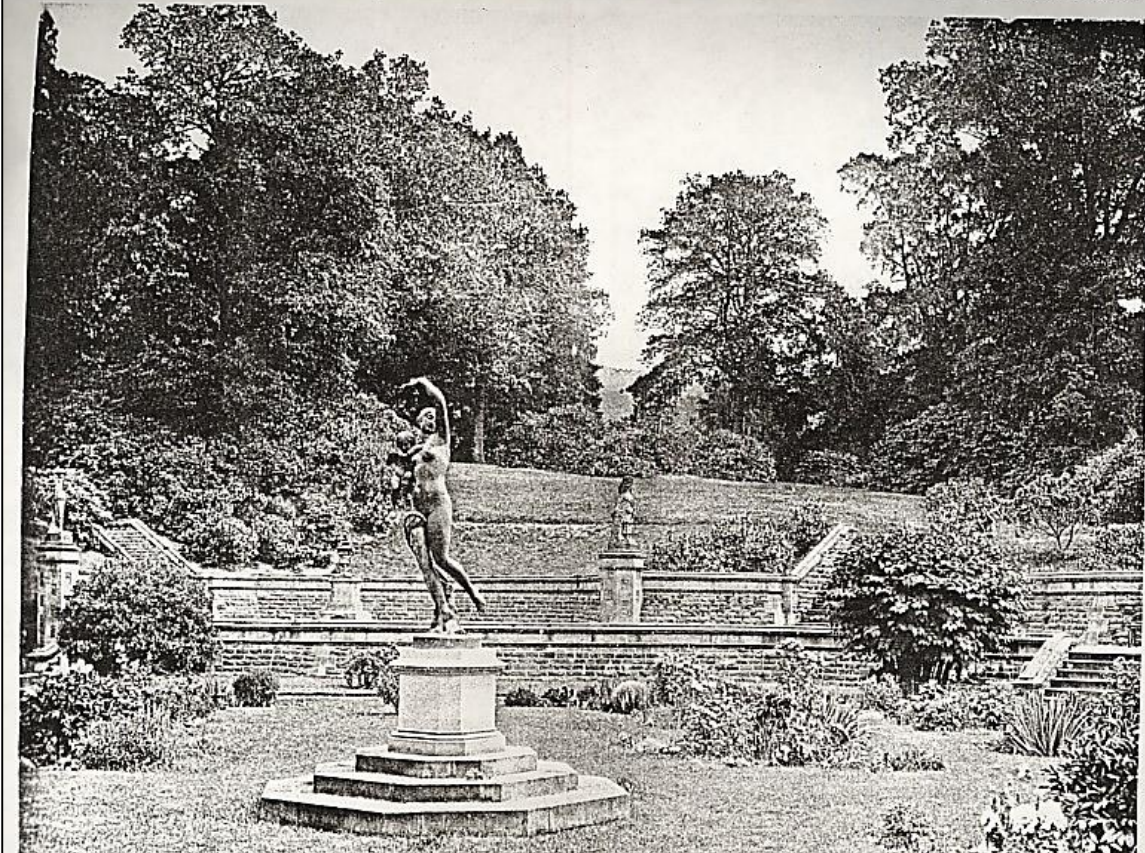
The south east terrace
