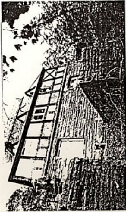
The ornate upper station showing the buttresses where the funicular cars stopped and the opening in the wall for the winding cable (J. Horsley Denton).
