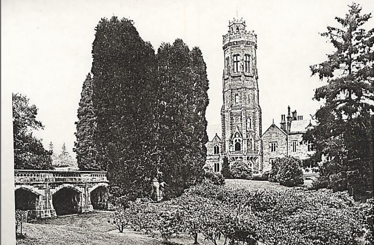
Bridge on the South East
