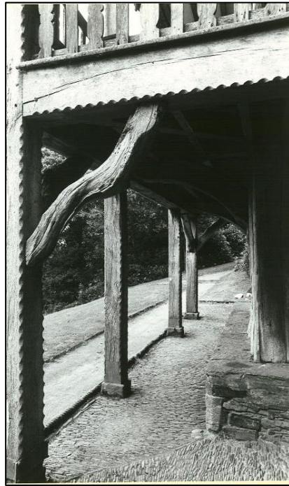
The ground floor timber supports to the veranda, and the pathway made of vertically laid pebbles.
