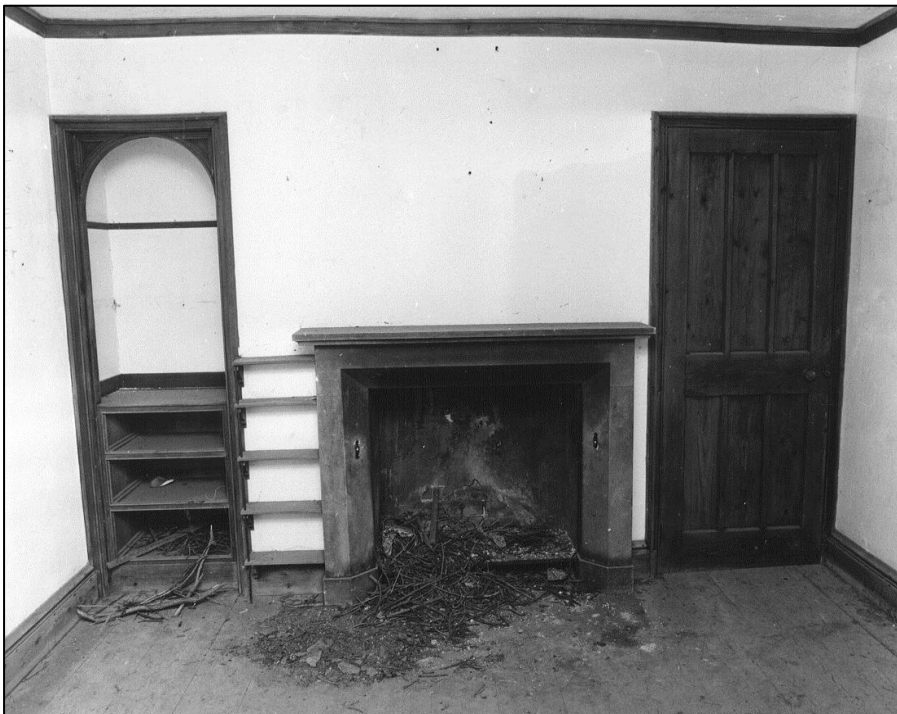
The attic bedroom before restoration
