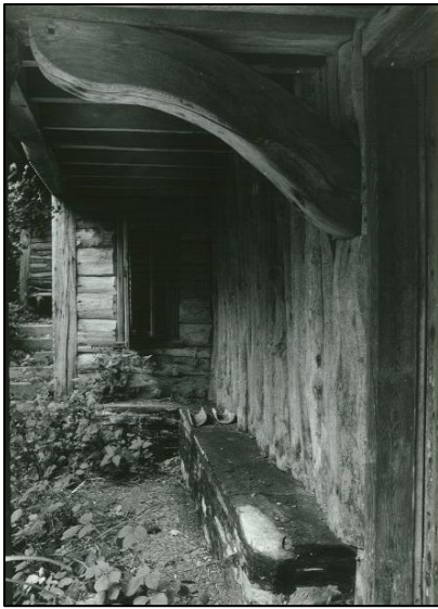
The fixed external bench during restoration
