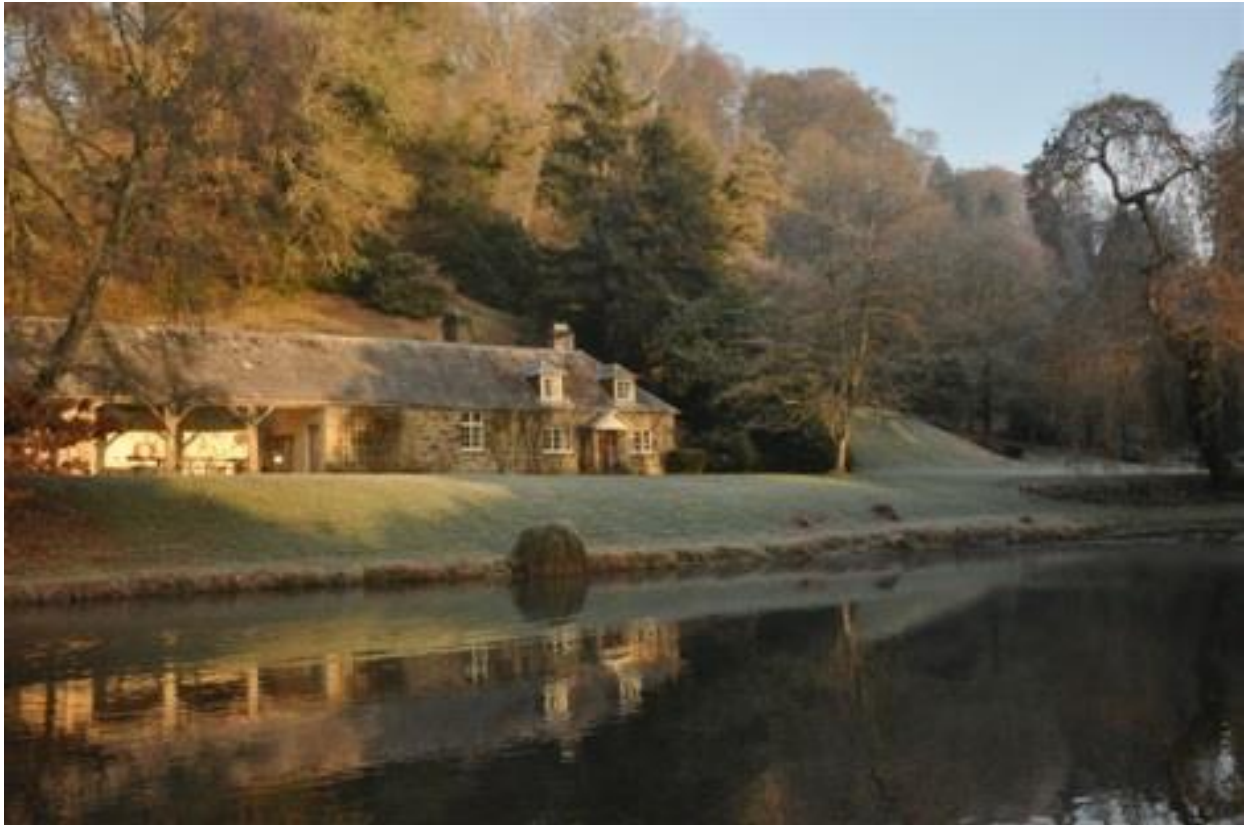
Pond Cottage beside Dairy Dell Pond in 1983 when the pond had largely dried up, and as it looks today. The Dairy stands just out of sight in the trees, atop the hillock to the right of the cottage.
