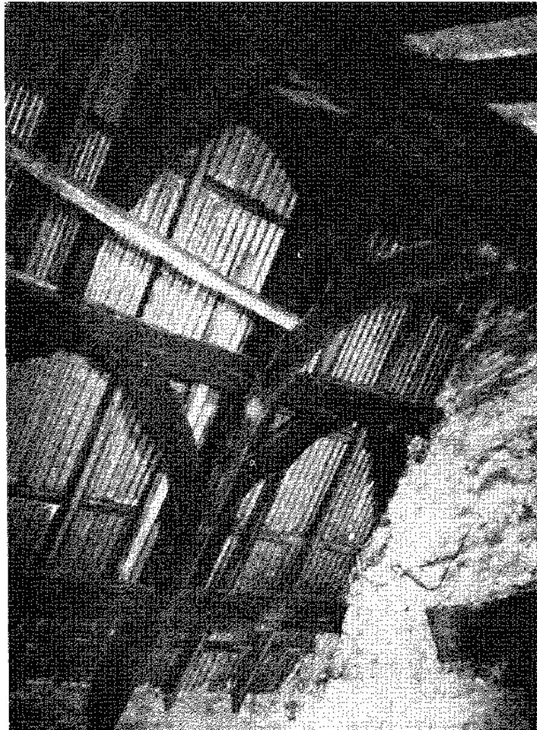
Fig. 6.—Plas Ucha. Secondary Roof Truss.
