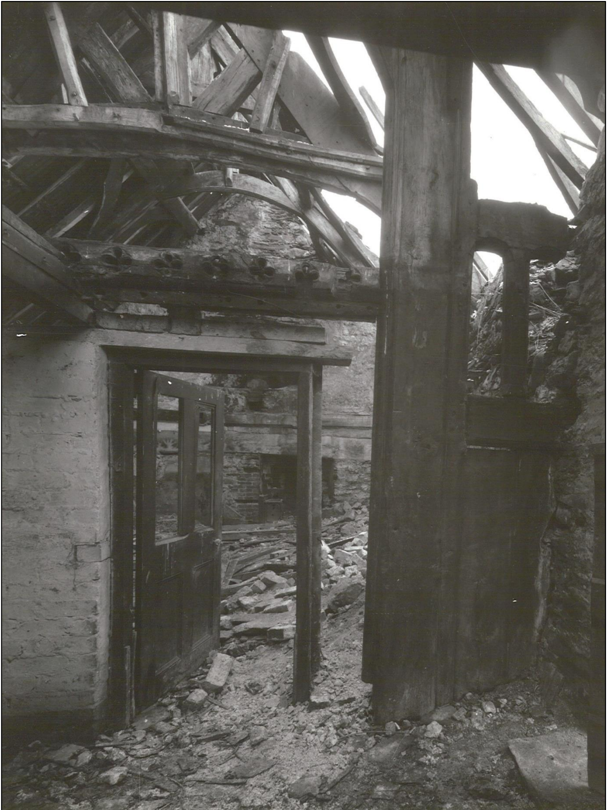
Interior in 1970, showing the spere truss and the beam linking the two aisle posts (RCAHMW).
