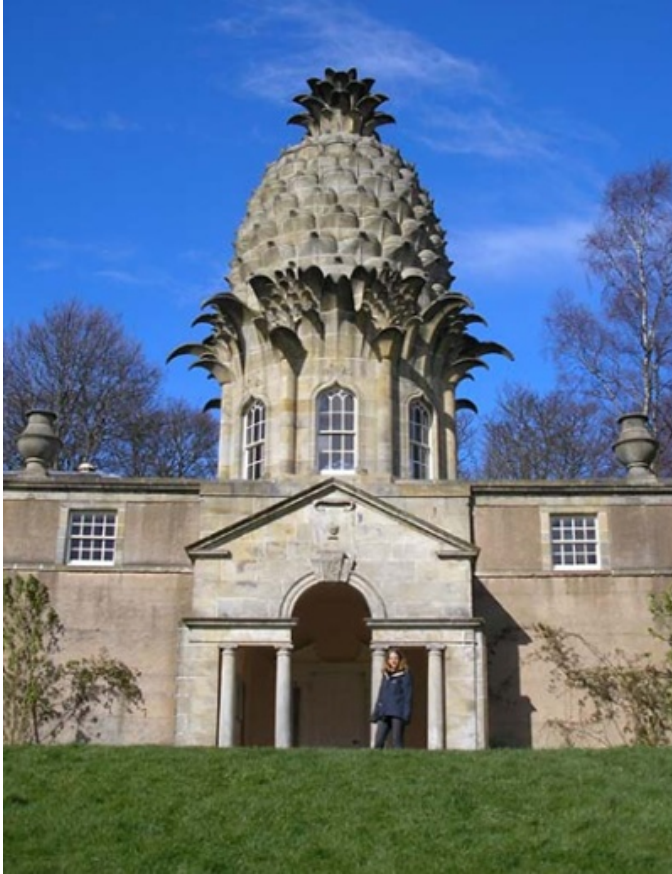
The extraordinary Pineapple Summerhouse at Dunmore, Scotland was once flanked by hothouses (1761–1776)
