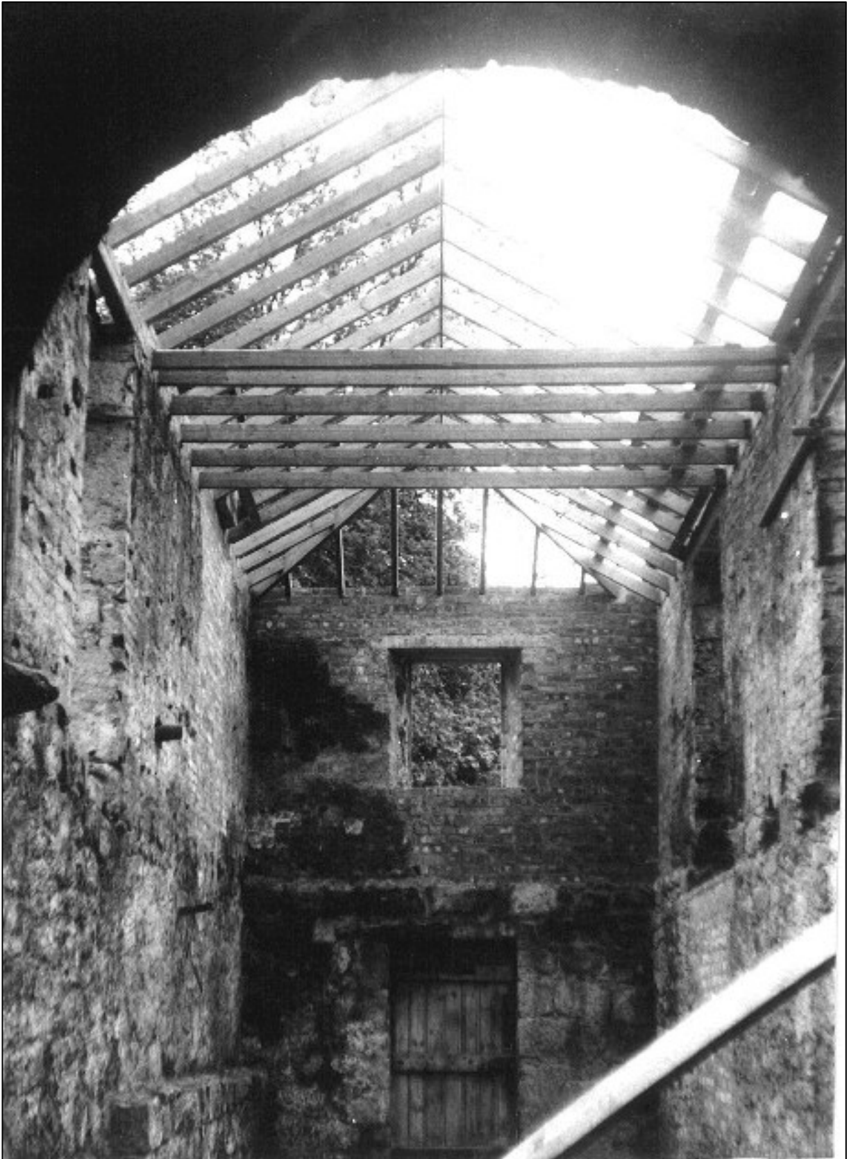
Re-roofing the East Wing.
