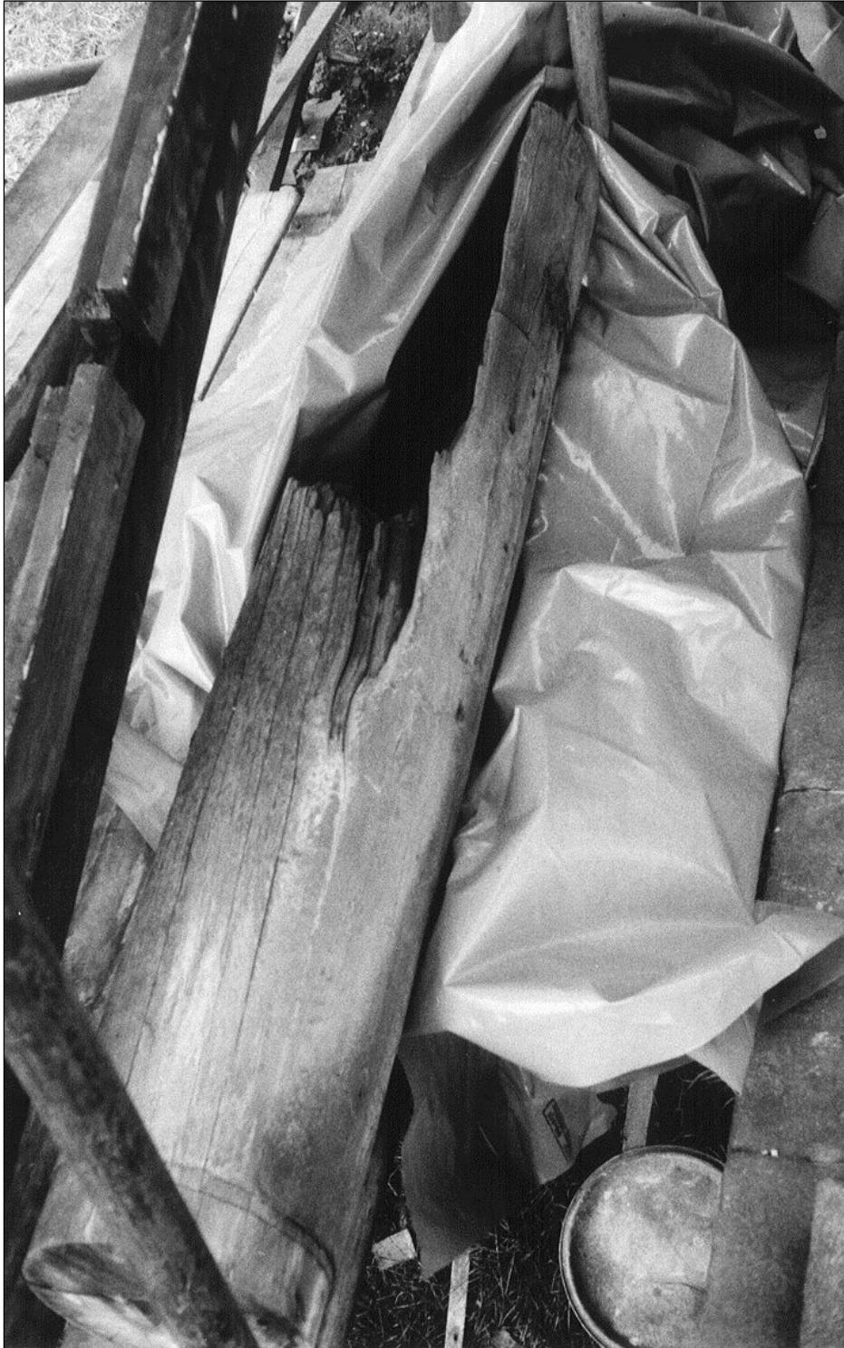
This column was too rotten to save, but helped to prevent the polythene from blowing away.
