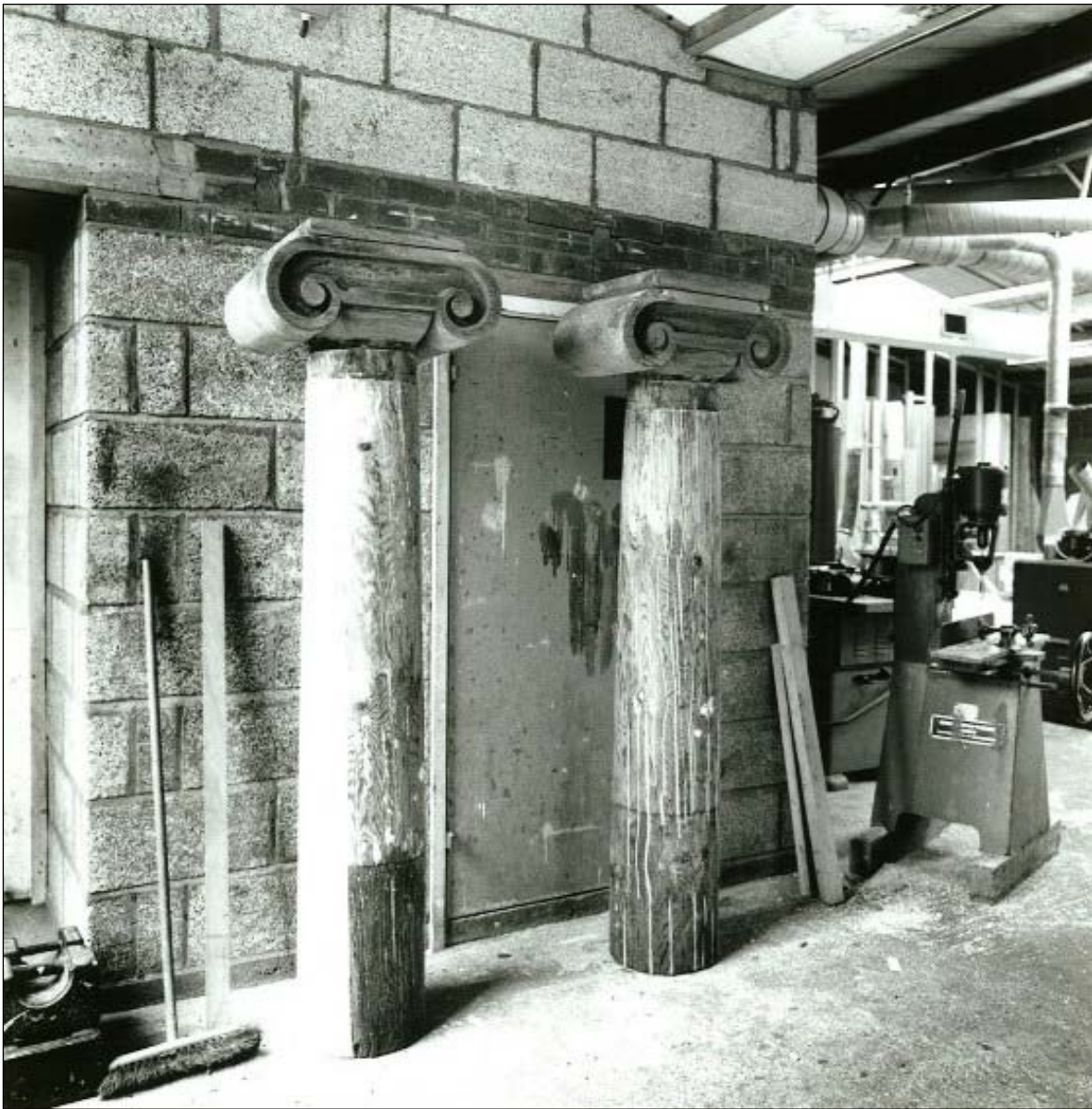
The two columns that could be saved. The paler strips are where new wood has been filleted in.
