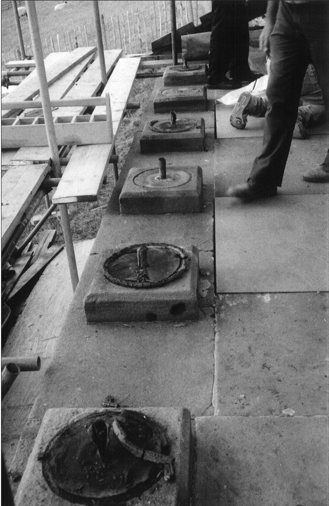
The bases of the columns after the portico was dismantled, and taken away for repair.
