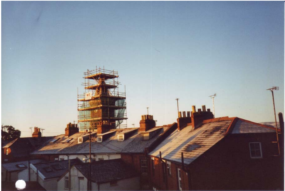
Restoration work in 1999
