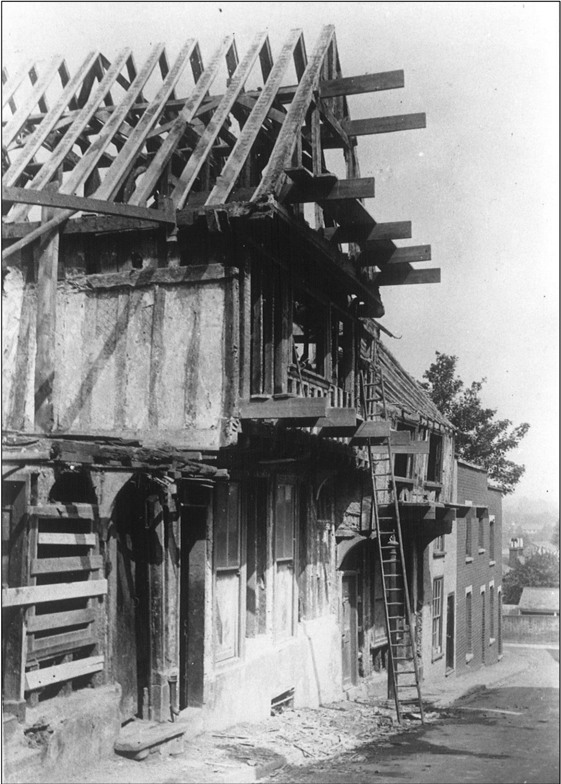
Peake's House in 1935 before restoration.
