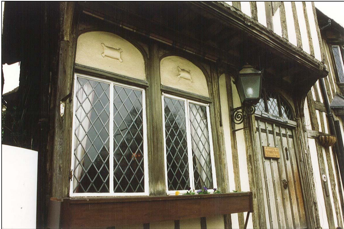
The lamp sits on a later stud inserted into the coffin doorway.
