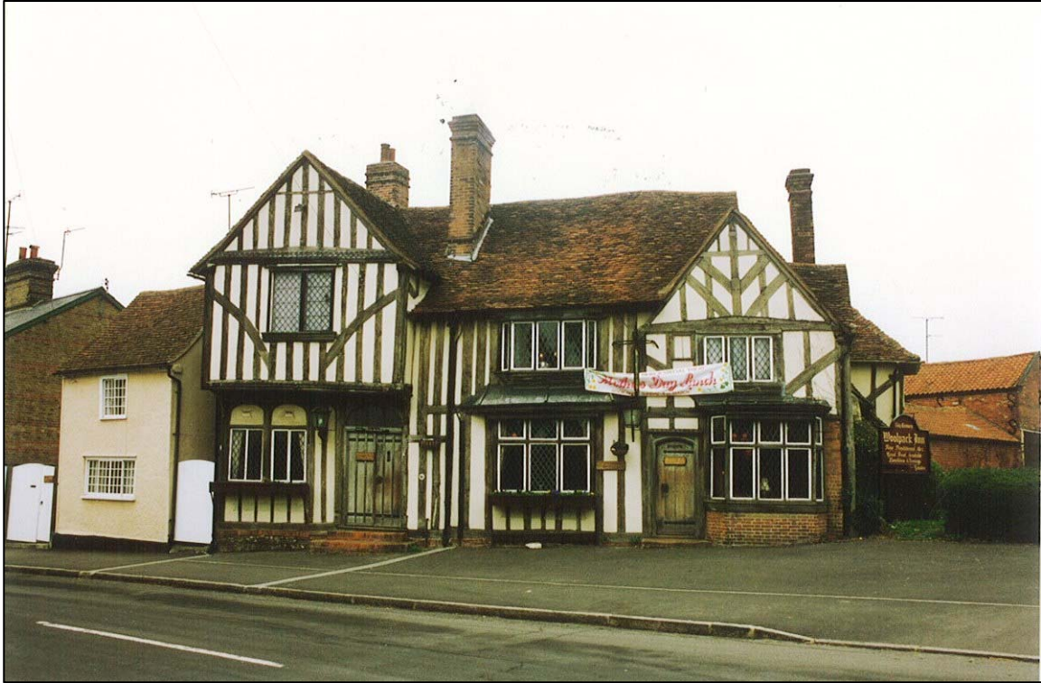
The Woolpack Inn, Coggeshall – the ground floor on the left hand side shows two shop windows and then the narrow coffin door.
