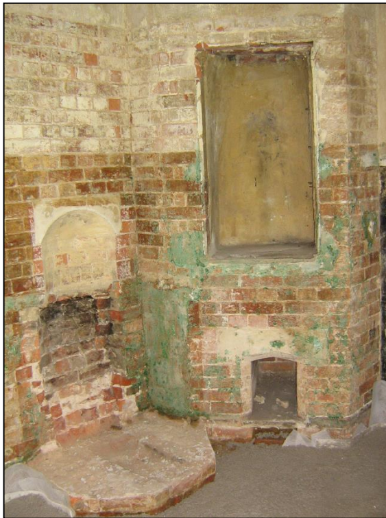
Decoding the original kitchen. Top: once this concrete floor screed was removed, the footprint of the base of the copper was revealed. Note the lowered ceiling. The walls have been ill advisedly painted with gloss paint in the past. Bottom left: the flagstones have been temporarily lifted to allow underfloor heating to be laid in a limecrete base. The ash hole for the bread oven is re-opened. Bottom right: the reconstructed copper plinth, complete with firehole.
