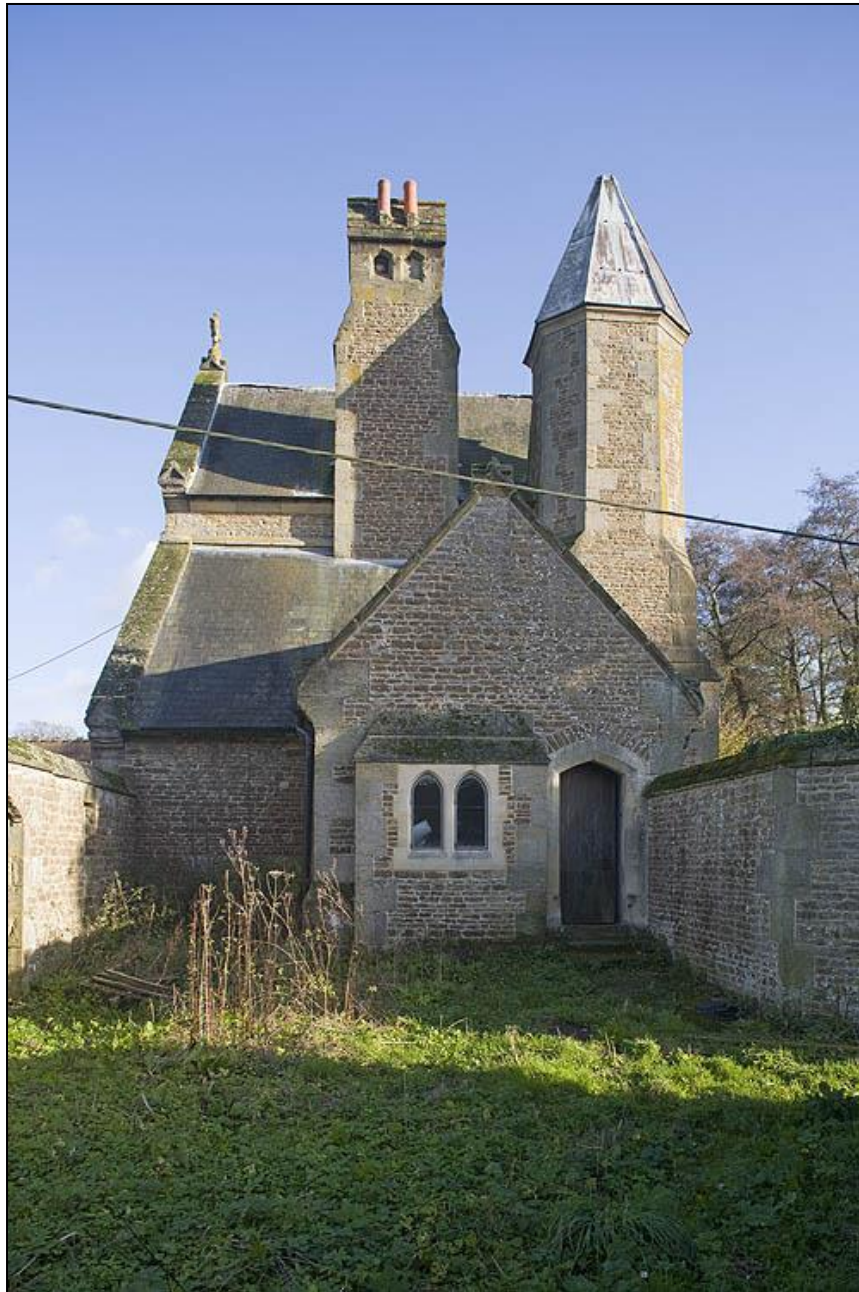
West elevation before work began.
