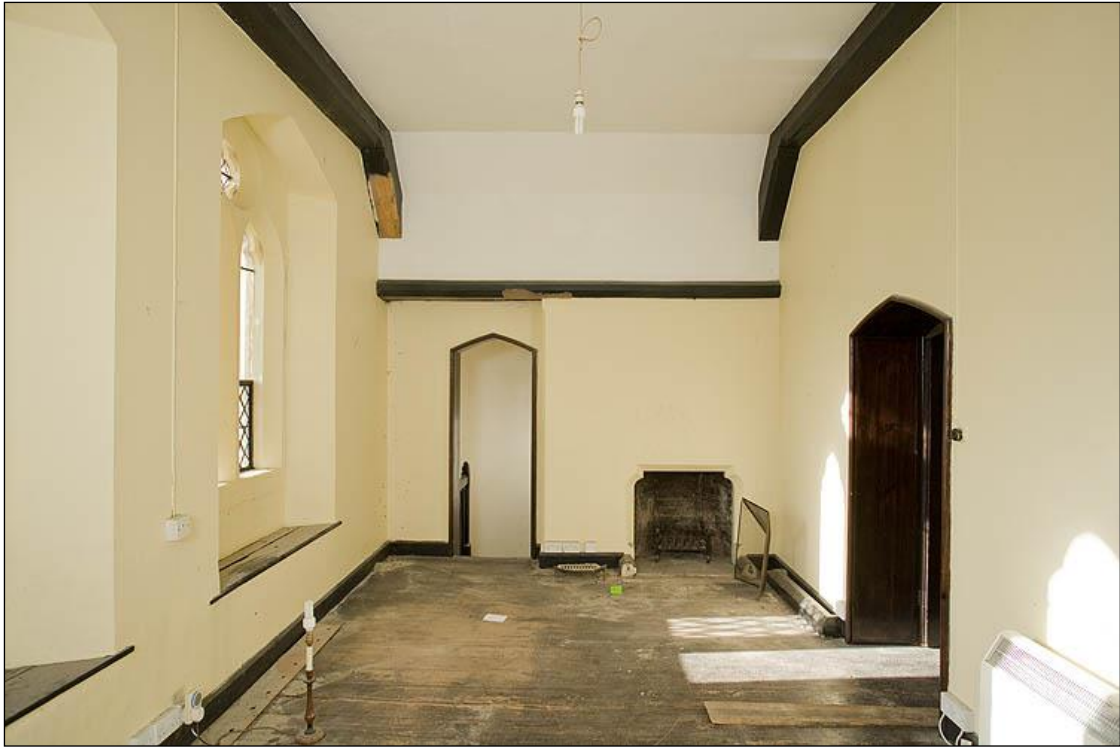
The living room before work began.
