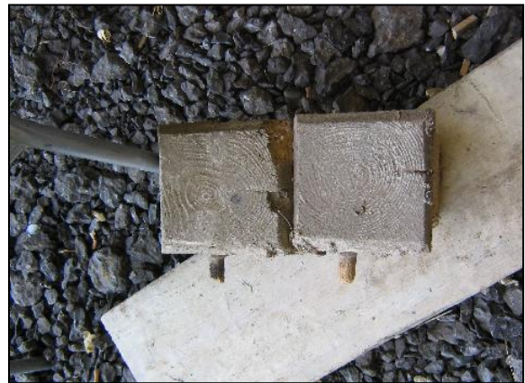
The oak 'cobbles' are surprisingly sophisticated in construction, being diagonally bedded, nailed and pegged.
