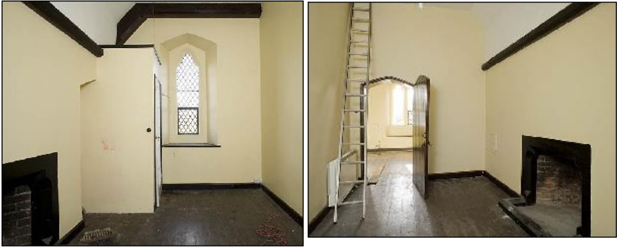
The kitchen before work began. The photo on the left shows the top of the modern staircase as it emerged into the room. The partition between the two rooms on the north side of the first floor appears to be original.
