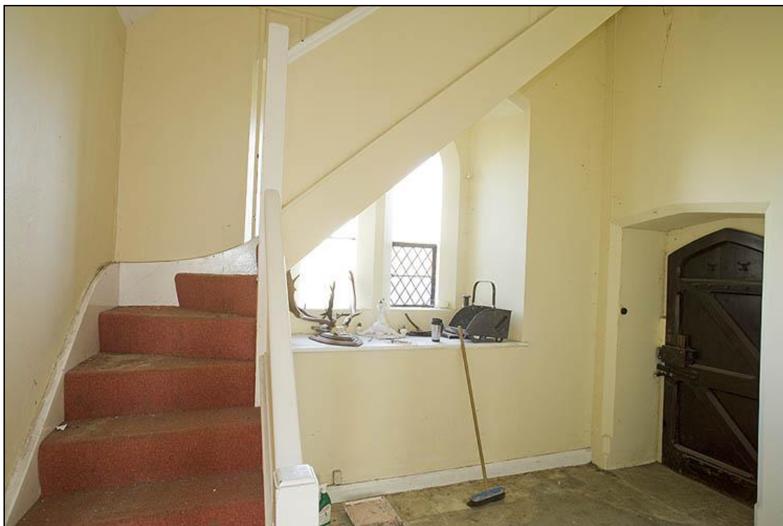
The inserted modern staircase in today's ground floor bedroom, now removed.
