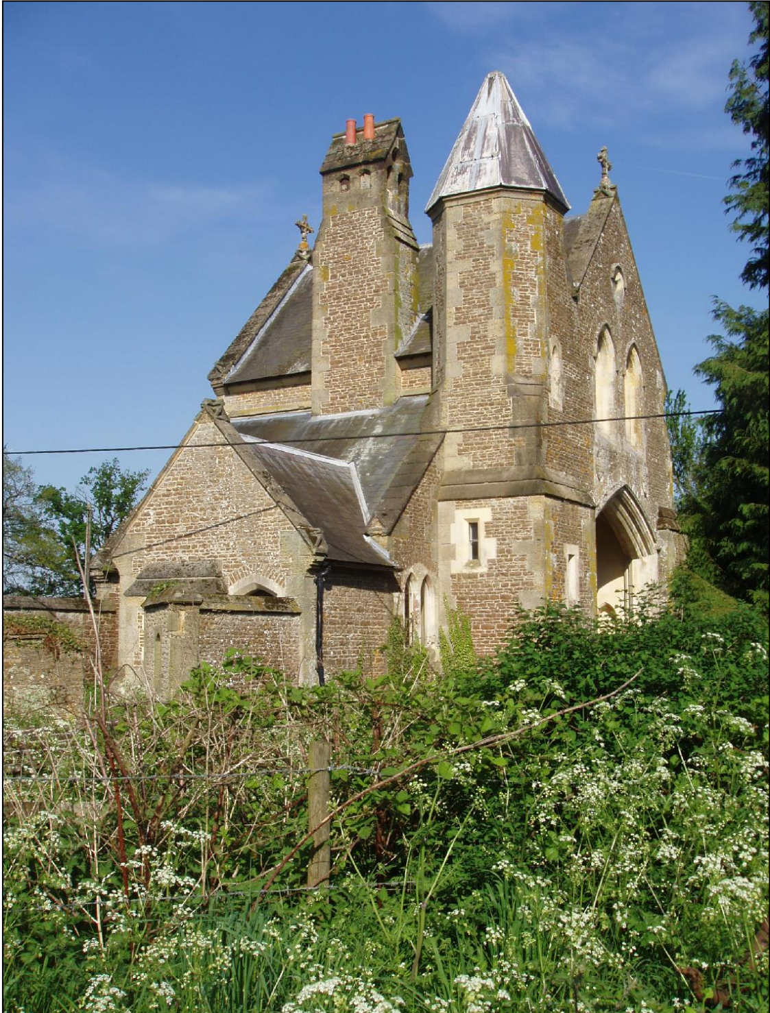
Oxenford Gatehouse in May 2008, before refurbishment began.
